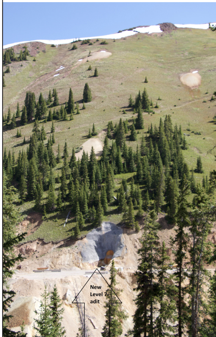
View of the Gold King Mine adit from across the North Fork Cement Creek gulch, showing stabilization efforts with Shock-Crete application. June 14, 2016.
