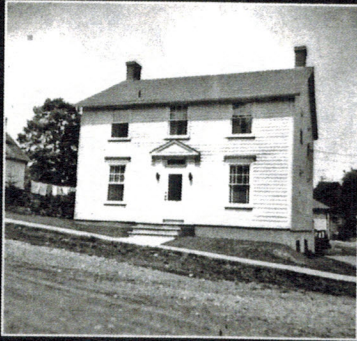
3. The verandah has been removed, the lower sashes have a single pane and a pediment has been placed over the doorway. c1940. Collection J. McKendry.
