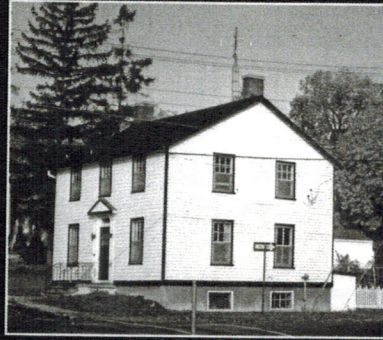
4. Stucco now covers the stone foundation, and the pronounced mouldings over the windows covered over when new siding was applied. 1993. Photo J. McKendry.
