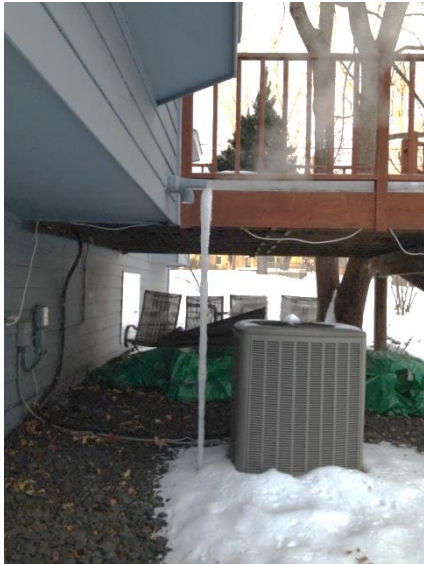
Residential Condensing Furnace Flue in MN
