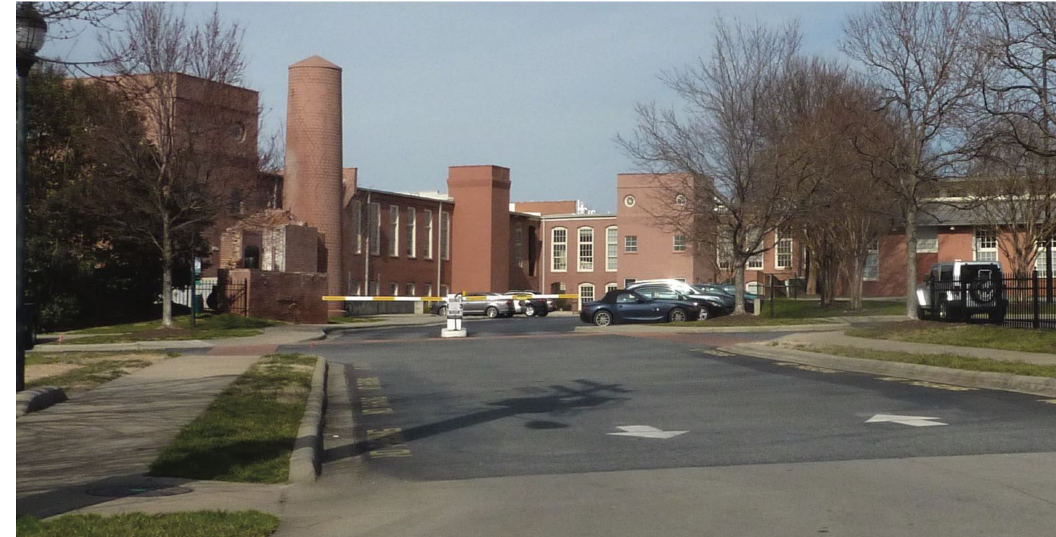
VIEW 05 looking N at site entry from N. Brevard St
