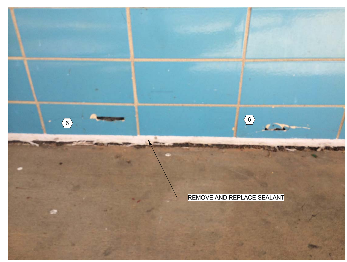
8 COLUMN R39 R40 PHOTO 1
