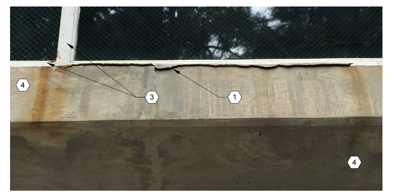
15 COLUMN R15 R16 PHOTO 1
