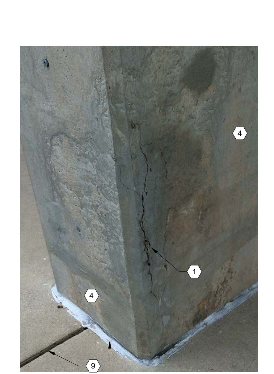
14 COLUMN R15 PHOTO 3
