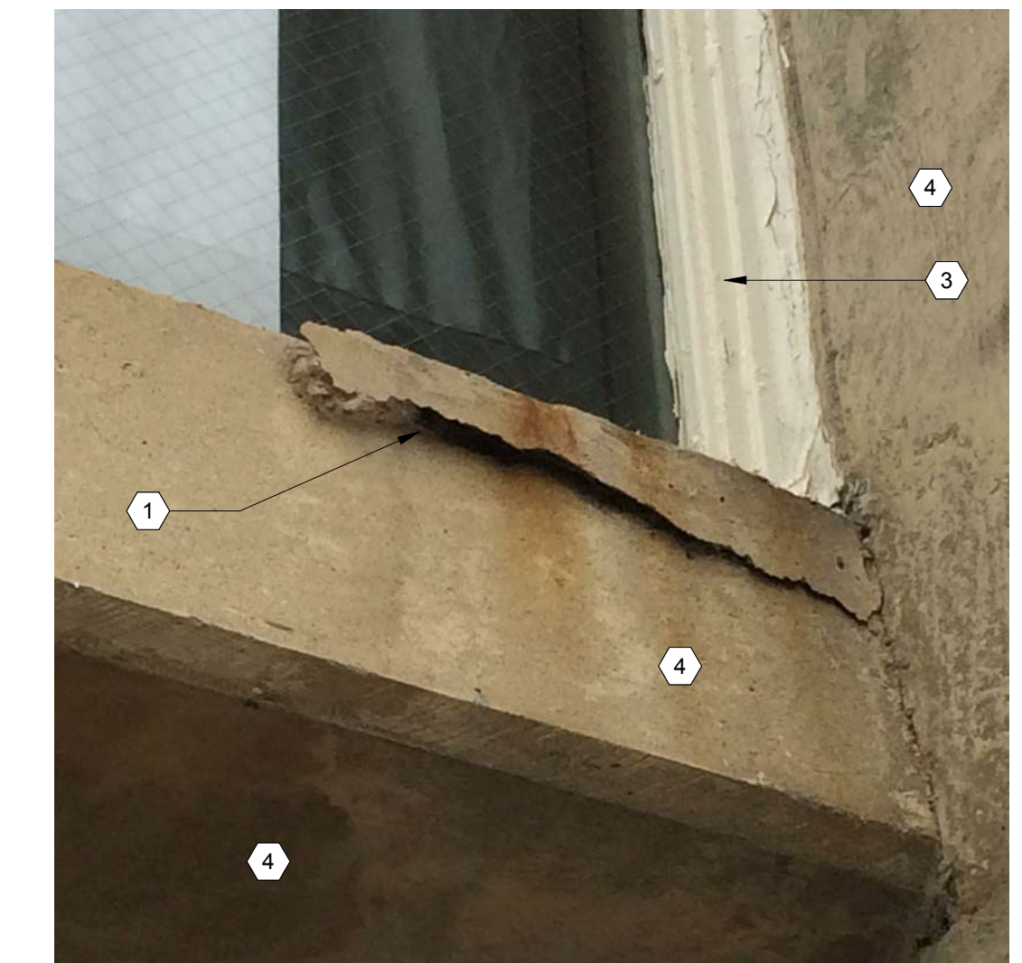
3 COLUMN R41 PHOTO 1
