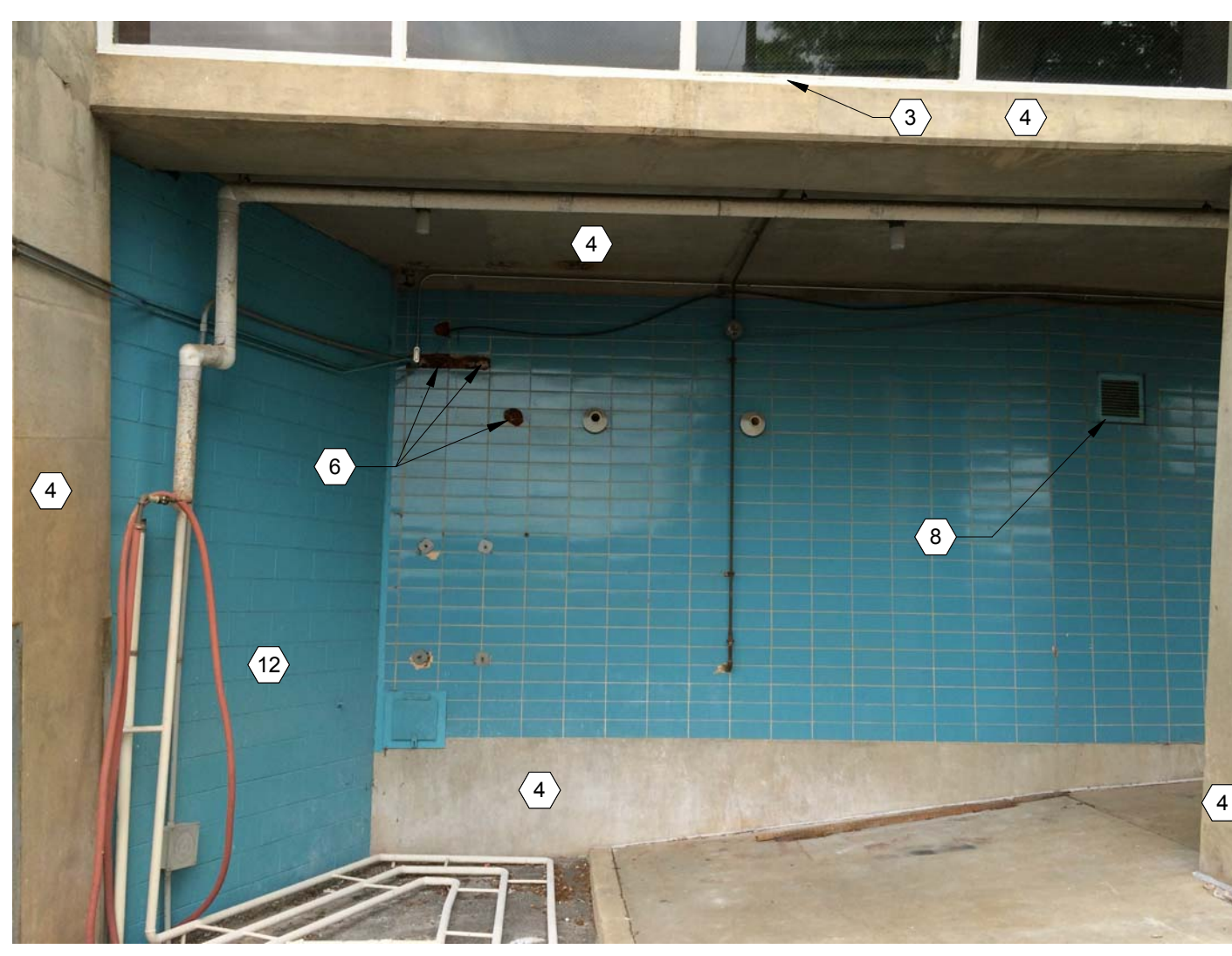
1 COLUMN R37-38 PHOTO 1
