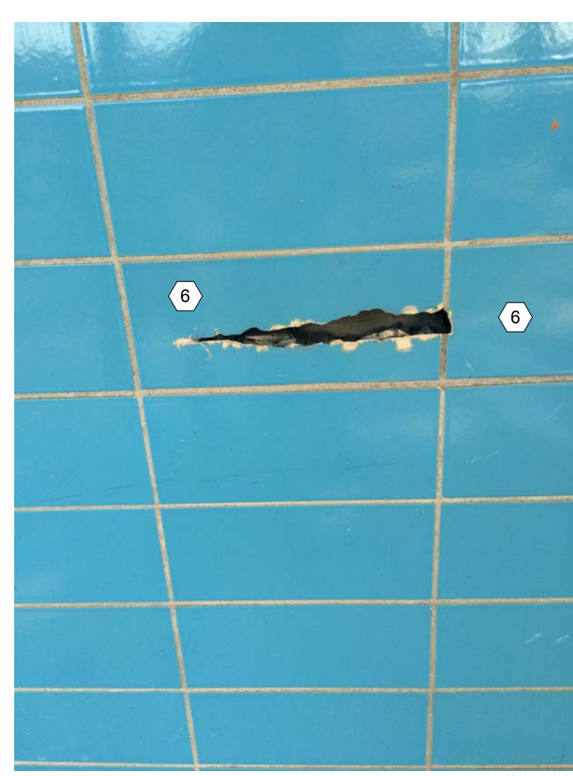
6 COLUMN R38 R39 PHOTO 1
