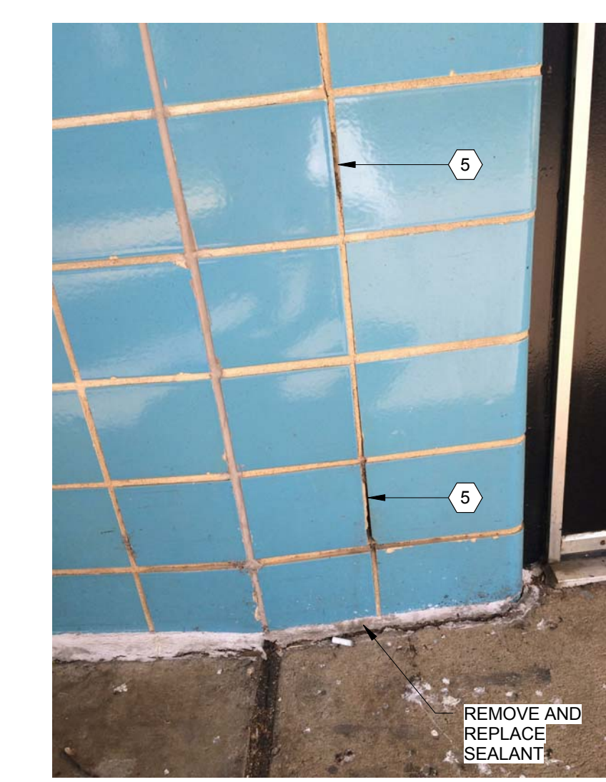
9 COLUMN R40 PHOTO 2
