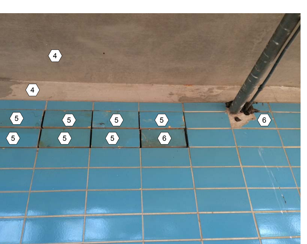
16 COLUMN R31 R32 PHOTO 1
