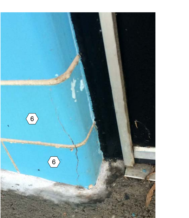
14 COLUMN R31 PHOTO 2
