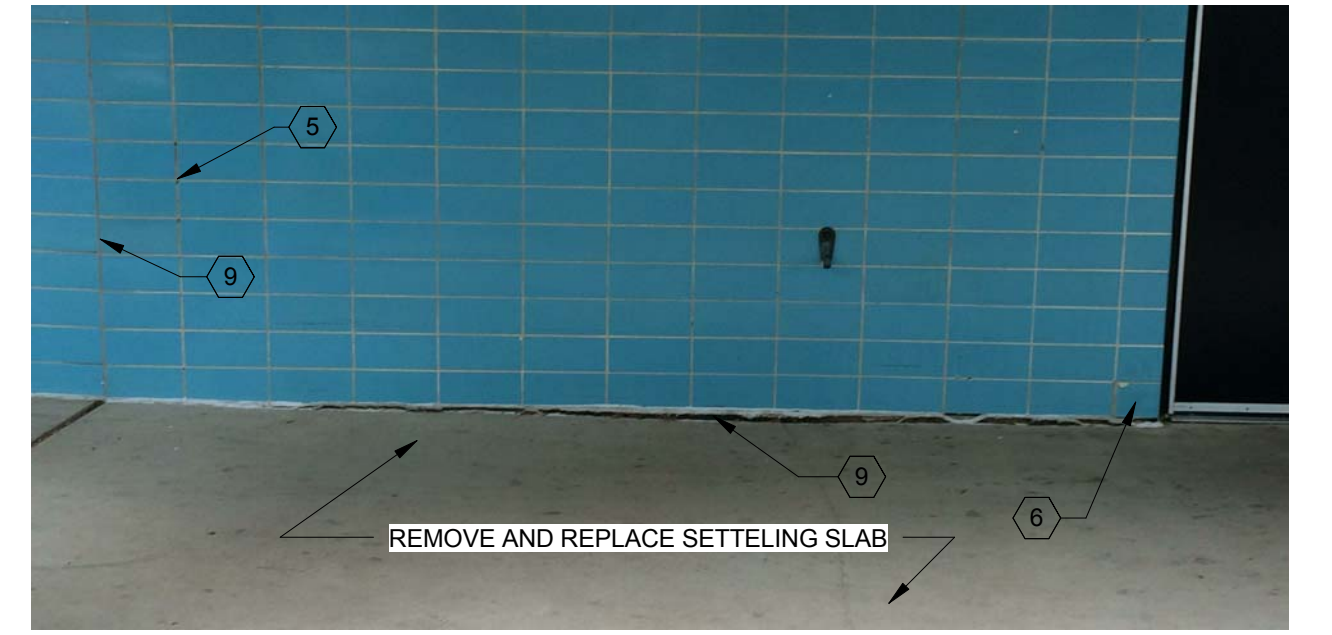
16 COLUMN R15 R16 PHOTO 2
