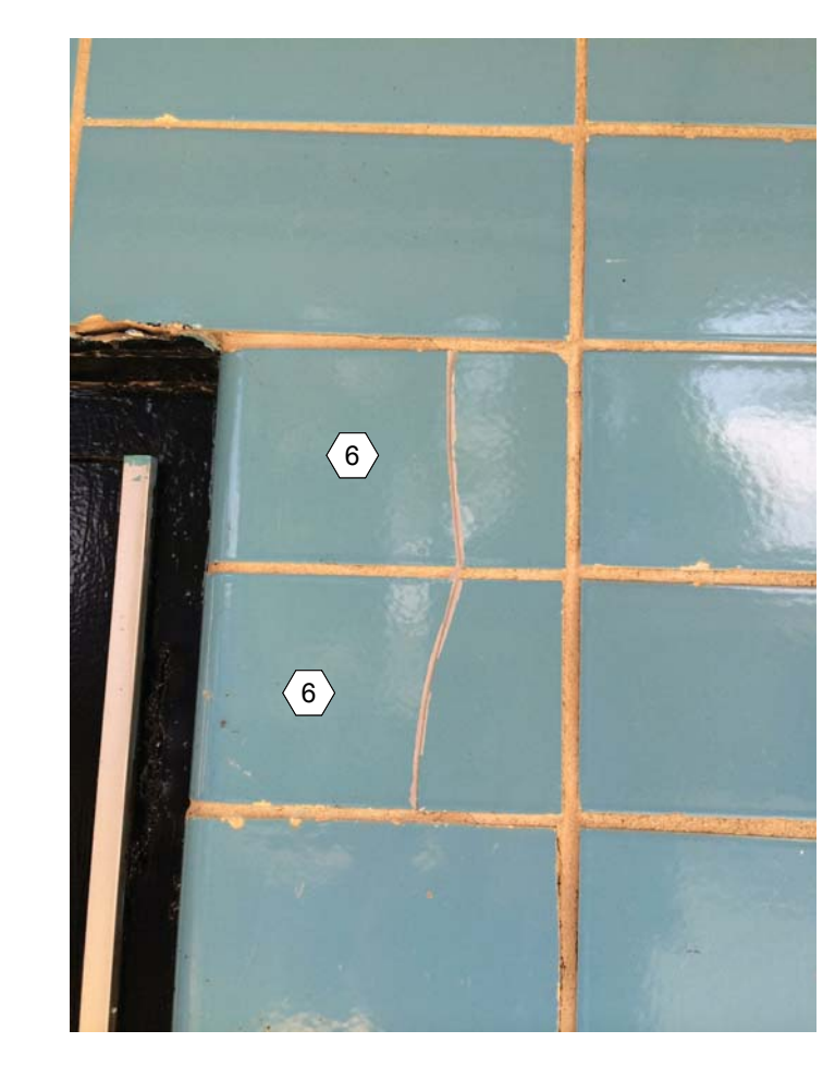
10 COLUMN R40 PHOTO 1
