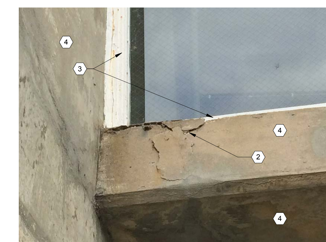
11 COLUMN R35 PHOTO 2
