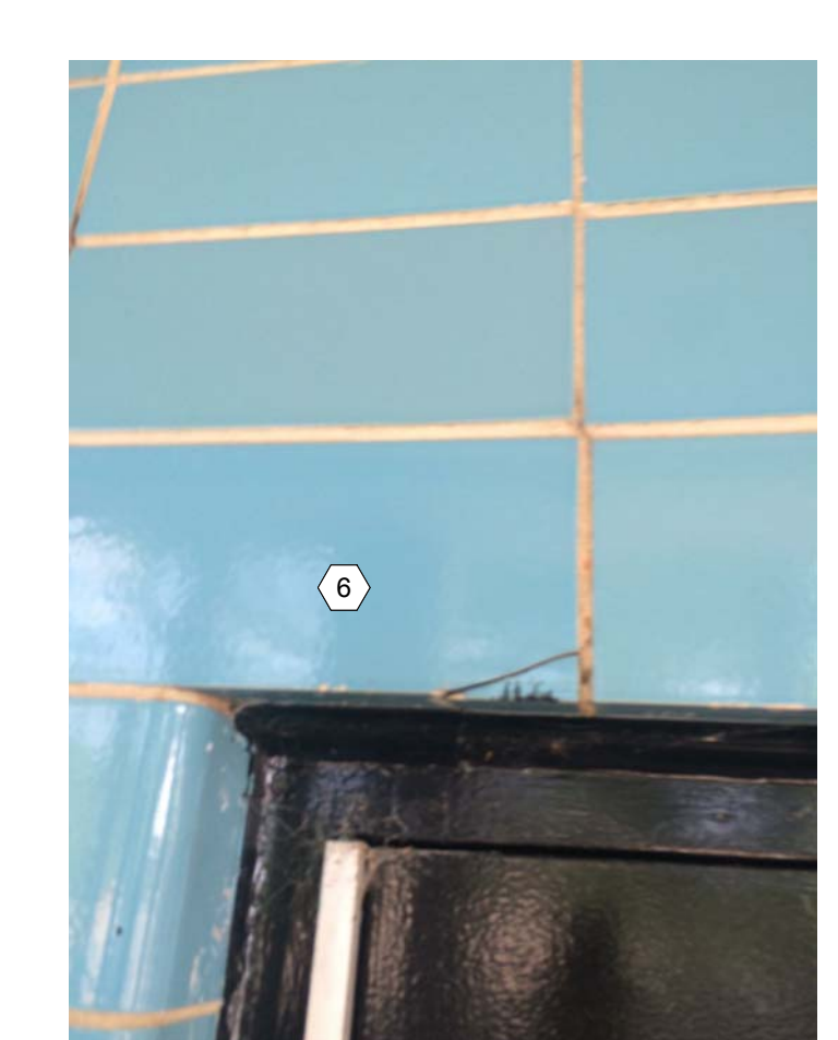
18 COLUMN R32 PHOTO 2
