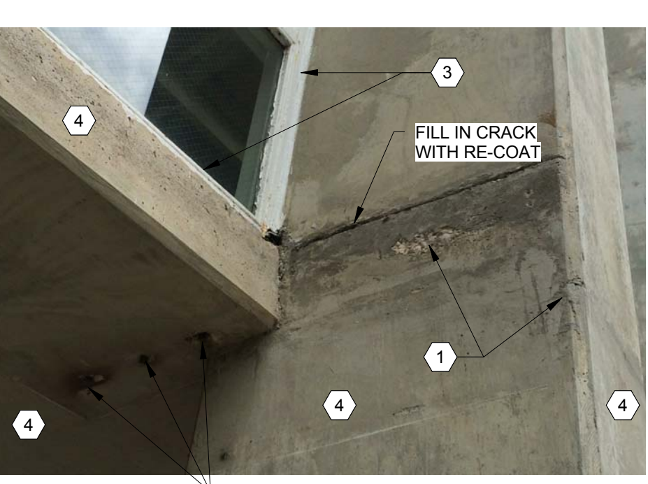
1 COLUMN R13 PHOTO 1
