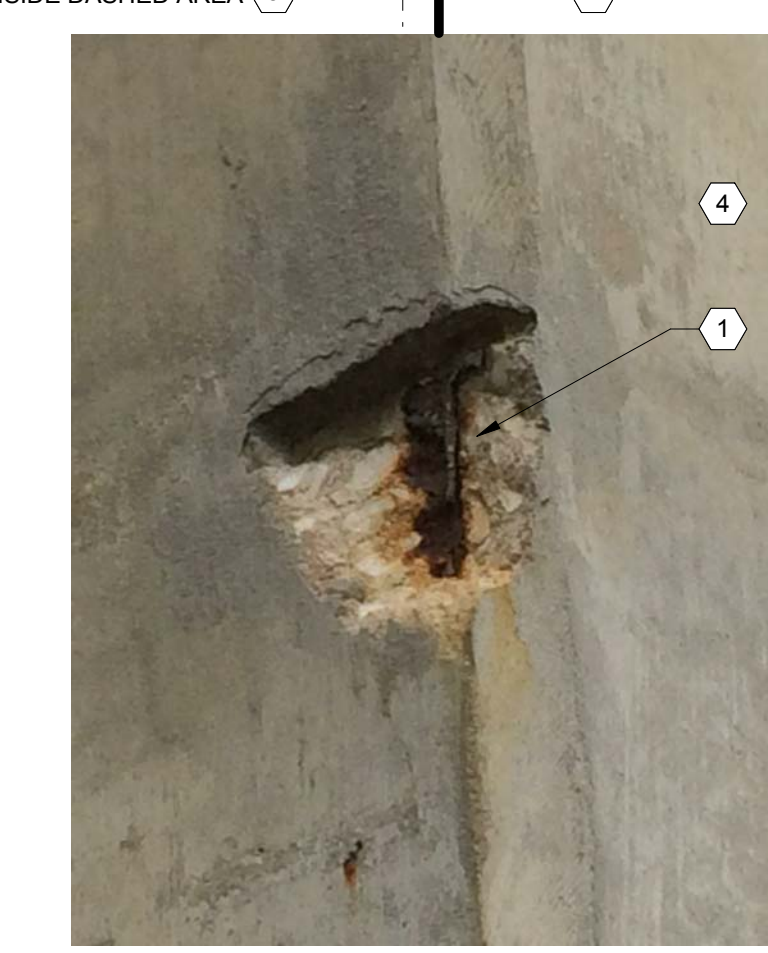
3 COLUMN R23 PHOTO 1
