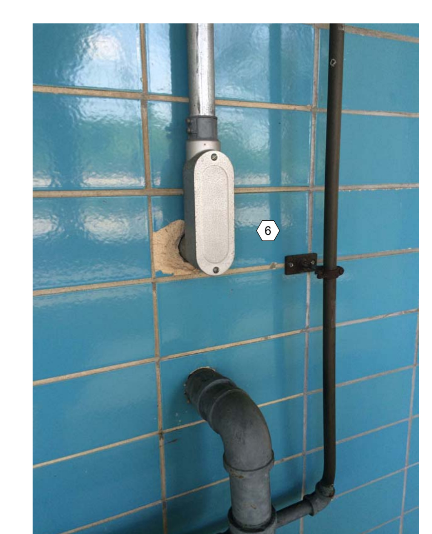
13 COLUMN R29 R30 PHOTO 3
