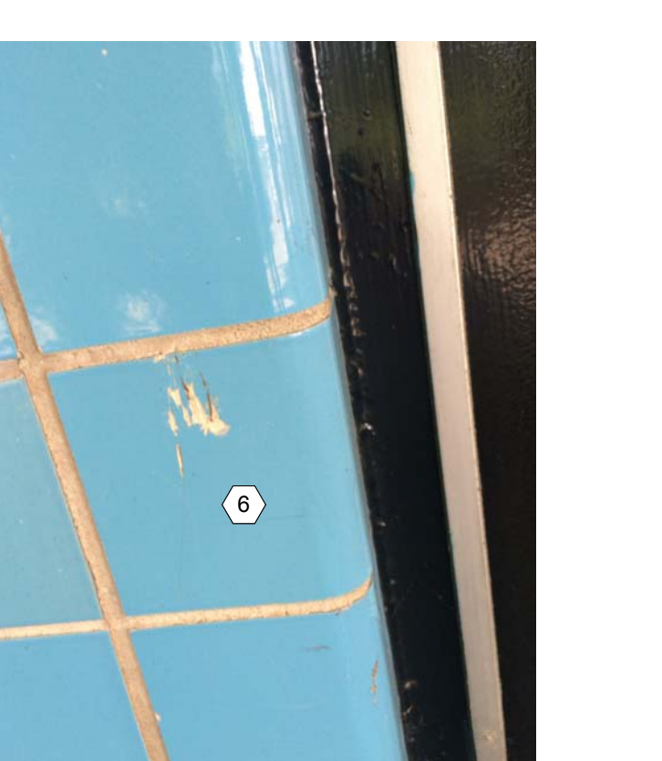
17 COLUMN R32 PHOTO 1
