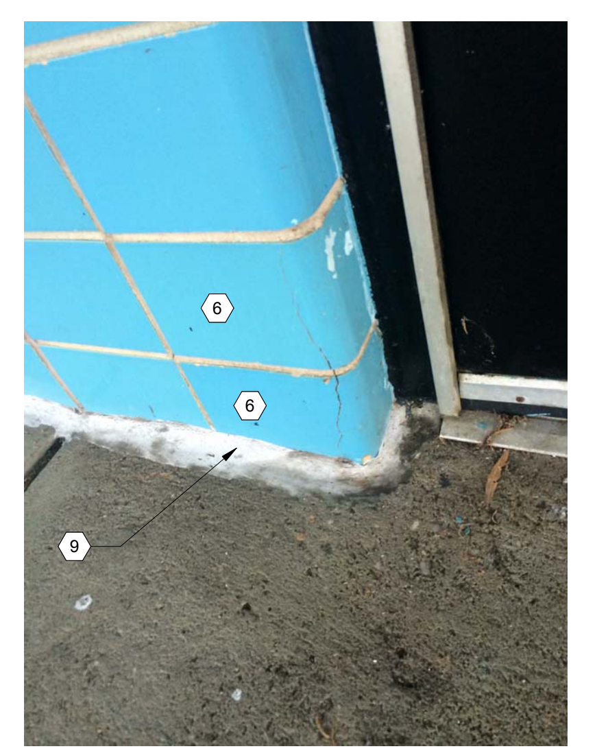
18 COLUMN R18 PHOTO 1
