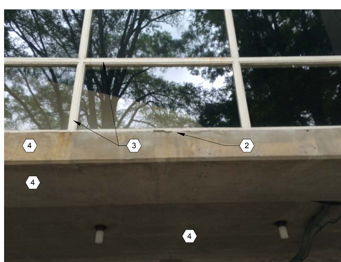
8 COLUMN R31-32 PHOTO 1
