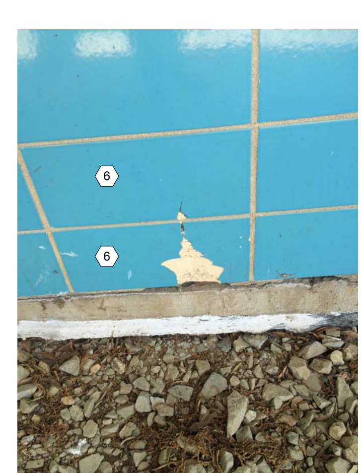
19 COLUMN R34 R35 PHOTO 1
