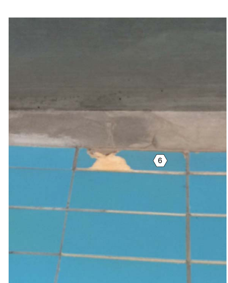
15 COLUMN R30 R31 PHOTO 1
