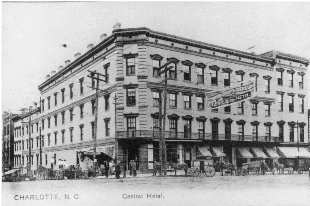
Central Hotel, courtesy of PLCMC
