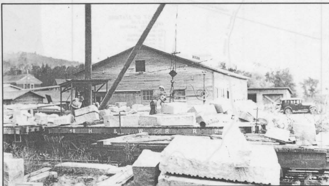
The travelling crane operator of the Woodbury Granite Co. above, must have been one busy fellow loading cars and feeding the surfacing, crusher and polishing machines. Coll. Stearns Jenkins. 8-170.
