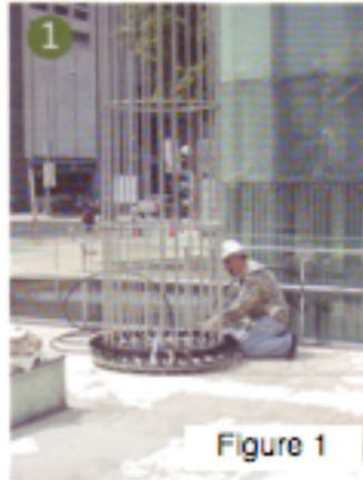
Figure 1: Fix the round iron tube on ground with the iron rods formed to desire shapes (example: round type).
