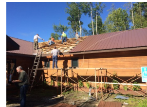
A VIM team from Tennessee work on the church roof.
