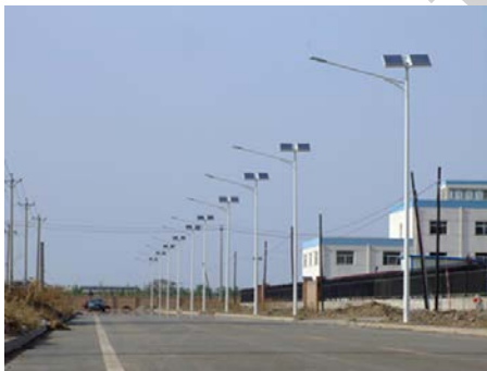
Type of PV Street Light : Battery Burying Site location: Naypyidaw, Myanmar.
