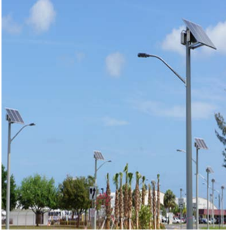
Type of PV Street Light : Battery Hanging Site location: Penang, Malaysia. Project completion date: 07, Nov. 2008
