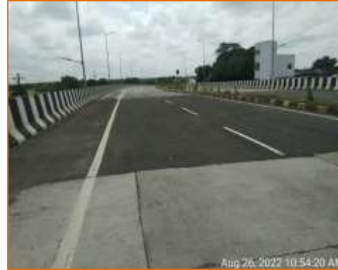
LVUP at km. 121.950 (RHS)
