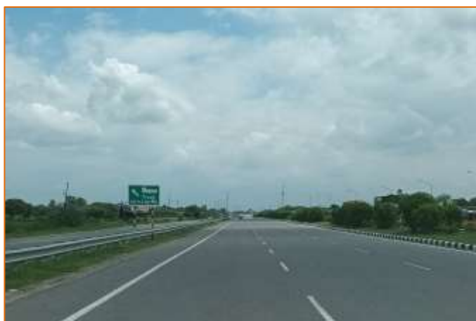
Truck Lay Bye at km. 727+900
