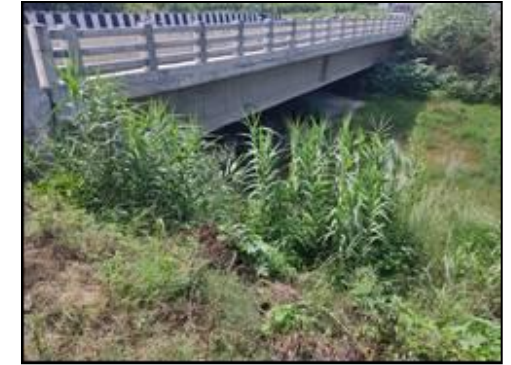
Minor Bridge at km. 66+020 (New Structure View)
