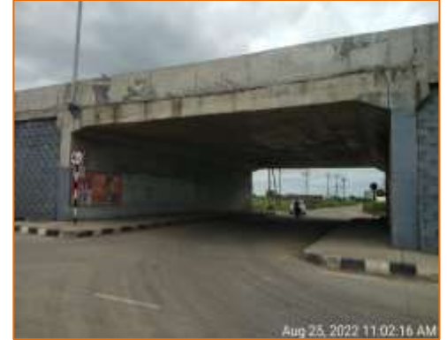
Side View of LVUP at km. 132.025 (RHS)
