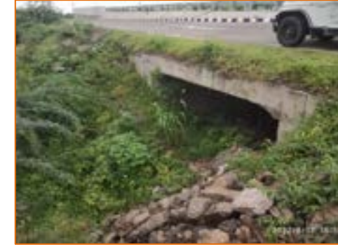
Box Culvert at km. 311.734
