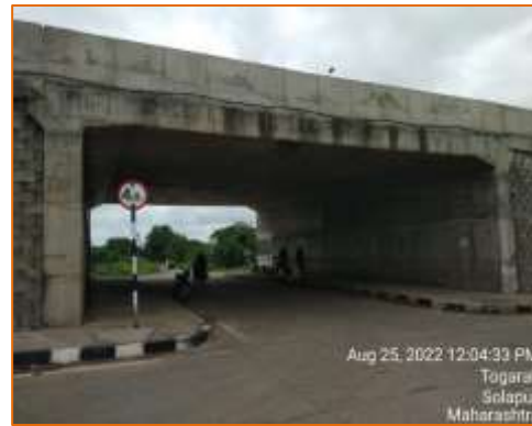
Side View of LVUP at km. 125.055 (LHS)
