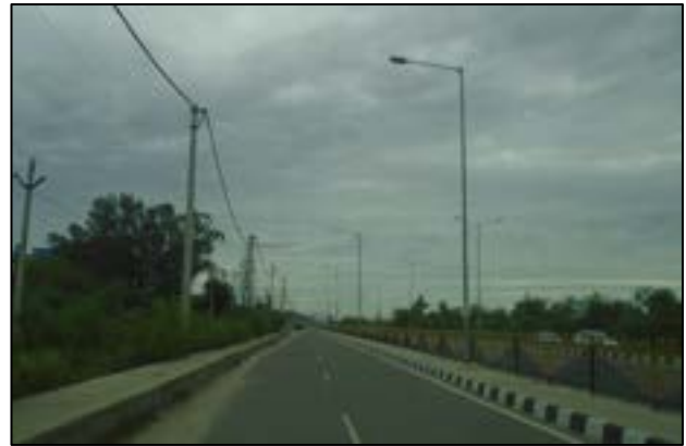
Street Lighting at Service Road
