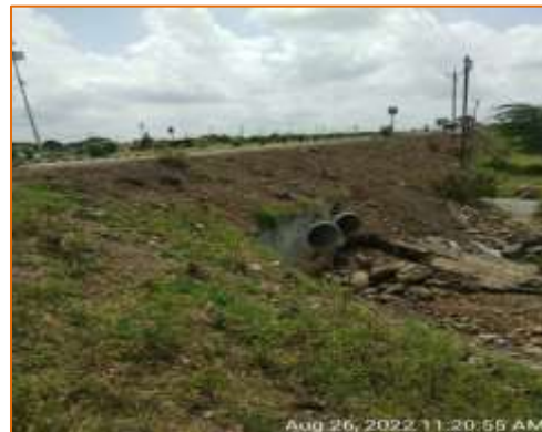
Pipe Culvert at km. 117.423 - LHS (Widening)
