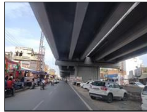
Elevated Structure at km. 25+319
