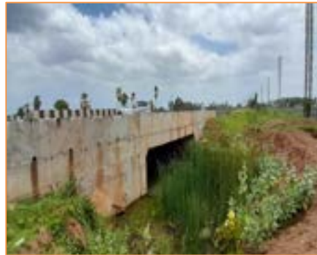
View of Minor Bridge at km. 26+850
