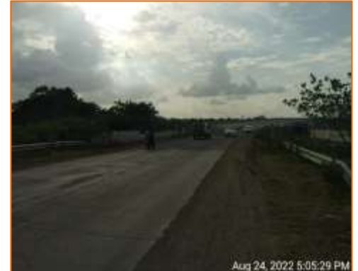
View of MNB at km. 99.586 (LHS)
