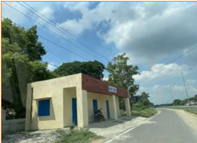
Rest Area at km. 727+800
