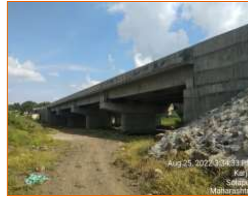
Side View of Major Bridge at km. 114.405 (RHS)
