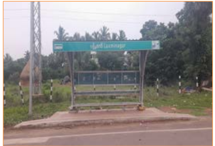
Bus Bay with Shelter at km. 56+140
