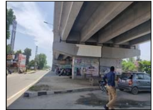
Flyover at km. 59+818
