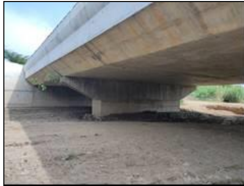
Minor Bridge at km. 68+519 (Substructure and Superstructure)
