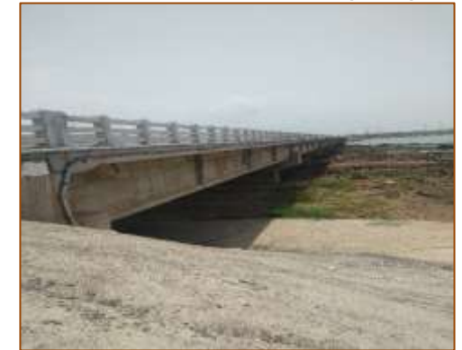
Side View of MJB - New at km. 433+276 (LHS)
