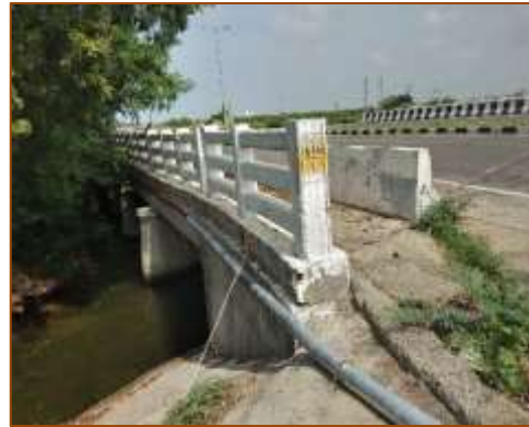
Side View of Minor Bridge at km. 483+502 (LHS) - Widening
