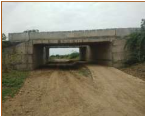
LVUP at km. 422+750 (RHS) - Under COS
