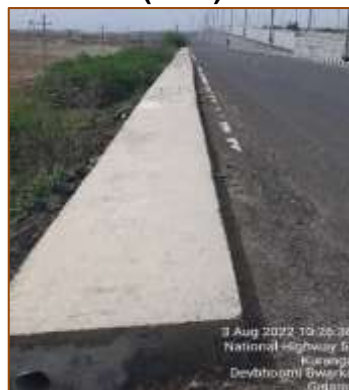
Built-up drain from km. 467+601 to km. 468+347 (RHS)
