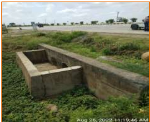
Pipe Culvert at km. 117.423 - RHS (Widening)
