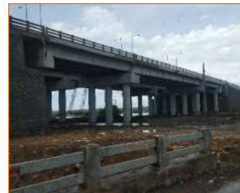
Side View of ROB at km. 0+527 (RHS)
