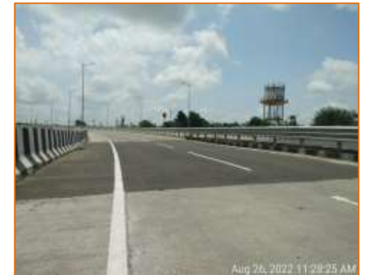
LVUP at km. 114.080 (RHS)
