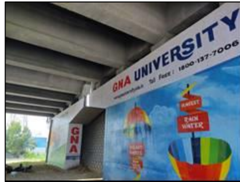
Flyover at km. 39+915
