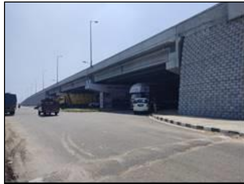
Flyover at km. 39+915
