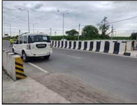
Minor Bridge at km. 77+613 (Top View)
