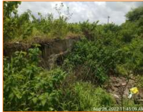
Pipe Culvert at km. 109.578 - LHS (Widening)
