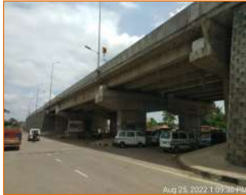
Side View of Flyover at km. 117.935 (LHS)
