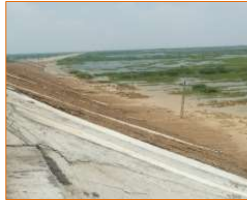
Side Slope @ A2 side of ROB at km. 0+527 (RHS)
