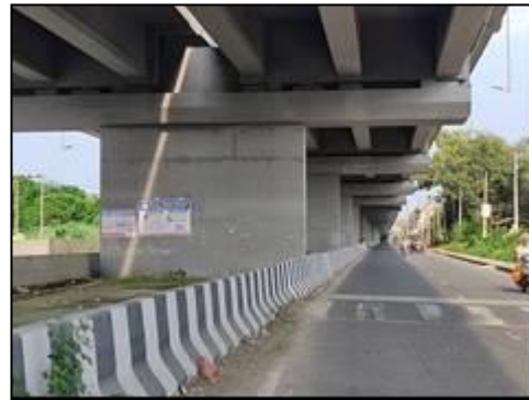
Elevated Structure at km. 25+319
