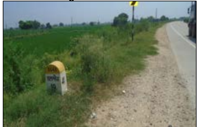
Kilometer Stone at km. 41+000
