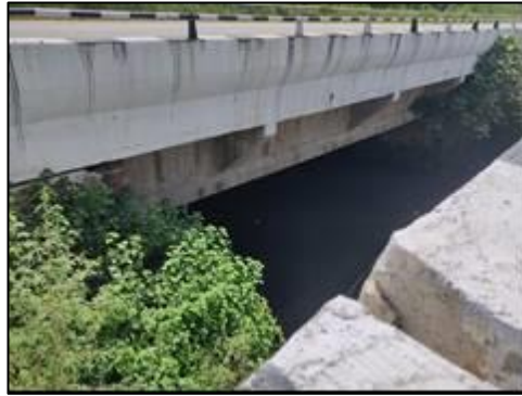
Minor Bridge at km. 62+704 (New Structure View)
