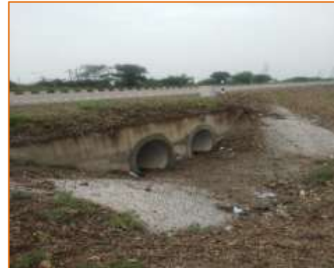
HPC at km. 70+640 (RHS)
