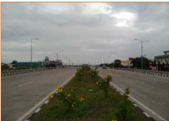
Pavement Condition at km. 285+750 (BHS)
