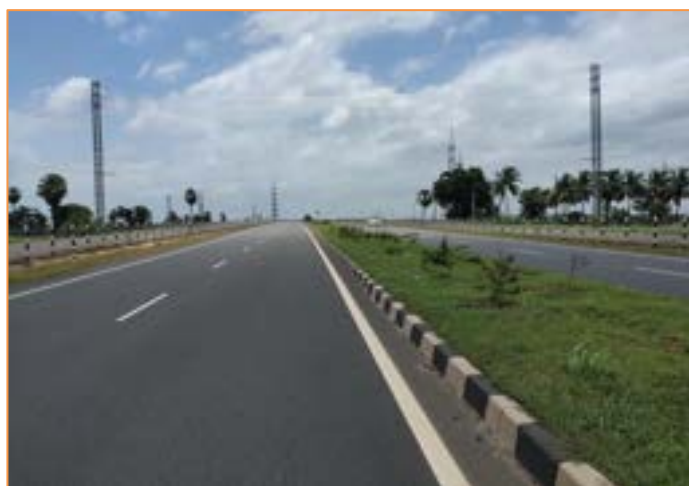
Pavement Condition at km. 76+900
