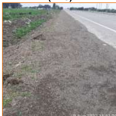
km. 44+000 to km. 43+000 (RHS)
