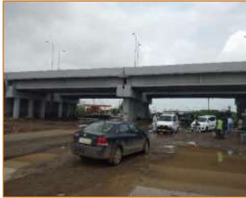
Side View of VUP at km. 12+420 (RHS)
