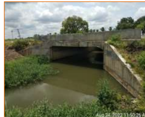
Side View of Minor Bridge at km. 104.348 (RHS)
