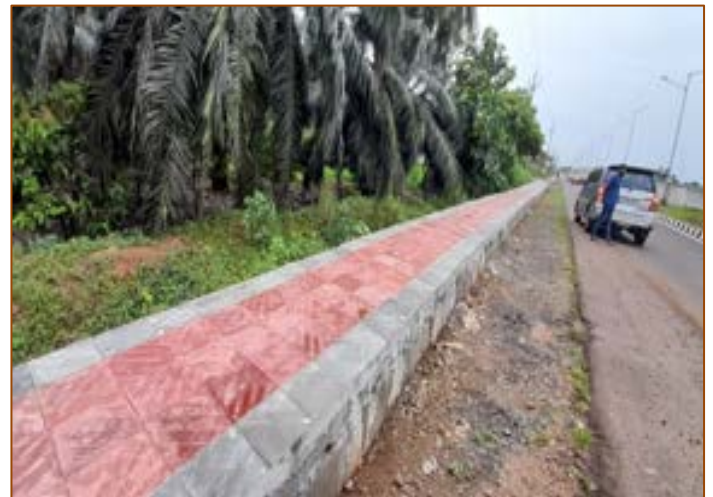
Built-up Drain cum footpath at km. 36+450
