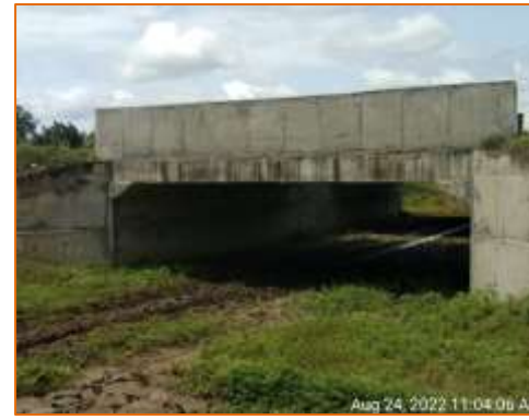
Side View of Minor Bridge at km. 101.260 (RHS)
