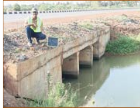
Box Culvert at km. 26+605
