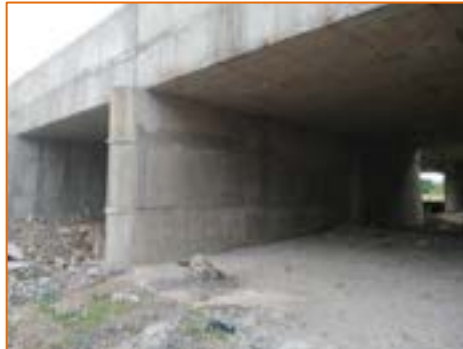
Widening of Existing Minor Bridge at km. 281.277
