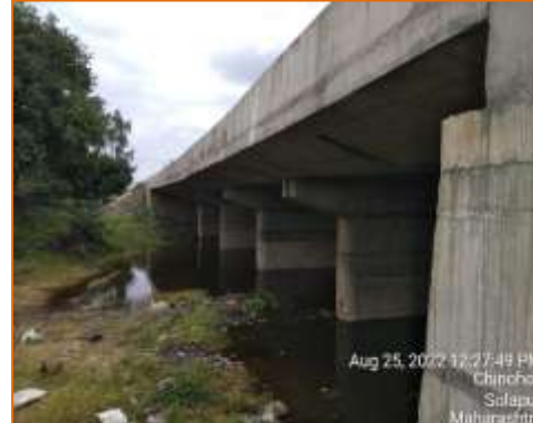
Side View of Minor Bridge at km. 124.337 (RHS)
