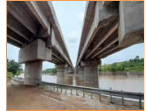
View of Major Bridge at km. 68+742
