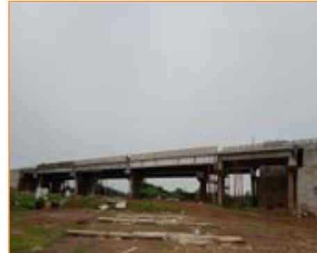
View of ROB at km. 18+677
