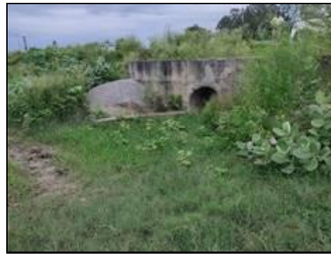
HP Culvert at km. 1+850
