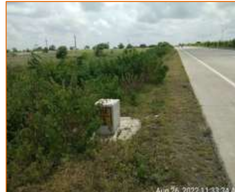
Pipe Culvert at km. 113.155 - RHS (Widening)
