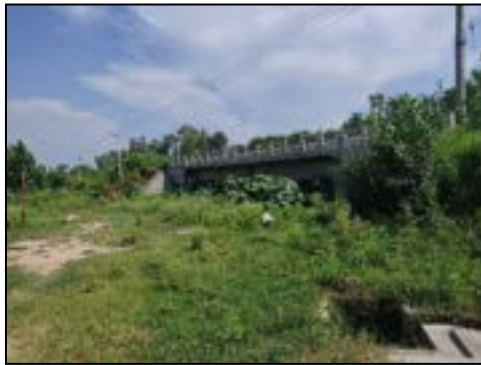
Minor Bridge at km. 62+704 (Existing Structure View)
