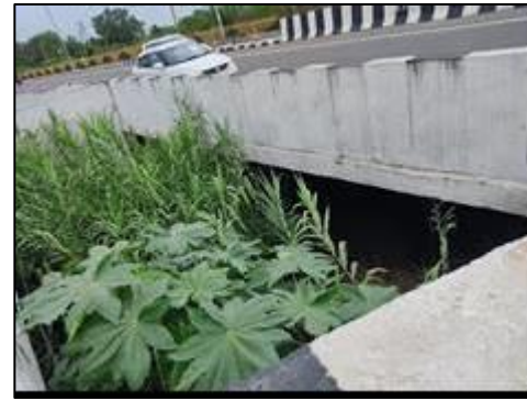
Minor Bridge at km. 78+636 (Structure View)
