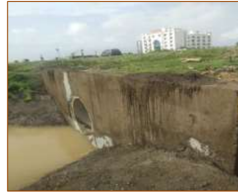
HPC at km. 490+350 (LHS)
