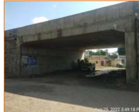
Side view of LVUP at km. 114.080 (RHS)
