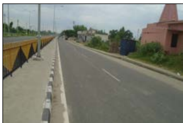
Service Road at km. 77+600 (LHS)
