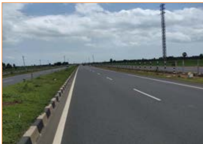
Pavement Condition at km. 71+300
