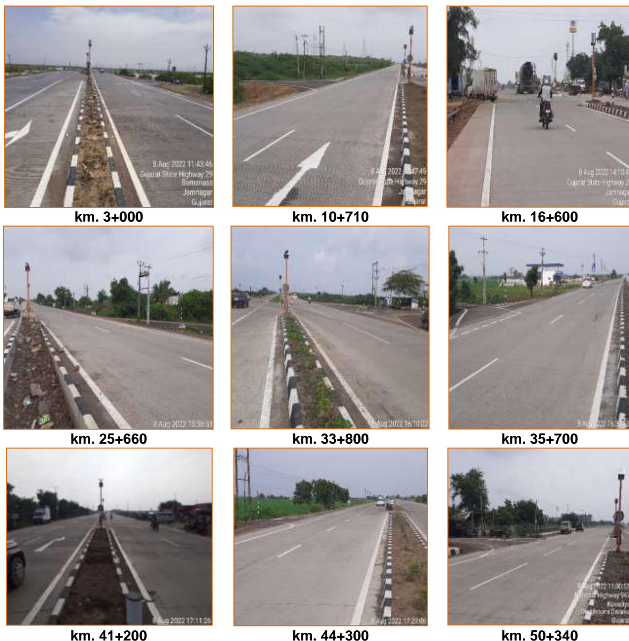
Figure 3-2 Photographs of Minor Intersection
