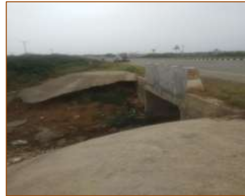
Slab culvert at km. 441+648 (LHS)
