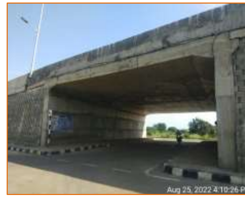
Side view of LVUP at km. 111.260 (RHS)
