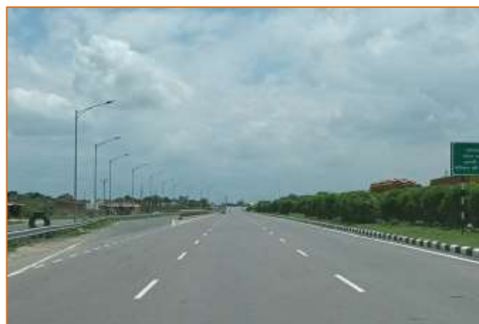
Truck Lay Bye at km. 767+330
