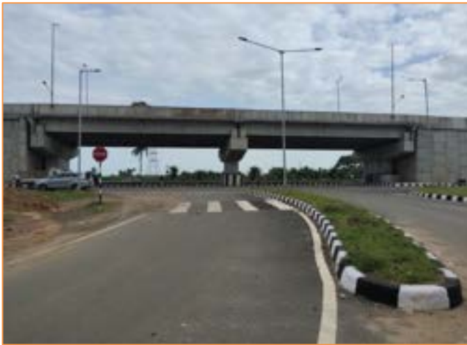
Highway Lighting at km. 45+645
