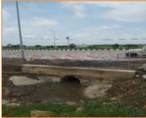
HPC at km. 5+800 (RHS)
