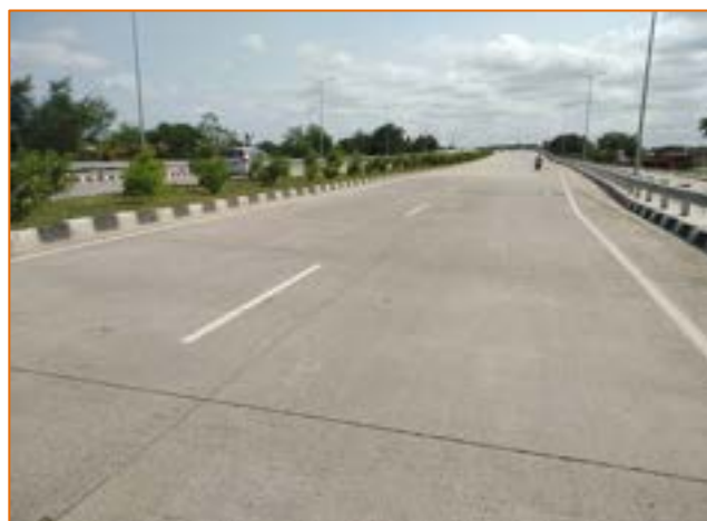
Start of Project Road at km. 276.000
