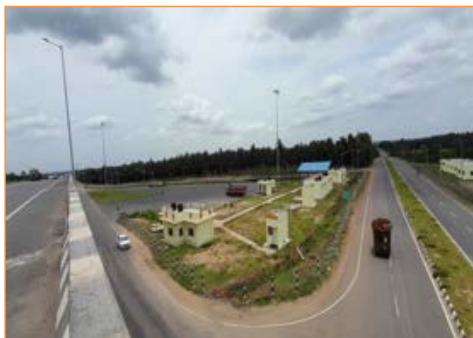
Rest Area at km. 66+800
