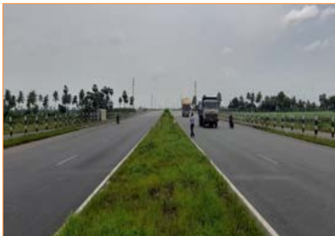
Pavement Condition at km. 41+200
