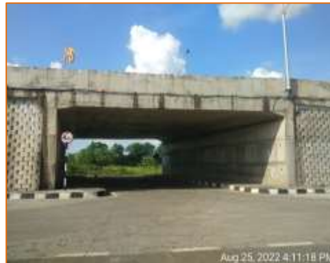
Side view of LVUP at km. 111.260 (LHS)
