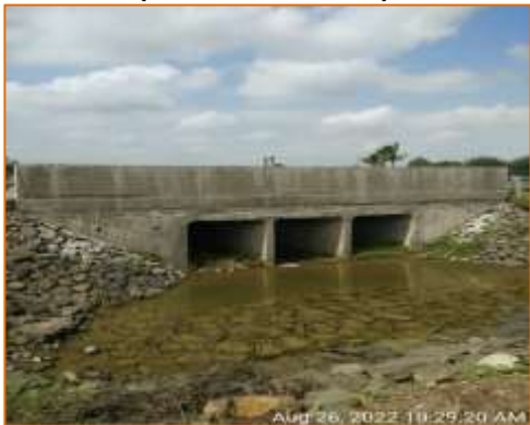
Box culvert at km. 128.229 - RHS (Reconstruction)
