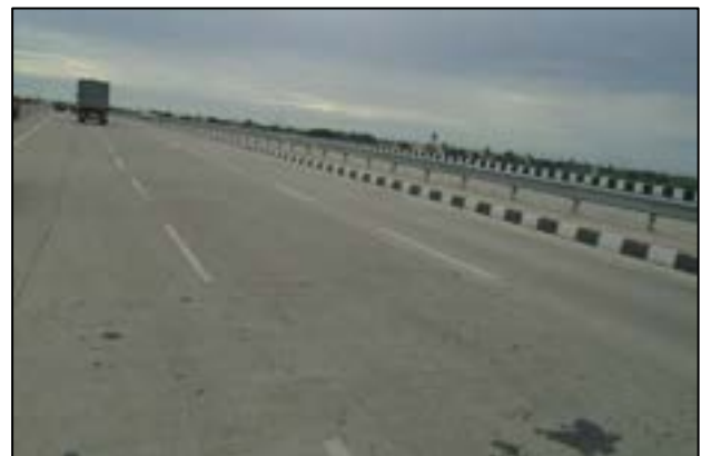
Crash Barrier at curve location
