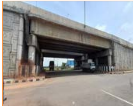
View of VUP at km 83+405
