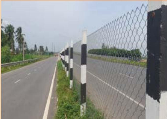
Chain fencing at km. 85+150
