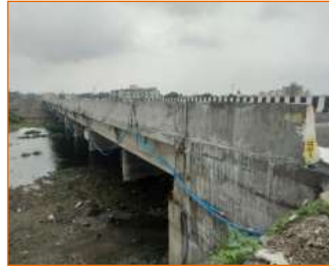
Side View of Major Bridge at km. 54+855 (LHS)
