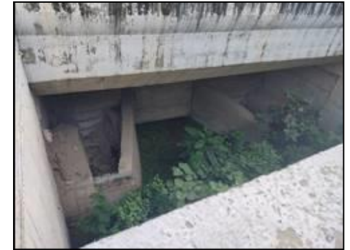
Minor Bridge at km. 69+815 (Existing Structure View)
