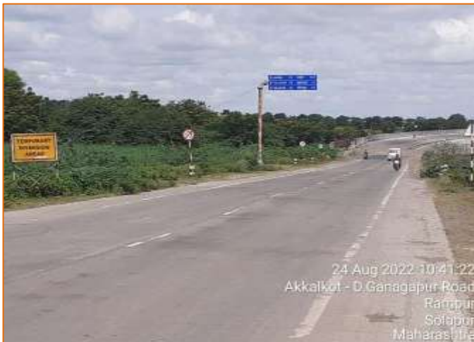
Start of the Project Highway at km. 99+400
