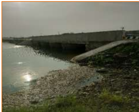
Side View of Minor Bridge at km. 45+893 (RHS)
