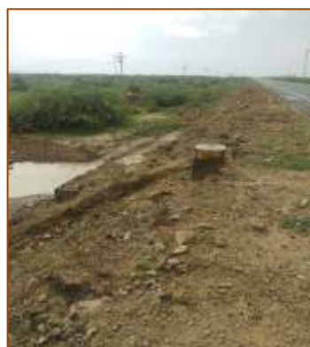
MJB at km. 487+054 (RHS)
