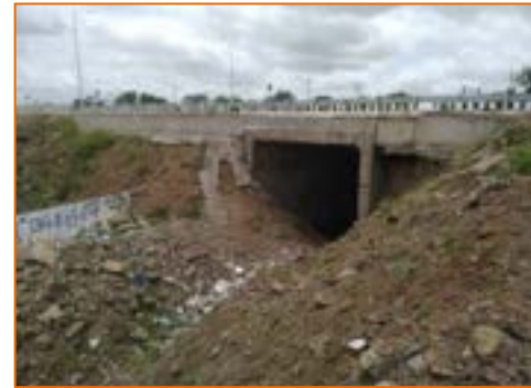
Box Culvert at km. 284+112
