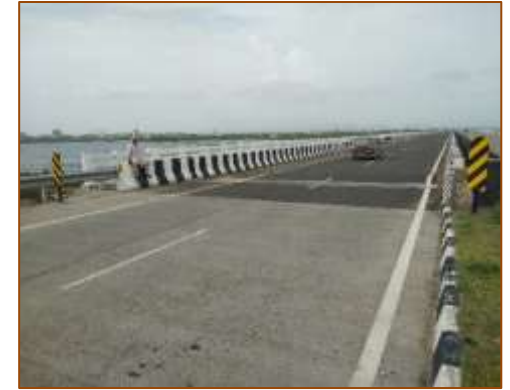
Wearing Coat of MJB at km. 386+750 (LHS)
