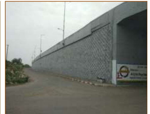
VUP at km. 396+865 (RHS) - A1 side
