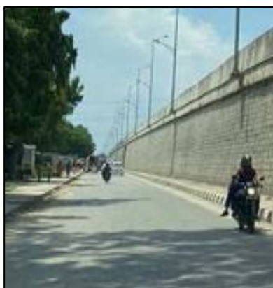
Service Road at km. 765+150
