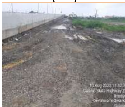
km. 11+800 to km. 13+100 (RHS)
