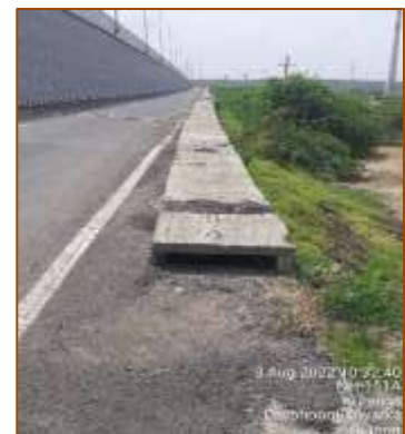
Built-up drain from km. 467+601 to km. 468+347 (LHS)
