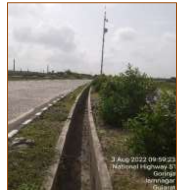
Median longitudinal drain from km. 483+000 to km. 484+000
