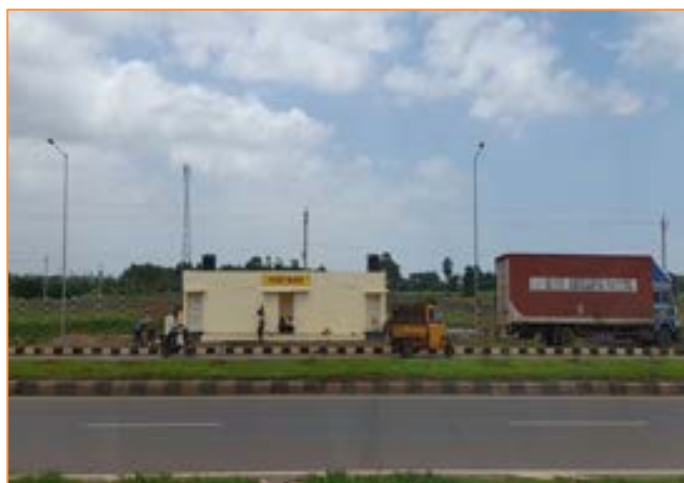
Truck Lay bye at km. 16+520
