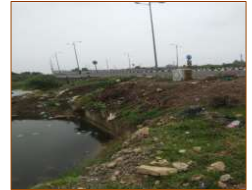
HPC at km. 391+096 (RHS)
