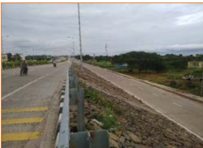
Slope Protection work at km. 284+500.000
