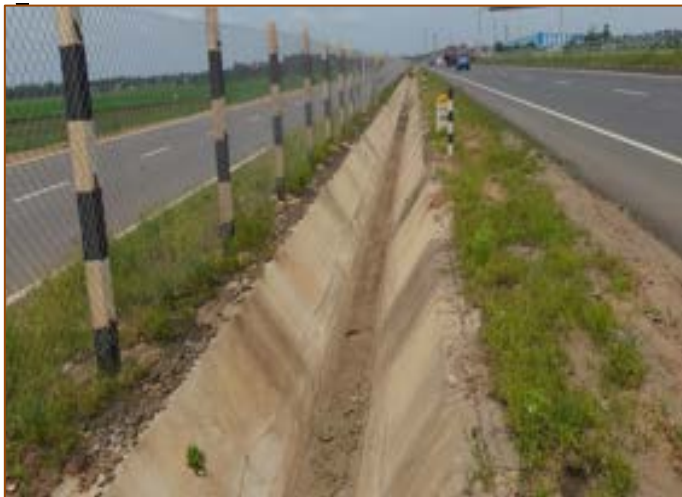
V Drain at km. 78+900
