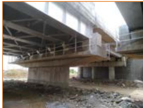
Rail Over Bridge at km. 294.125
