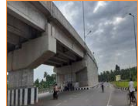
View of UDFO at km. 48+830
