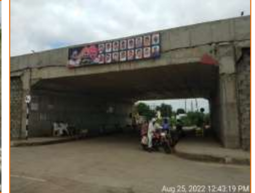
Side View of LVUP at km. 121.950 (LHS)
