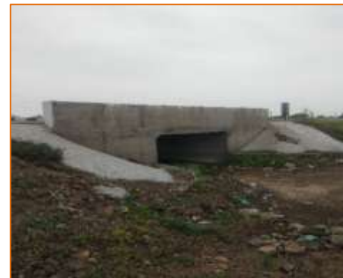
Box culvert at km. 62+720 (LHS)
