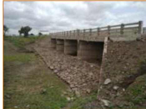
New Minor Bridge at km. 282.548
