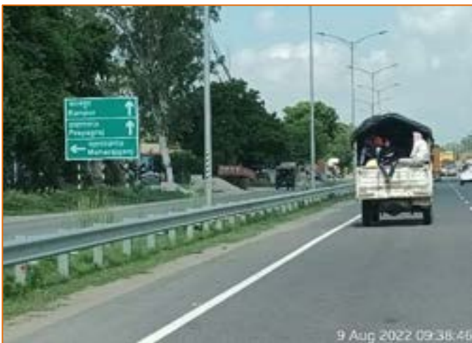
Sign Board at km. 767+100.
