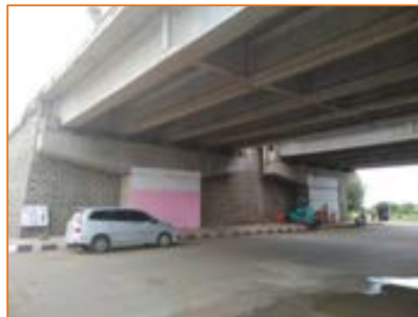
Vehicular Underpass at km. 292.230
