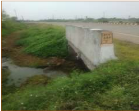
Slab culvert at km. 439+458 (LHS)
