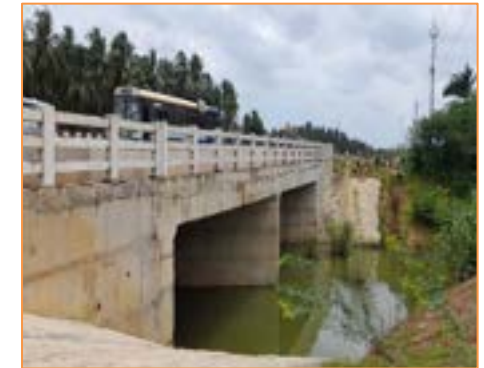
View of Minor Bridge at km. 30+774
