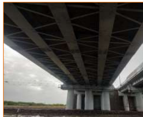
Bottom View of ROB's Girders at km. 0+527
