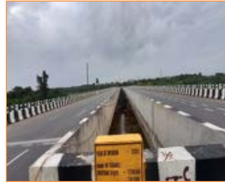
View of Major Bridge at km. 51+929
