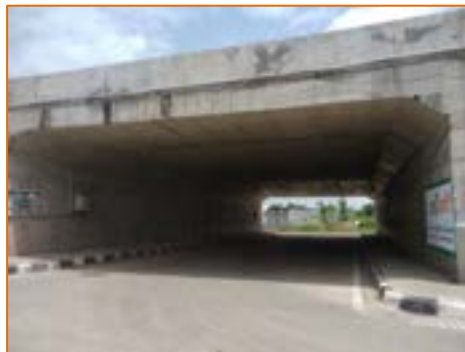
Light Vehicular Underpass at km. 276.900
