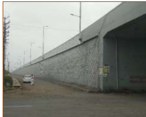
VUP at km. 400+681 (RHS) at A1 side
