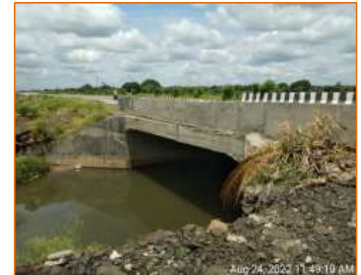
Side View of Minor Bridge at km. 104.348 (LHS)
