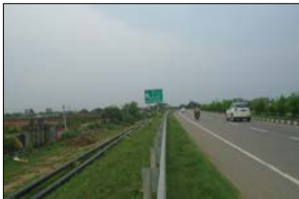
Crash Barrier at high embankment
