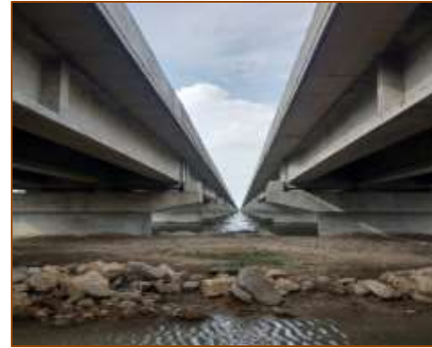
Mid Portion of MJB at km. 386+750
