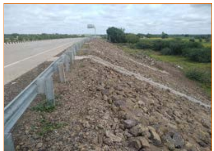
Slope Protection work at km. 298+300
