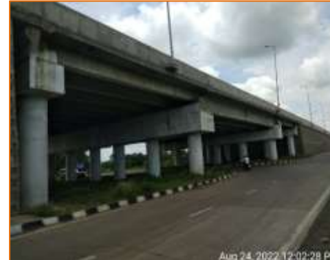
Side View of Flyover at km. 106.240 (RHS)
