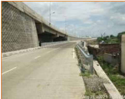
Side View of Minor Bridge at km. 117.796 - LHS (MCW & SR)
