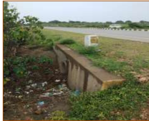
HPC at km. 380+328 (RHS)
