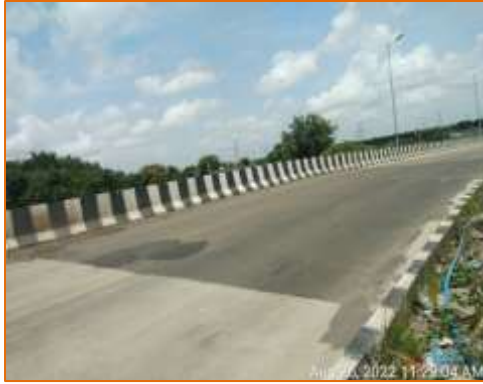
LVUP at km. 114.080 (LHS)
