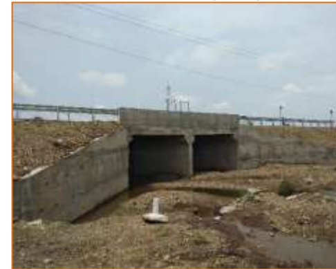
Side View of Minor Bridge at km. 64+765 (RHS)
