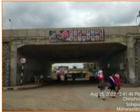
Side View of LVUP at km. 121.950 (RHS)
