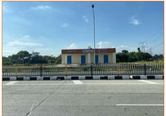
Rest Area at km. 767+500
