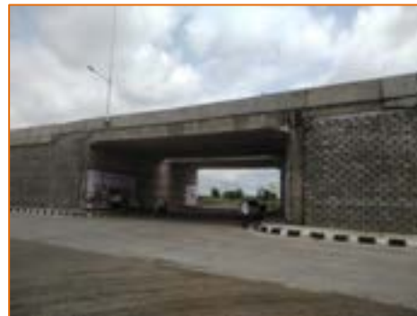
Vehicular Underpass at km. 292.758
