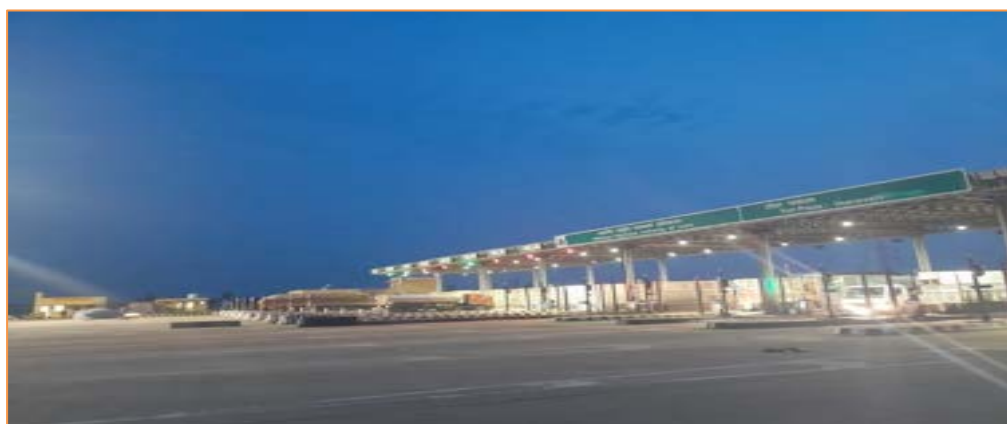
Figure 3-13 View of Toll Plaza
