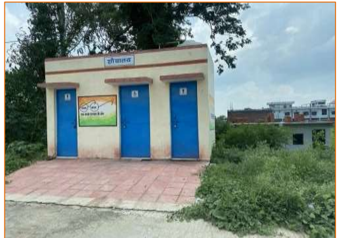
Toilet Block at km. 768+420
