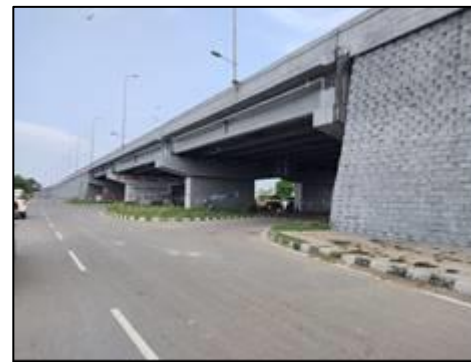
Flyover at km. 9+335
