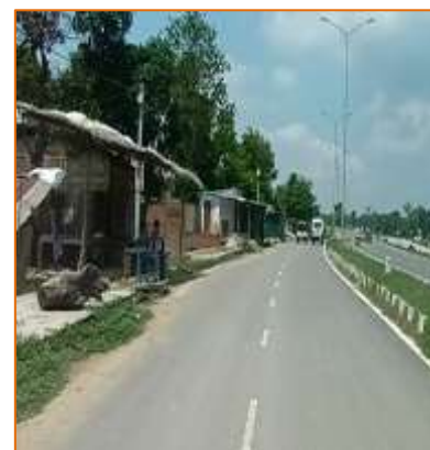
Service Road at km. 780+750
