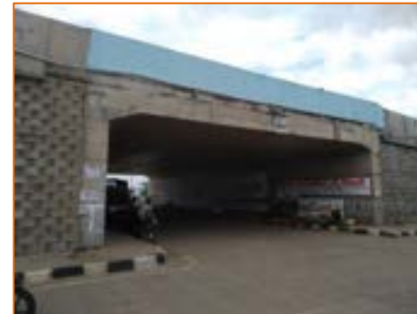
Light Vehicular Underpass at km. 283.165
