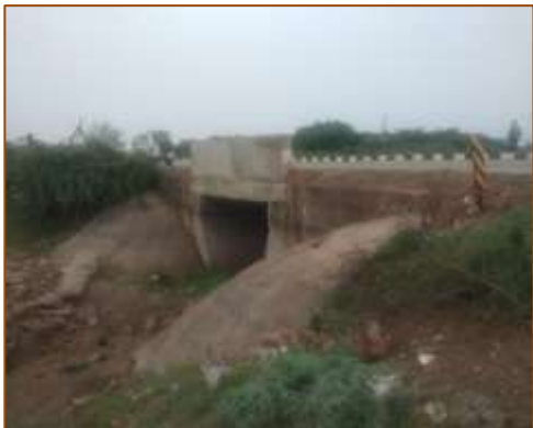
Slab culvert at km. 444+062 (LHS)
