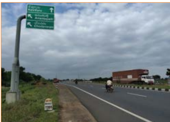
Cantilever Sign at km. 67+000
