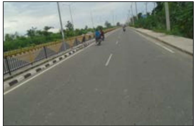
Pedestrian Guard Rail at km. 69+400
