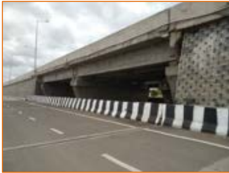
New Minor Bridge at km. 288.035
