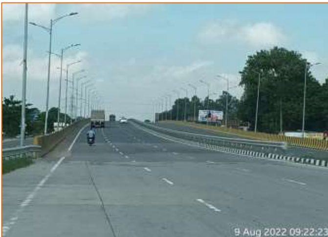
Highway Lighting at km. 773+100
