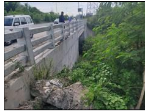
Minor Bridge at km. 69+815 (New Structure View)
