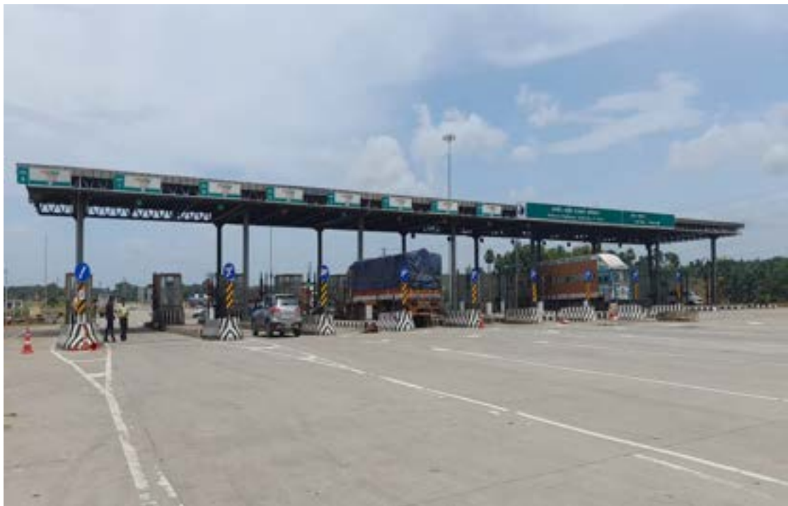
Figure 9-1 View of Toll Plaza (km. 53+700)
