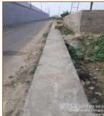
Built up drain from km. 489+000 to km. 490+000 (RHS)
