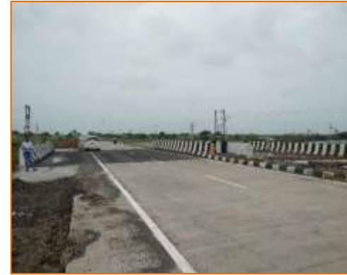
Wearing Coat of Minor Bridge at km. 13+410 (LHS)
