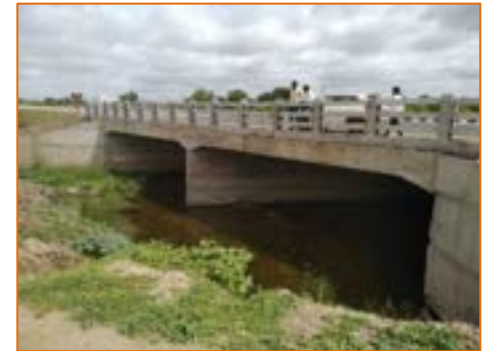
New Minor Bridge at km. 295.622
