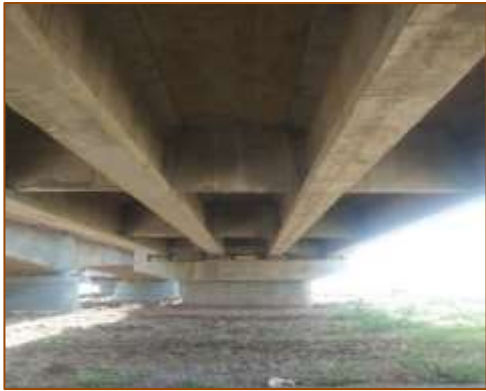
Bottom of MJB - New at km. 433+276 (LHS)
