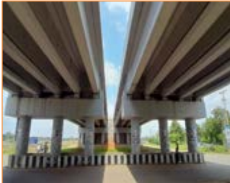
View of Flyover at km. 23+164
