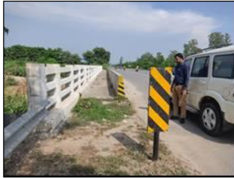
Minor Bridge at km. 66+020 (Top View)
