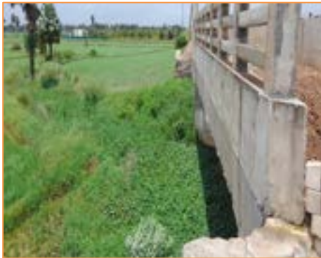
View of Minor Bridge at km. 24+603
