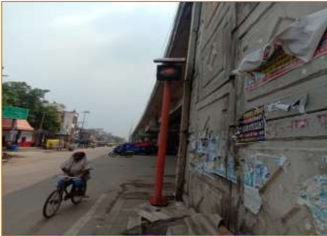
LED Blinker at km. 741+010
