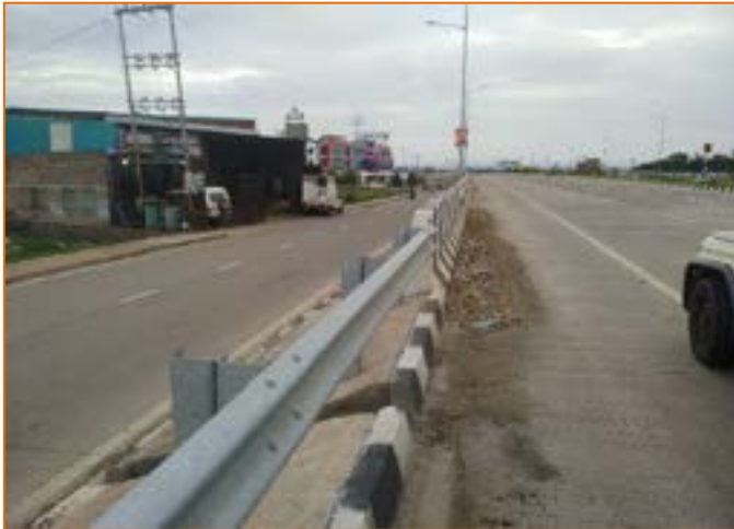
Crash Barrier at km. 285+650
