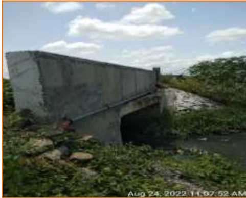
Box culvert at km. 101.823 - LHS (New Construction)
