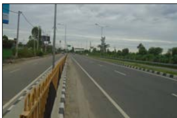
Approach to End of Project Road
