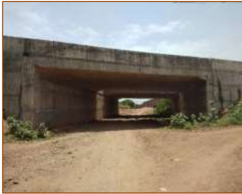
LVUP at km. 381+600 (RHS) - Under COS
