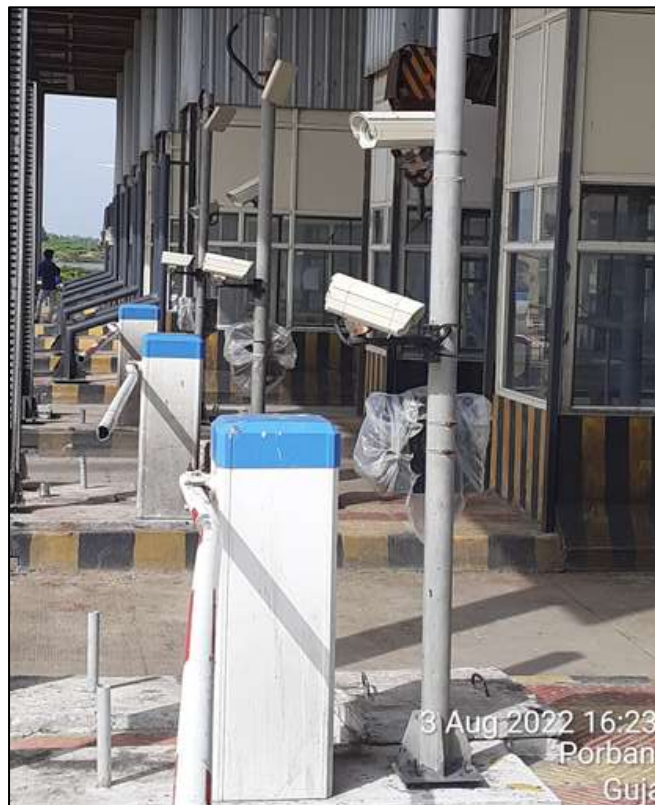
Figure 9-8 LPIC and AVC cameras
