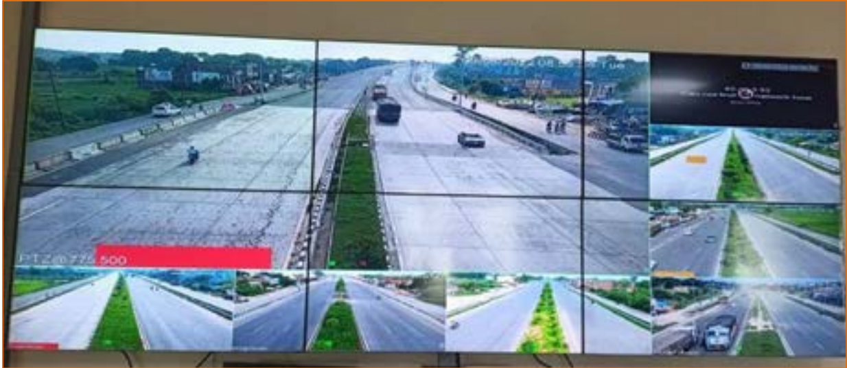
Figure 9-10 Video wall in ATMS control centre
