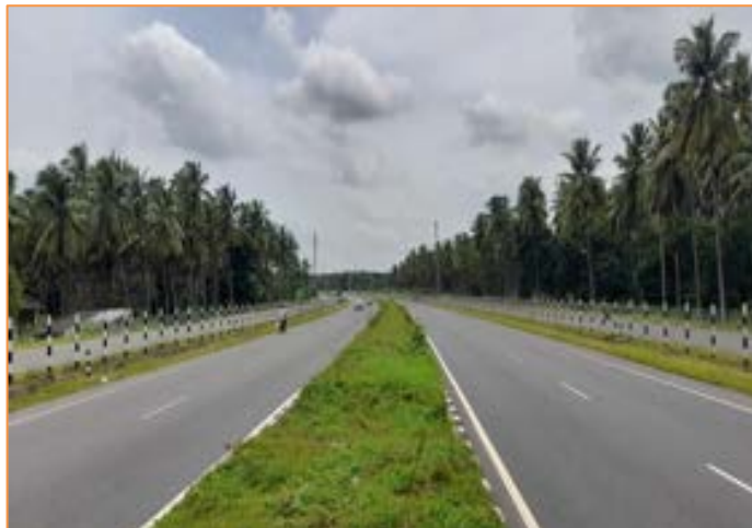
Pavement Condition at km. 46+700
