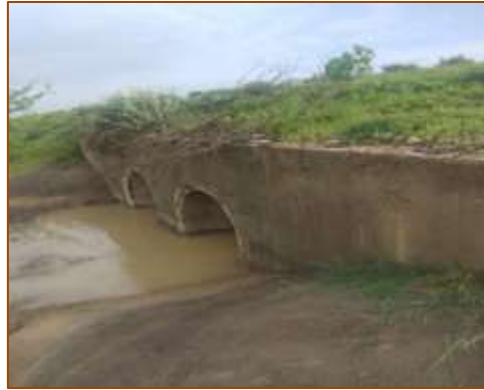
HPC at km. 487+054 (RHS)
