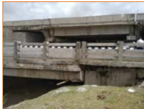
New Minor Bridge at km. 292.148
