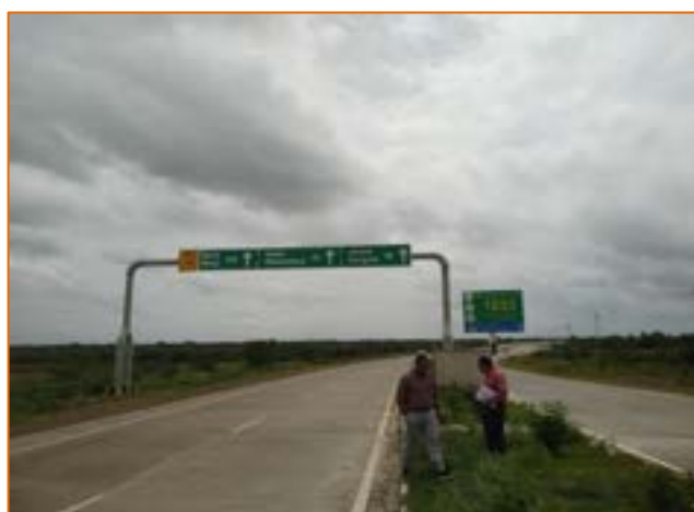
End of Project Road km. 321.600
