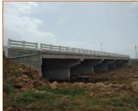
Side View of Minor Bridge at km. 450+241 (LHS) - New
