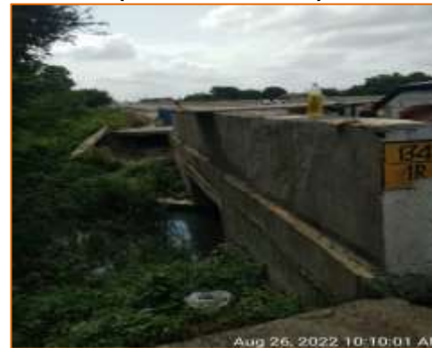
Box culvert at km. 133.524 - RHS (Reconstruction)
