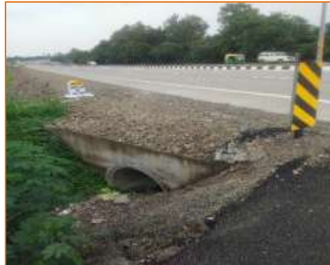
HPC at km. 66+010 (LHS)
