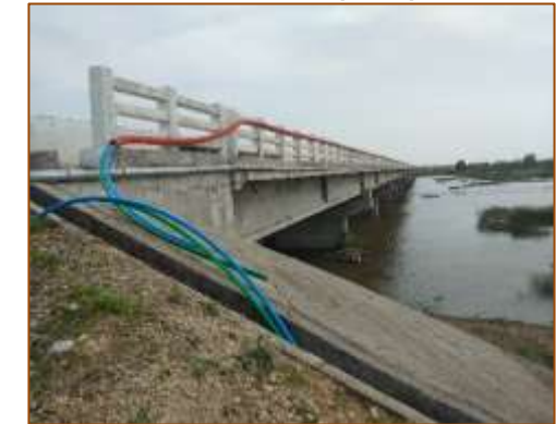
Side View of Major Bridge at km. 389+295 (LHS)
