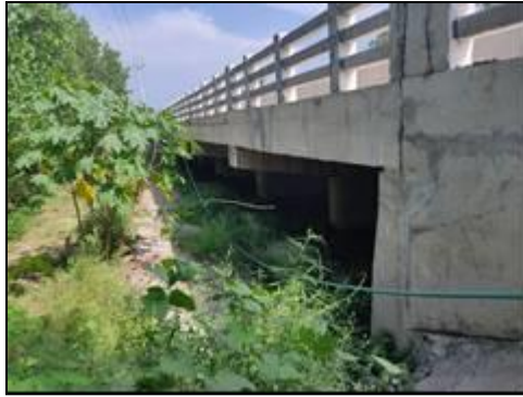
Minor Bridge at km. 64+791 (New Structure View)
