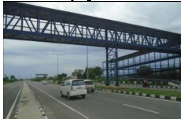
Foot Over Bridge (FOB) at km. 6+600
