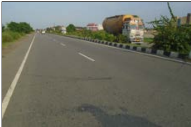
Pavement Condition at km. 6+950
