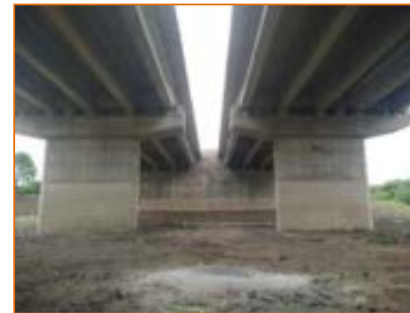
New Major Bridge at km. 298.190
