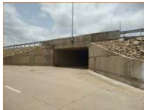
Pedestrian Underpass at km. 284.500
