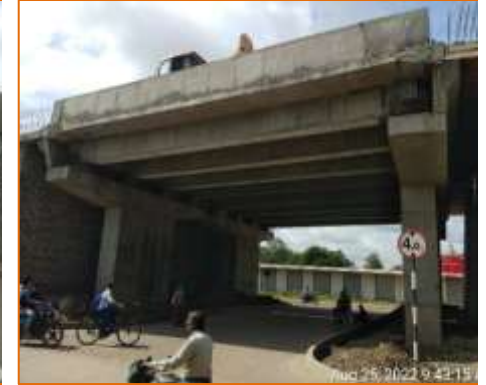
Side View of PUP at km. 136.657 (RHS)
