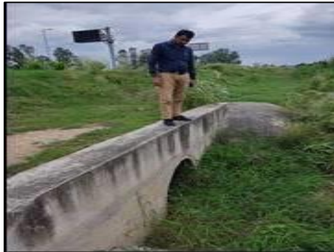
HP Culvert at km. 69+420
