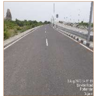
km. 390+177 to km. 390+953 (RHS)
