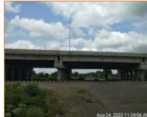
Side View of Flyover at km. 102.700 (RHS)
