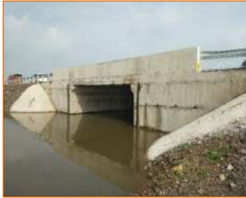
Side View of Minor Bridge at km. 34+400 (LHS)
