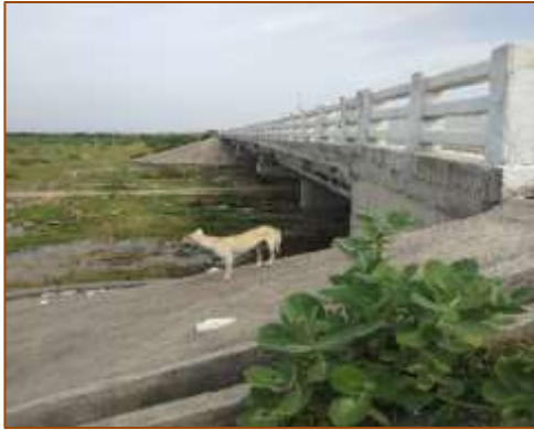
Side View of Major Bridge at km. 395+255 (RHS)
