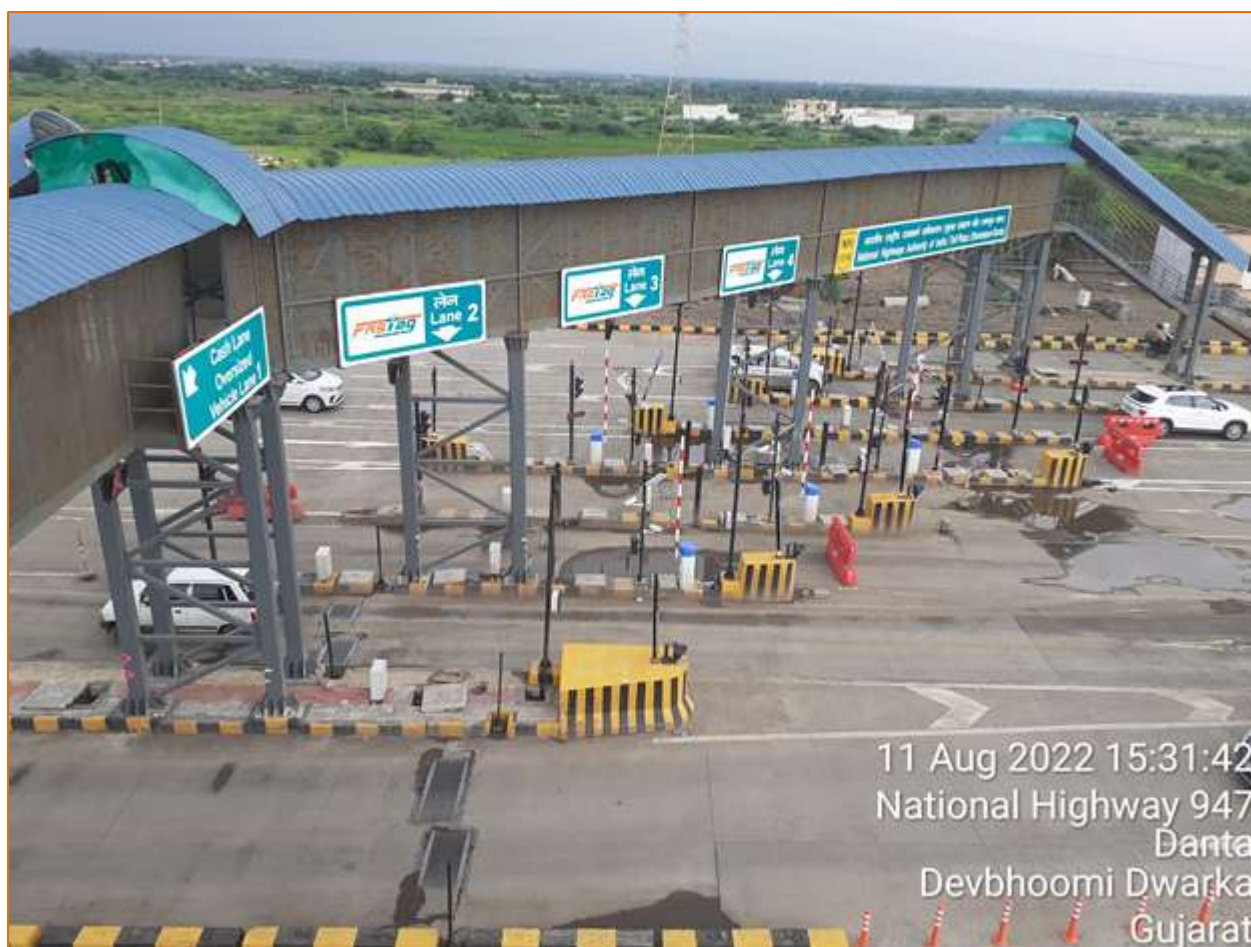
Figure 8-1 Views of Dharampur Dante Toll Plaza
