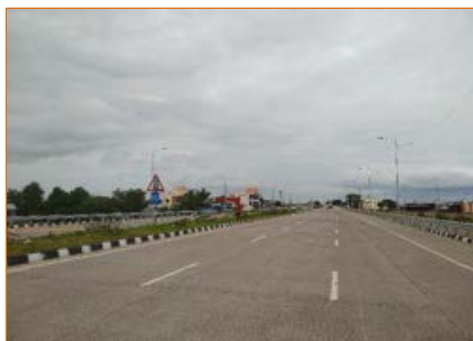
Road Markings at km. 286+600
