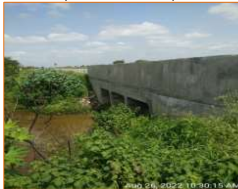
Box culvert at km. 128.229 - LHS (Reconstruction)
