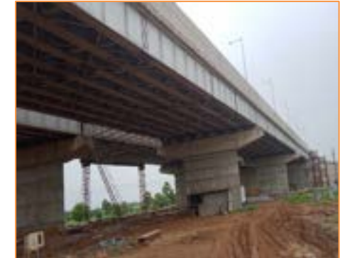
View of ROB at km. 18+677
