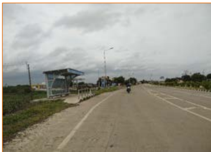
Bus Bay at km. 312+150 (Andhalgaon)
