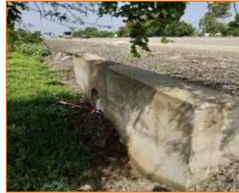
HPC at km. 32+520 (RHS)
