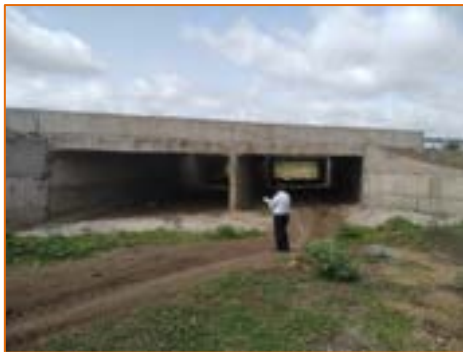
New Minor Bridge at km. 296.580
