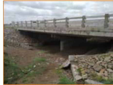
New Minor Bridge at km. 289.260
