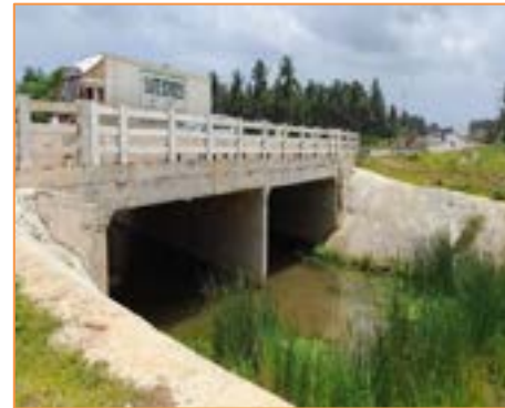
View of Minor Bridge at km. 28+782
