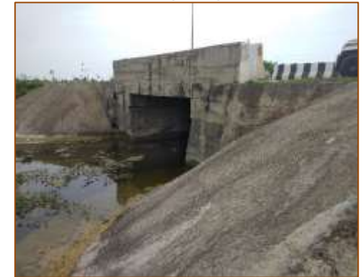
Side View of Minor Bridge at km. 460+812 (LHS) - New
