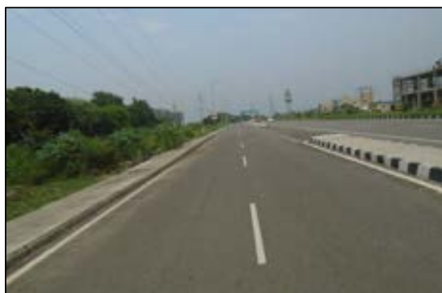
Service Road at km. 0+630 (LHS)
