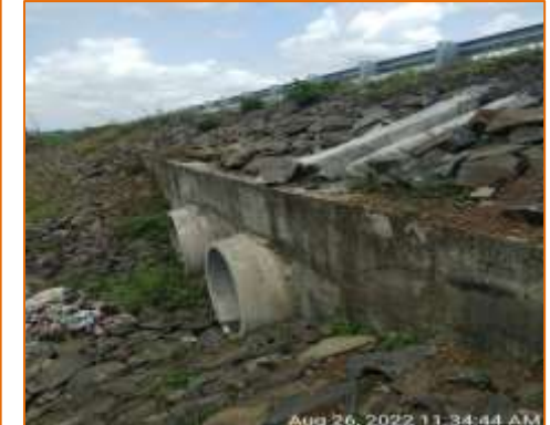
Pipe Culvert at km. 113.155-LHS (Widening)
