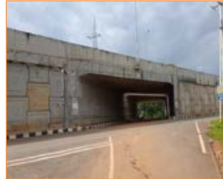
View of LVUP at km 44+135
