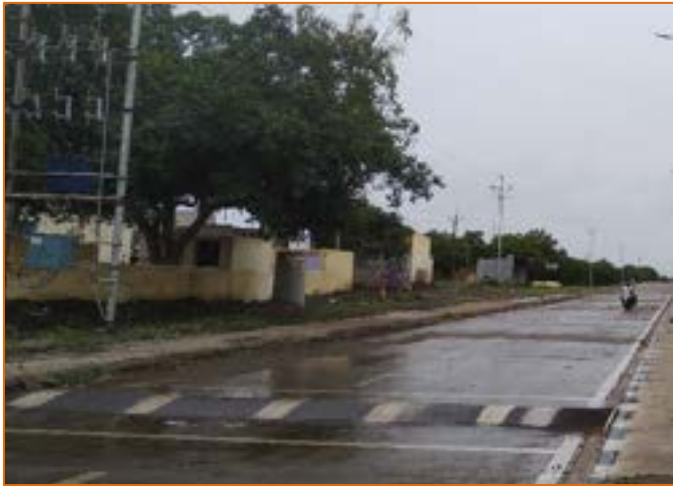
Built-up Drain at km. 314+735
