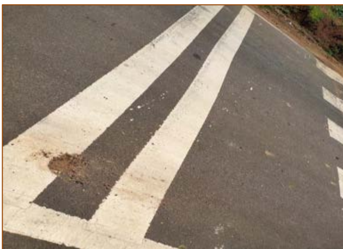
Road Markings at km. 29+400
