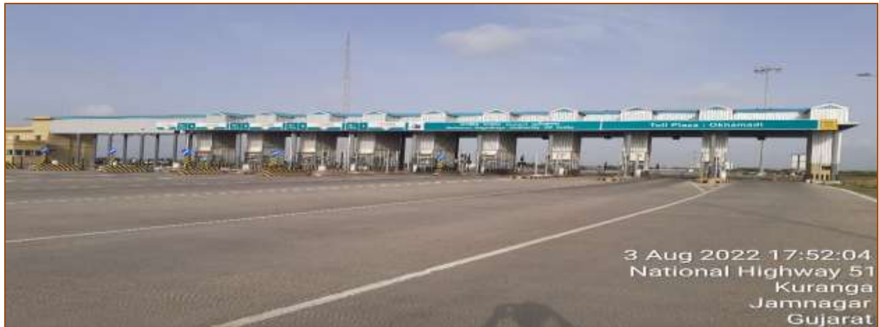
Figure 9-2 View of Okhamadi Toll Plaza
