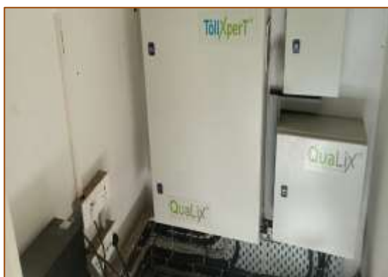
TP-1 at km. 409+500
