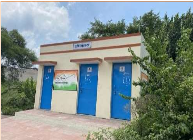
Toilet Block at km. 764+770
