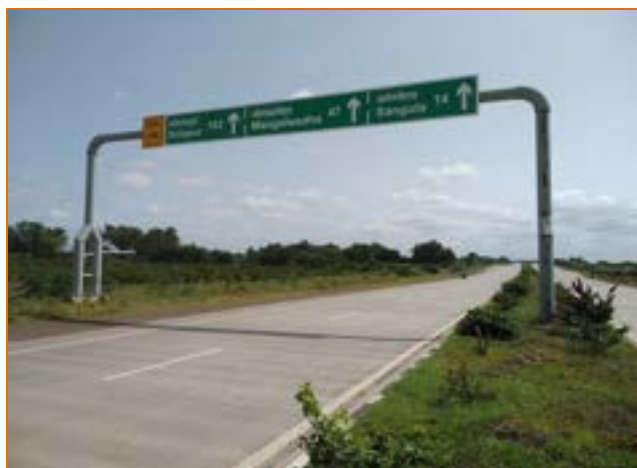
Start of Project Road at km. 276.000
