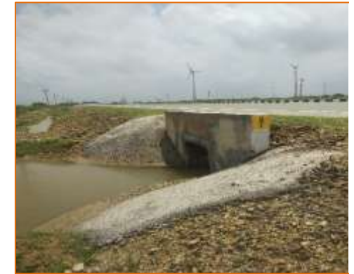
Box culvert at km. 7+240 (RHS)
