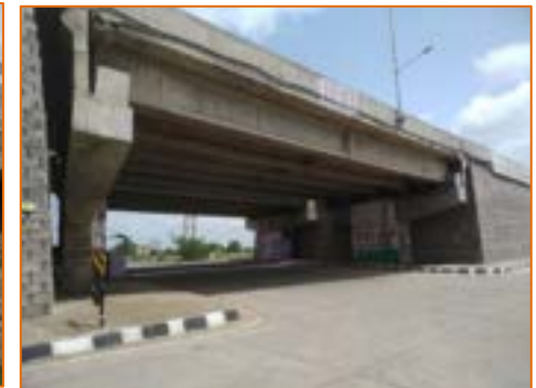
Vehicular Underpass at km. 290.700
