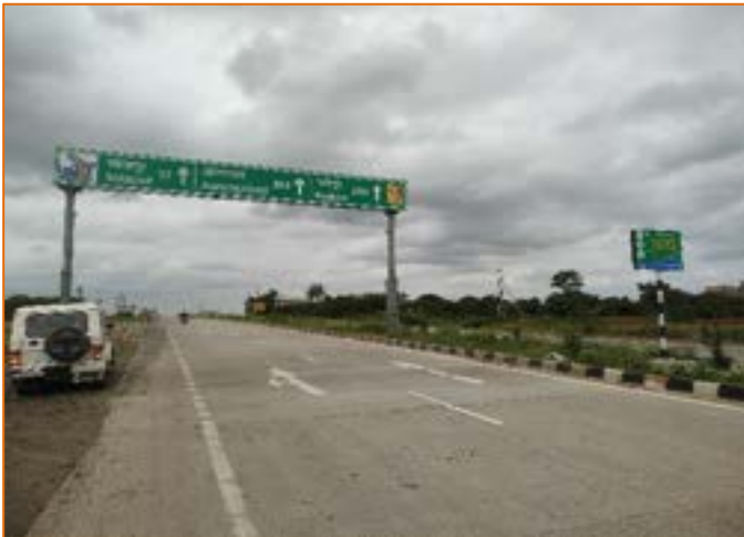
Cantilever Gantry Sign at km. 321+600
