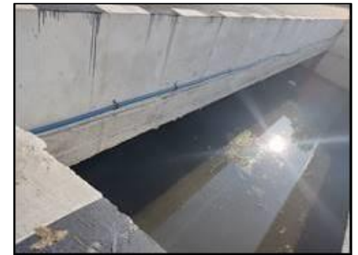
Minor Bridge at km. 71+727 (Structure View)
