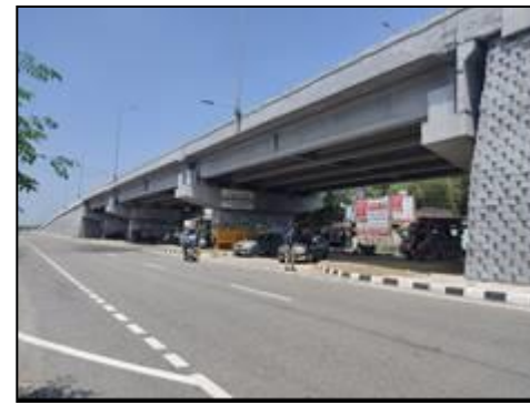
Flyover at km. 59+818
