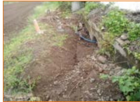
Pipe Culvert at km. 299+507
