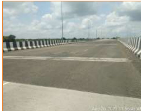
Flyover at km. 106.240 (LHS)
