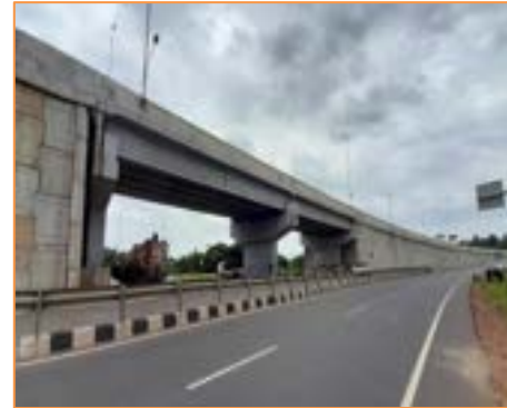
View of UDFO at km. 34+915
