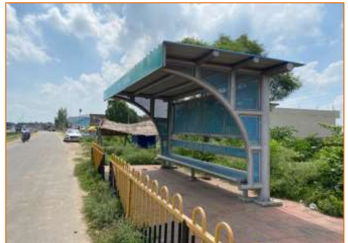
Bus Shelter at km. 767+915
