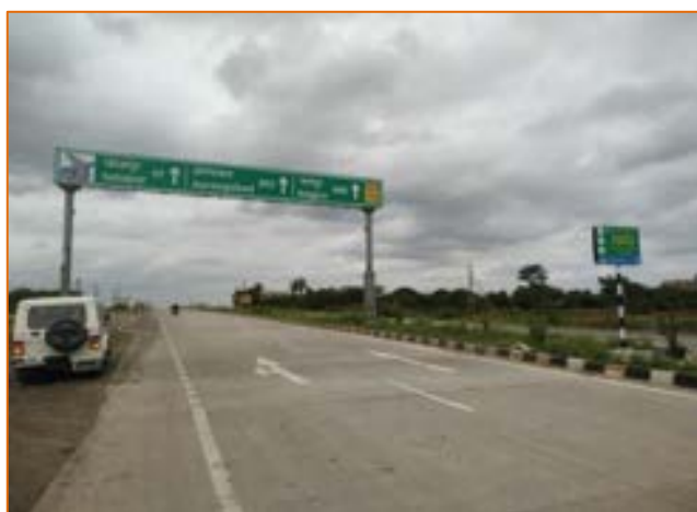
End of Project Road at km. 321.600
