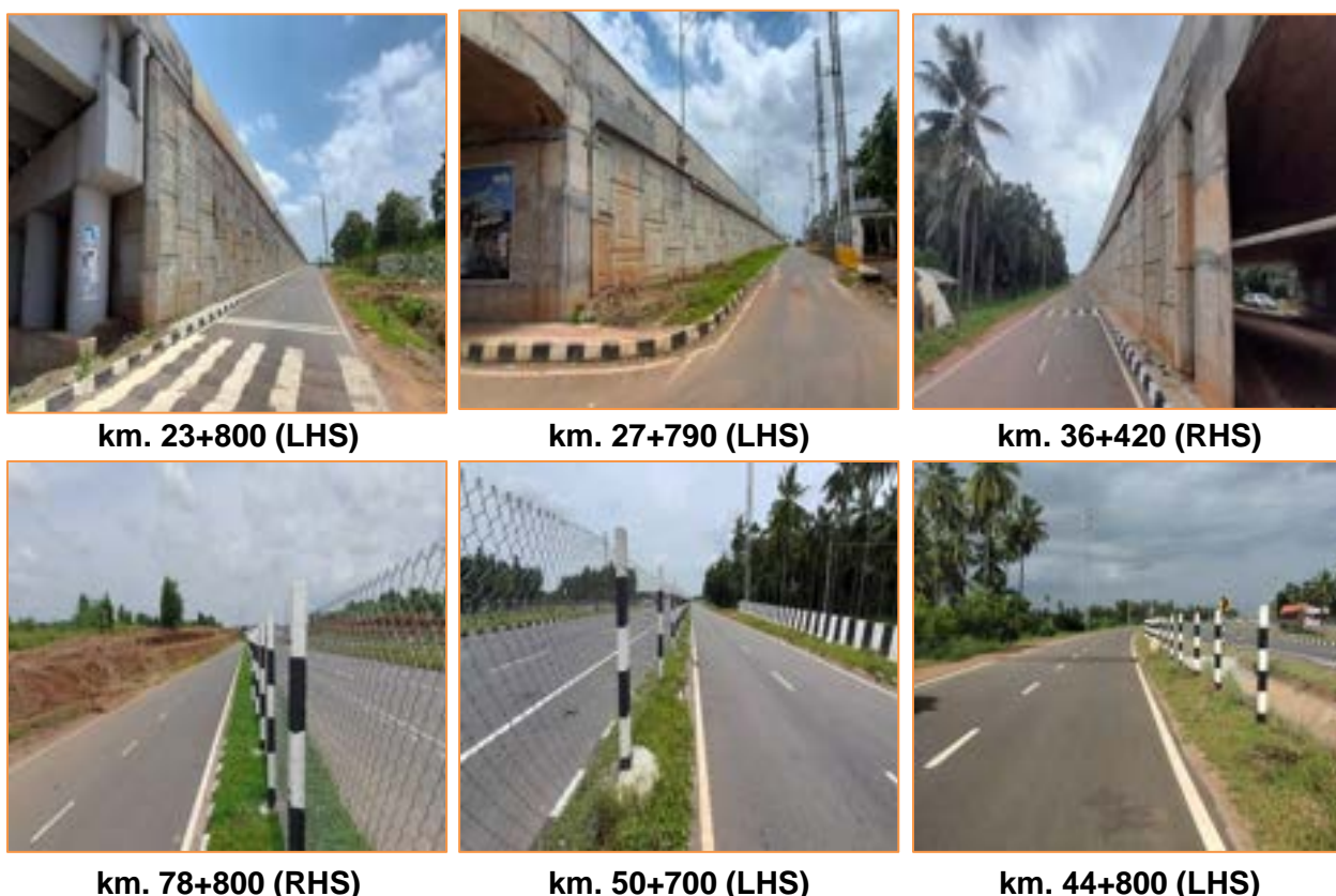
Figure 3-3 Photographs of Service Road
