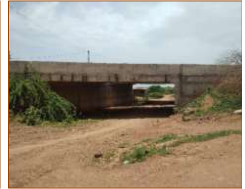
LVUP at km. 488+981 (RHS) - Under COS
