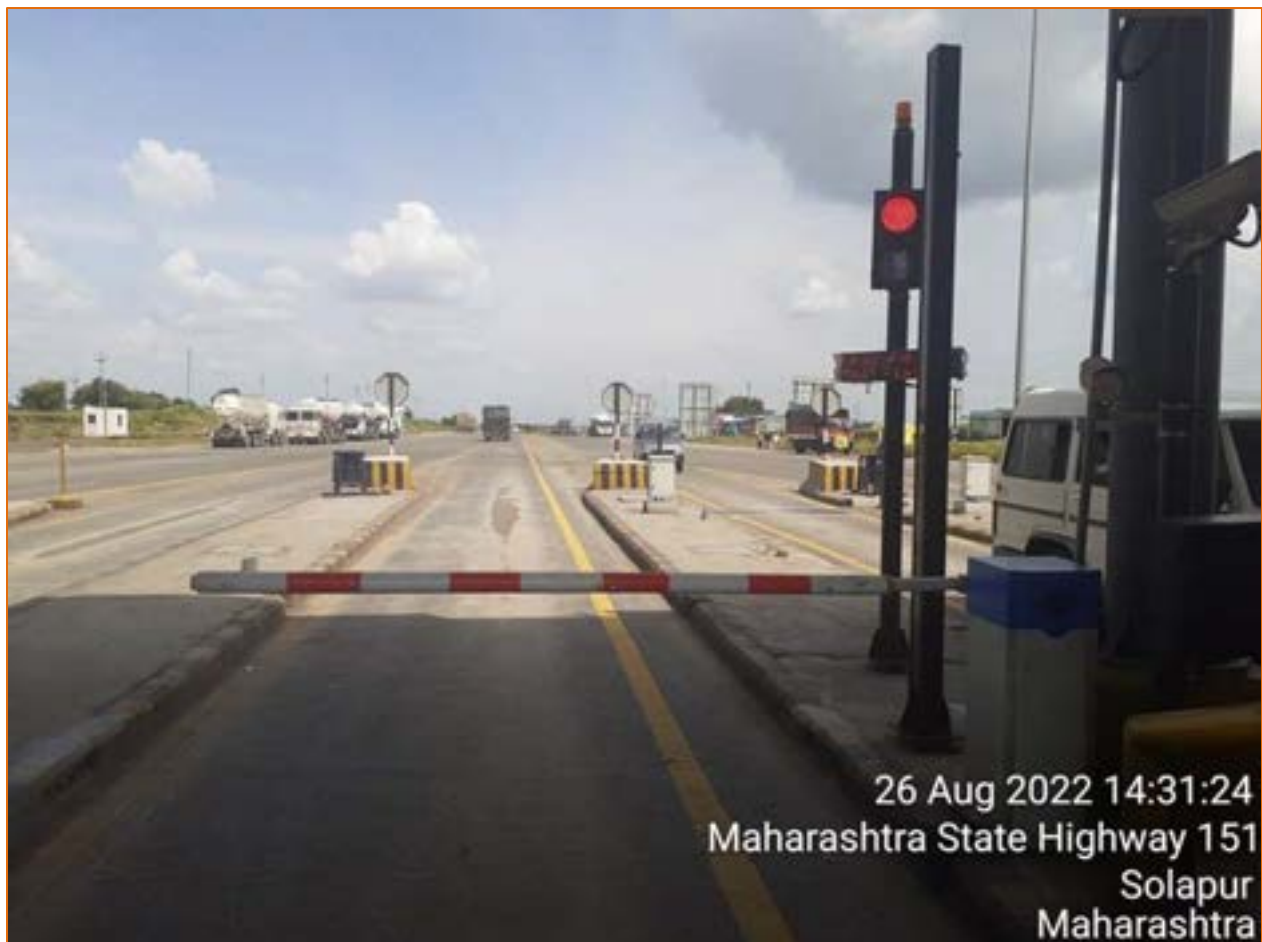
Figure 9-4 Automatic Lane Barrier
