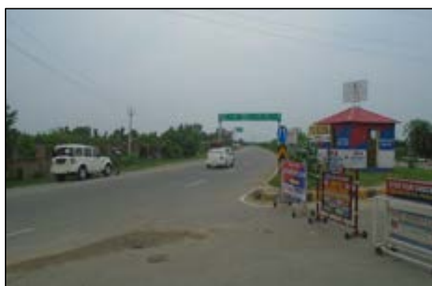
Start of Project Road - Left Carriageway
