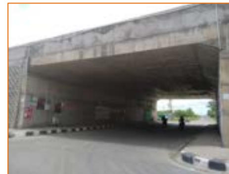
Light Vehicular Underpass at km. 285.432
