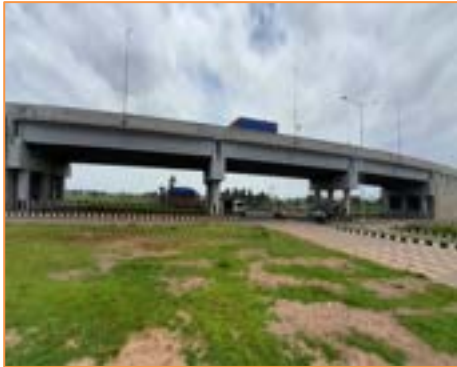
View of UDFO at km. 15+800
