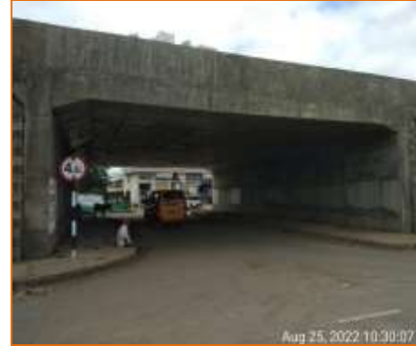
Side View of LVUP at km. 135.100 (LHS)
