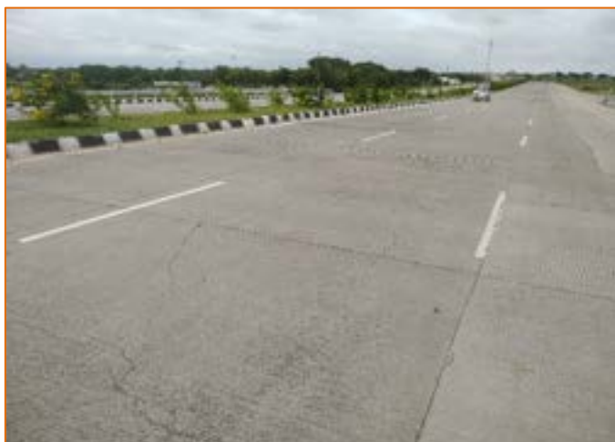
Road Markings at km. 306+500
