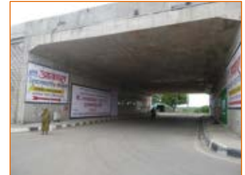
Light Vehicular Underpass at km. 283.650
