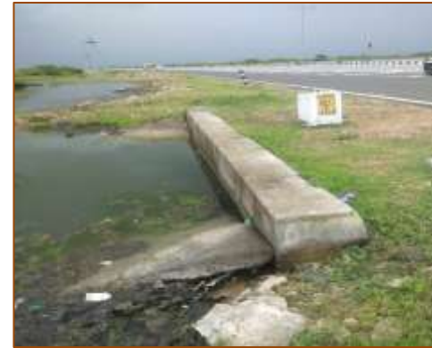
HPC at km. 391+096 (LHS)
