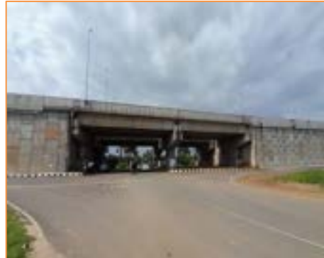
View of Flyover at km. 45+645
