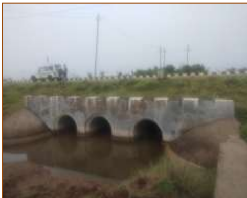
HPC at km. 437+025 (LHS)
