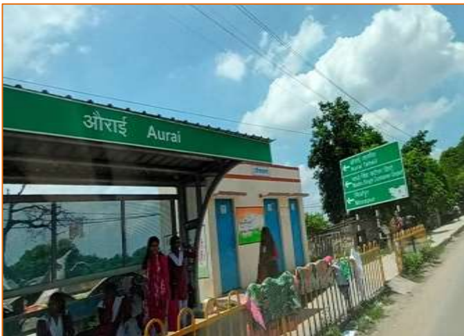
Toilet Block at km. 754+130
