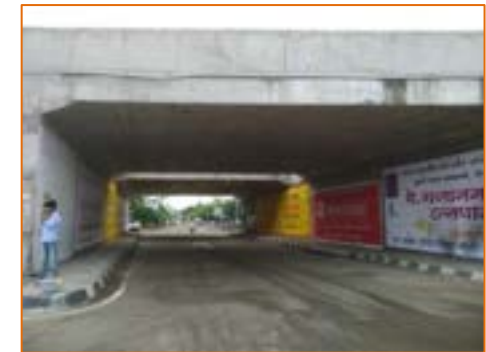
Light Vehicular Underpass at km. 298.613
