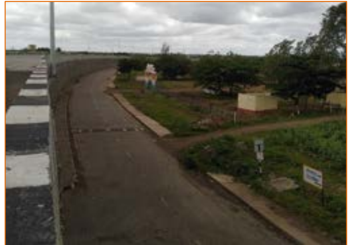
Built-up Drain at km. 299+350
