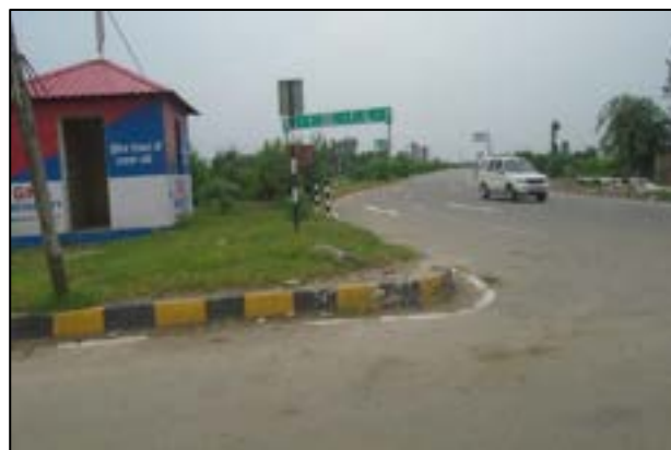
Start of Project Road - Right Carriageway
