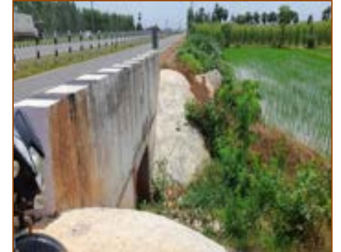
Box Culvert at km. 56+650
