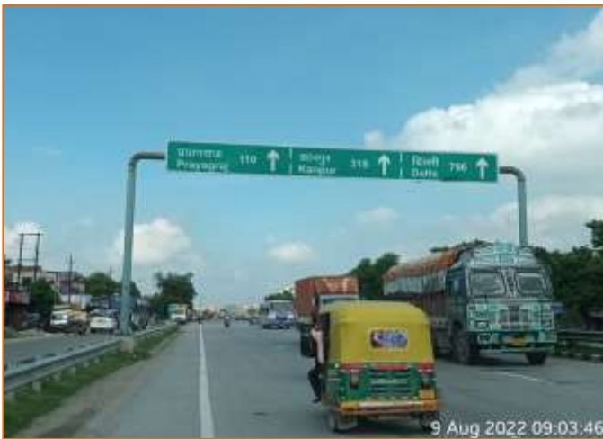
Overhead Gantry Sign at km. 785+040
