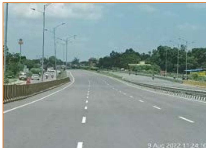
Pavement Condition at km. 722+100 (RHS)
