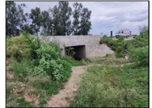
Box Culvert at km. 10+481
