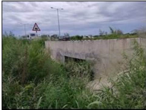
Box Culvert at km. 36+929
