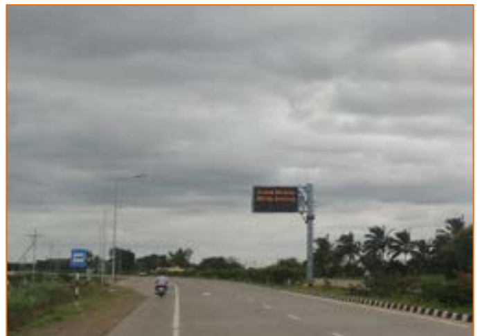
VMS Board at km. 301+100
