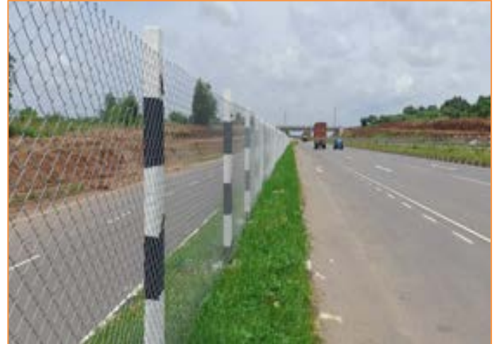
Chain fencing at km. 78+800
