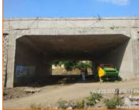
Side view of LVUP at km. 114.080 (LHS)
