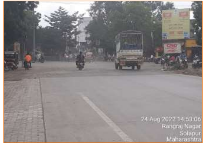
End of the Project Highway at km. 138+352
