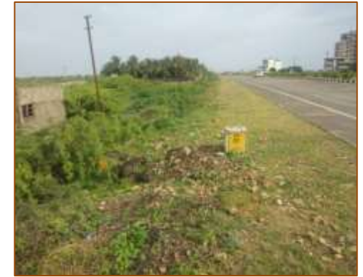
HPC at km. 490+350 (RHS)
