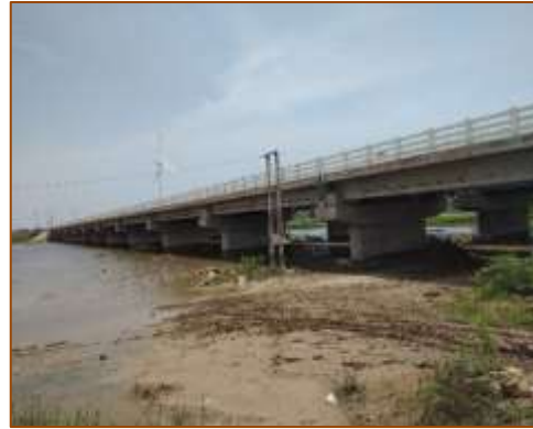
Side View of Major Bridge at km. 415+929 (RHS)
