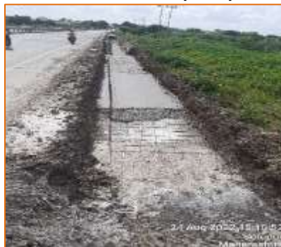
km. 133.300 WIP (RHS)
