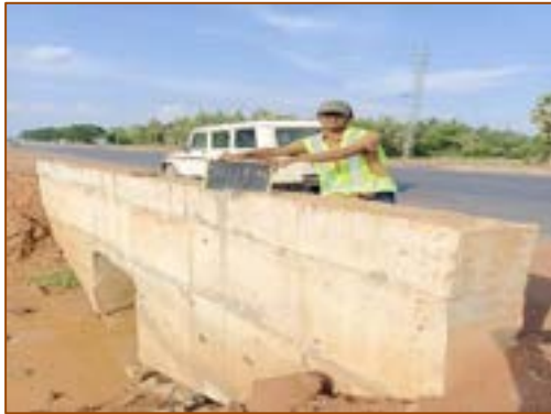
Box Culvert at km. 30+874
