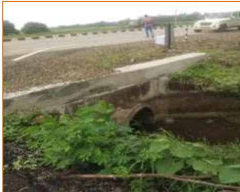
HPC at km. 66+010 (RHS)
