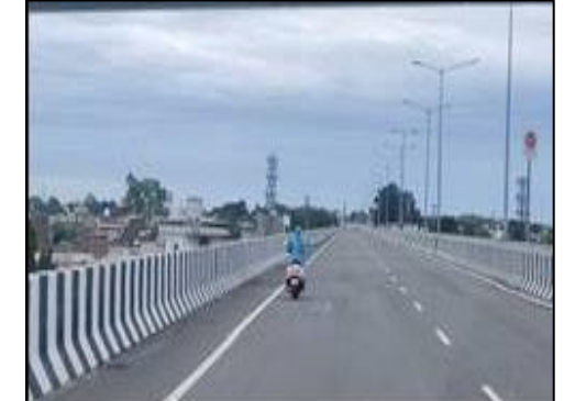
Elevated Structure at km. 25+319
