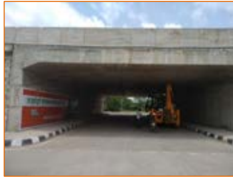
Light Vehicular Underpass at km. 288.116
