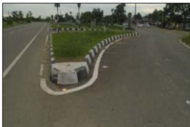
Major Junction at km. 57+260 (RHS)
