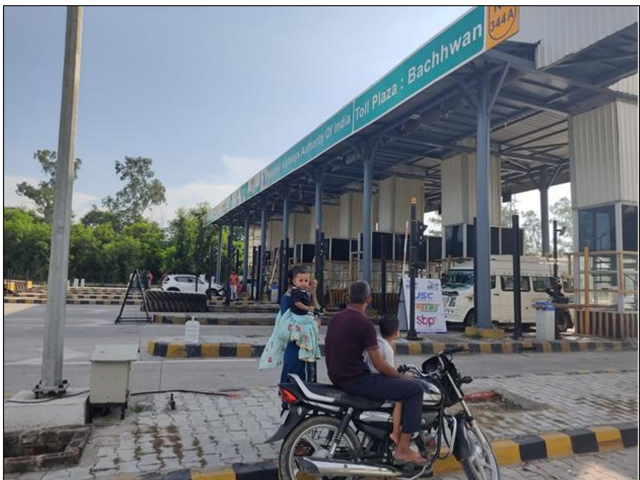
Figure 9-2 View of Bachhwan Toll Plaza (km. 70+240)
