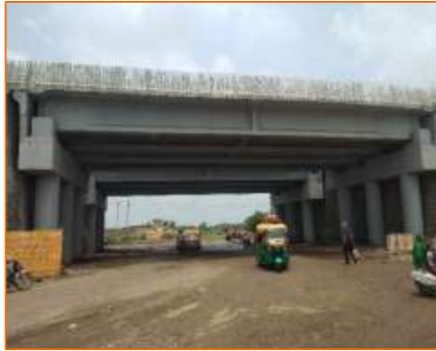
Side View of VUP at km. 57+975 (RHS)
