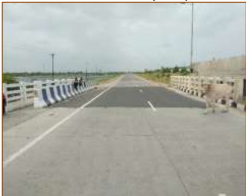
Minor Bridge at km. 406+170 (RHS) - Widening - Wearing Coat
