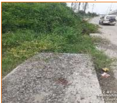
km. 121.470 (RHS) partially completed
