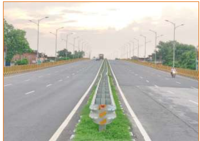
Highway Lighting at km. 740+300
