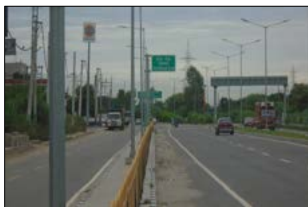
End of Project Road
