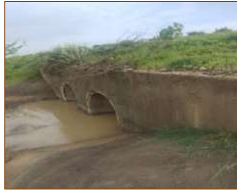
HPC at km. 487+054 (RHS)
