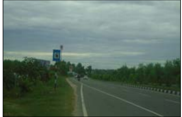
Traffic Sign Board at km. 72+000
