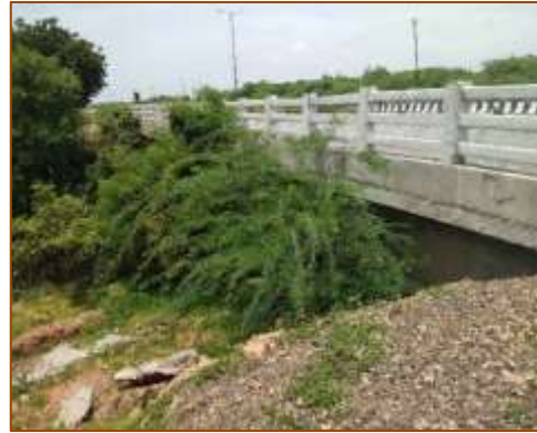
Side view of Minor Bridge at km. 427+321 (LHS) - Widening
