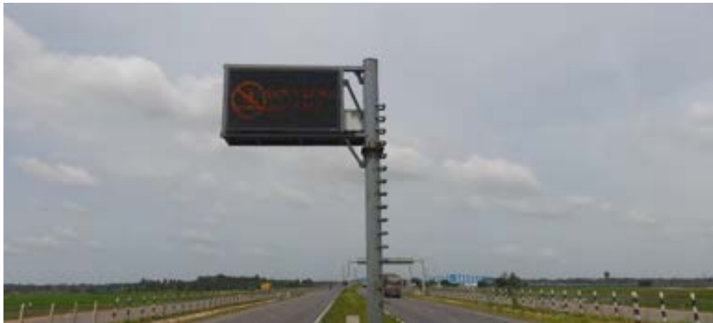
Figure 9-16 VMS on project highway
