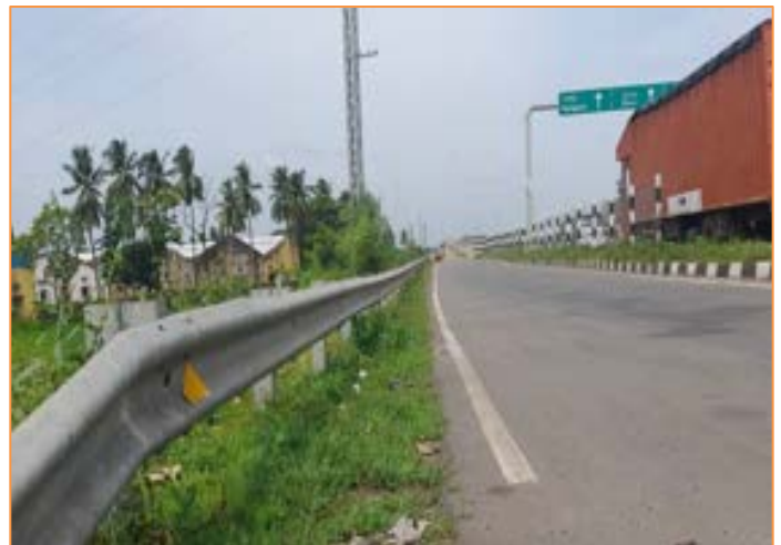
W beam Crash Barrier at km. 85+204
