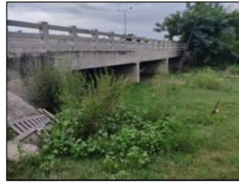
Minor Bridge at km. 72+900 (Structure View)
