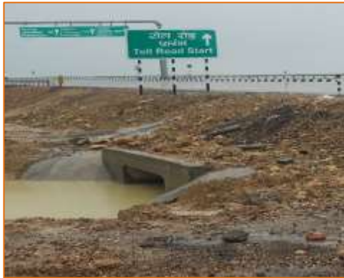
Box culvert at km. 0+060 (LHS)
