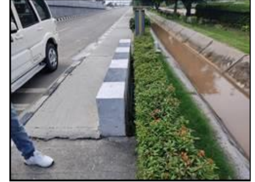
HP Culvert at km. 6+874
