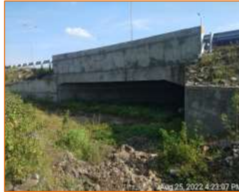
Side View of Minor Bridge at km. 110.930 (RHS)
