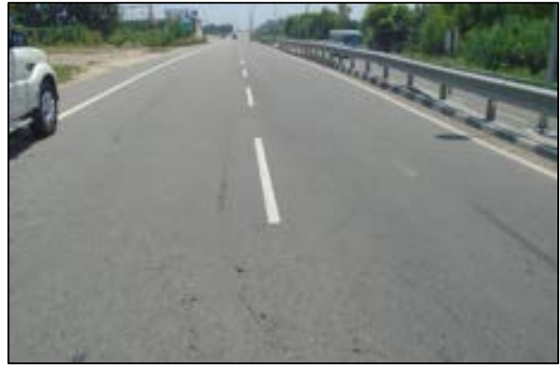
Pavement Condition at km. 59+000
