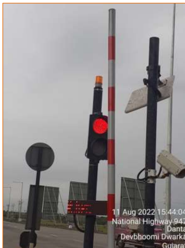
Figure 8-4 Lane Traffic Light (LTL) and User Fare Display (UFD)
