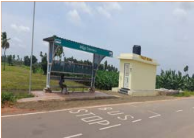
Bus Bay with Shelter at km. 79+200
