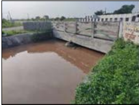
Minor Bridge at km. 35+812 (Existing Structure View)
