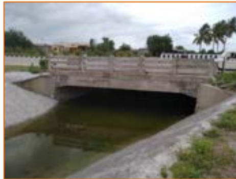
New Minor Bridge at km. 319.849 on LHS
