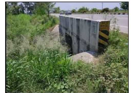
Box Culvert at km. 53+510
