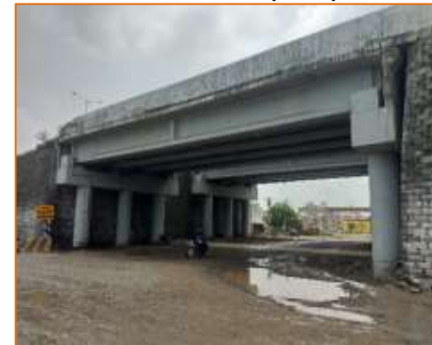
Side View of VUP at km. 57+975 (LHS)
