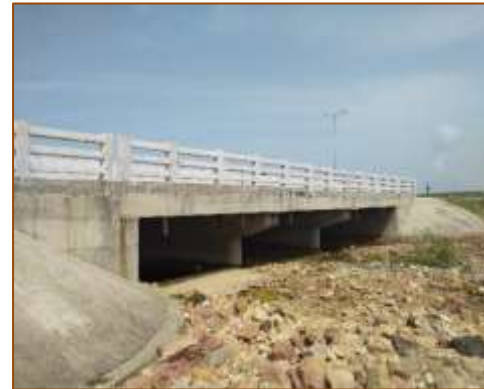
Side View of Minor Bridge at km. 480+171 (LHS) - Widening
