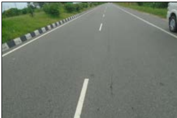
Pavement Condition at km.33+000
