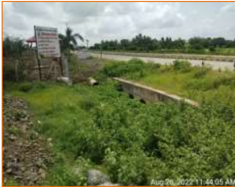
Pipe Culvert at km. 109.578 - RHS (Widening)
