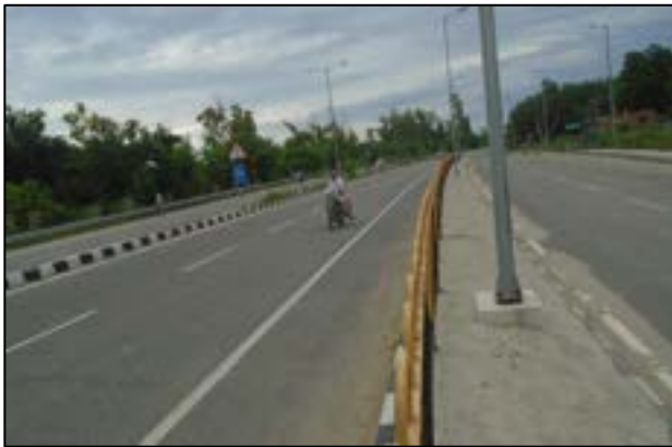
Pedestrian Guard Rail at km. 69+400
