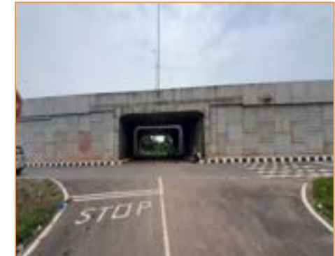
View of LVUP at km 61+932
