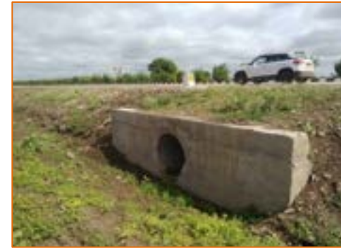
Pipe Culvert at km. 292+135
