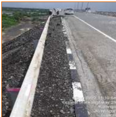
Figure 3-6 Photographs of Slope Protection Works
