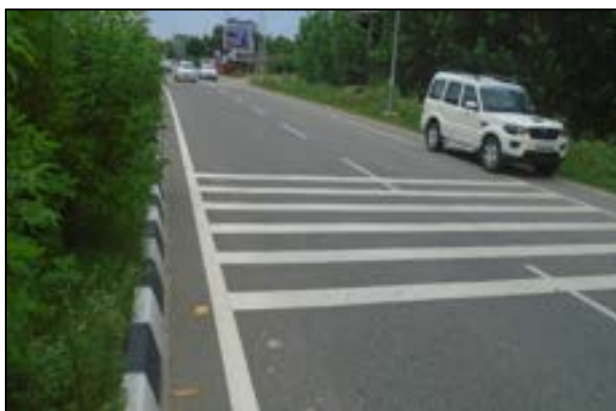
Road Marking at km. 70+000 (RHS)
