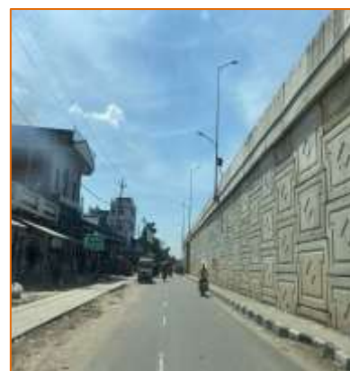
Service Road at km. 734+175
