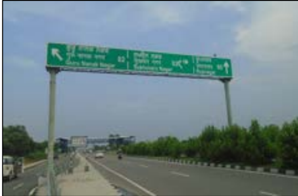
Overhead Gantry Sign Board at km. 8+400
