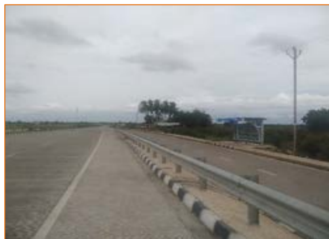
End point of Sangola Bypass at km. 299+150
