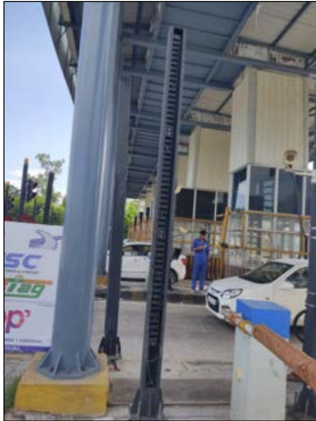
Figure 9-5 Height sensors
