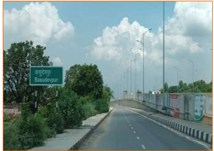
Drain at Service Road at km. 757+200
