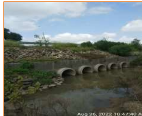
Pipe Culvert at km. 124.106 - RHS (Widening)
