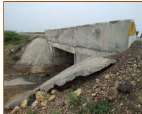
Slab culvert at km. 475+860 (LHS)
