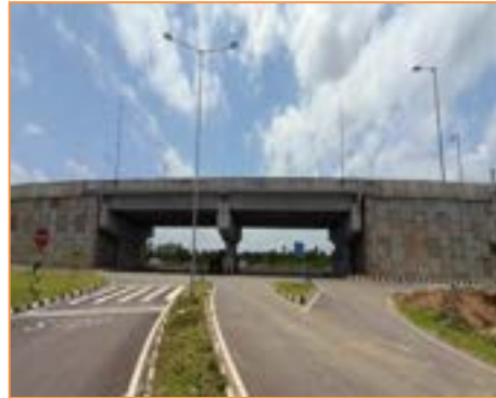
View of UDFO at km. 20+440
