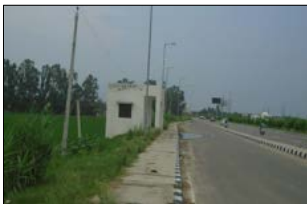
Truck Lay-Bye at km. 1+600
