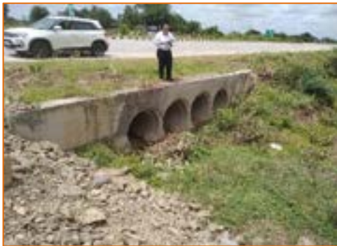
Pipe Culvert at km. 276+190
