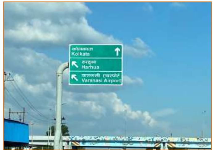
Cantilever Gantry Sign at km. 782+500
