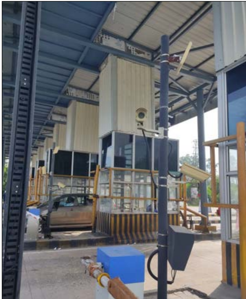
Figure 9-9 LPIC and AVC Cameras
