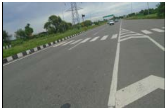
Road Marking at km. 15+800 (RHS)
