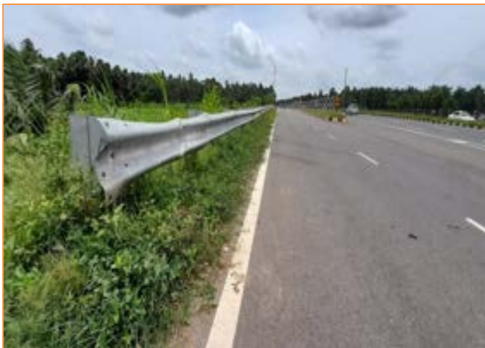
W beam Crash Barrier at km. 52+300
