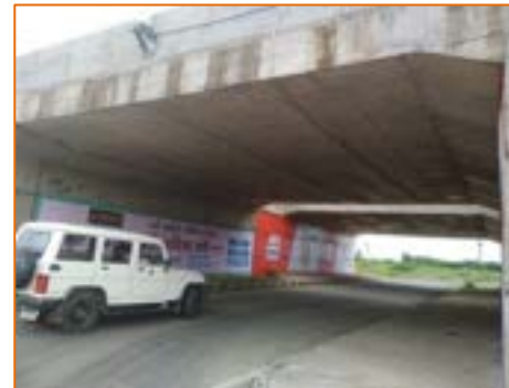
Light Vehicular Underpass at km. 320.900
