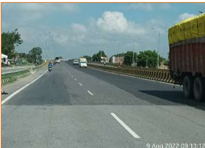
Road Marking to be done at km. 779+850
