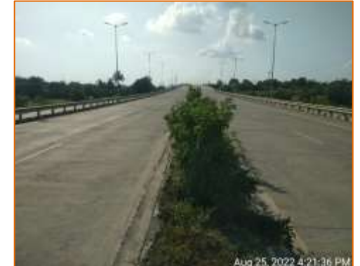
Good PQC surface of MCW at MNB at km. 110.930 (BHS)
