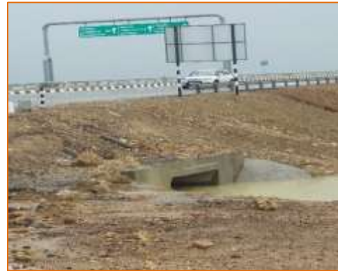
Box culvert at km. 0+060 (RHS)
