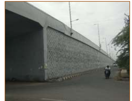
VUP at km. 400+681 (LHS) at A1 side
