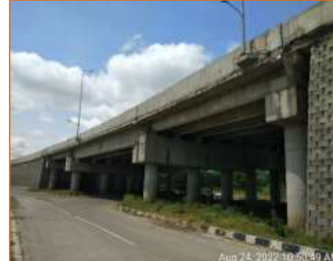
Side View of Flyover at km. 99.900 (RHS)
