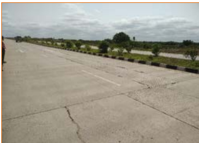
Panel Repair work done at km. 276+050 (LHS)
