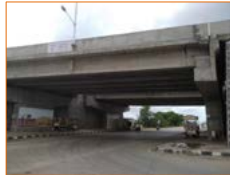
Vehicular Underpass at km. 294.456
