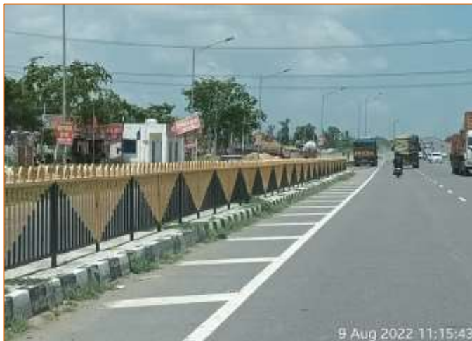
Pedestrian Guard Rail at km. 727+900
