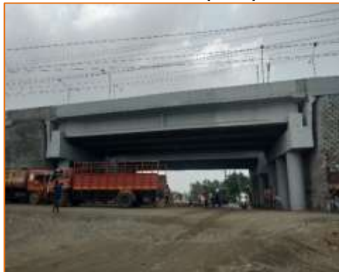
Side View of VUP at km. 55+300 (LHS)
