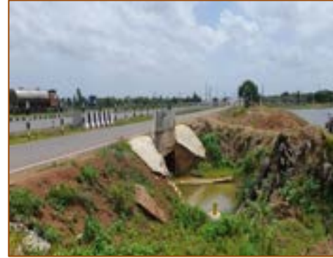
Box Culvert at km. 35+736
