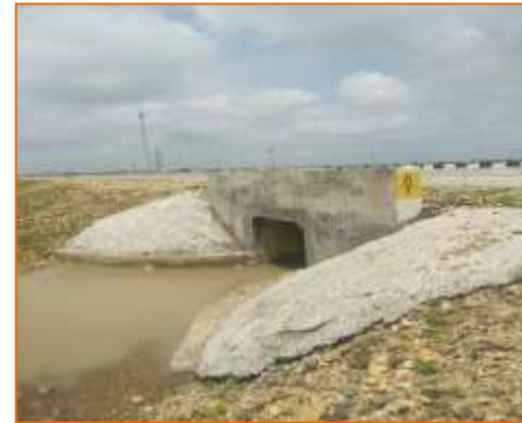
Box culvert at km. 7+240 (LHS)
