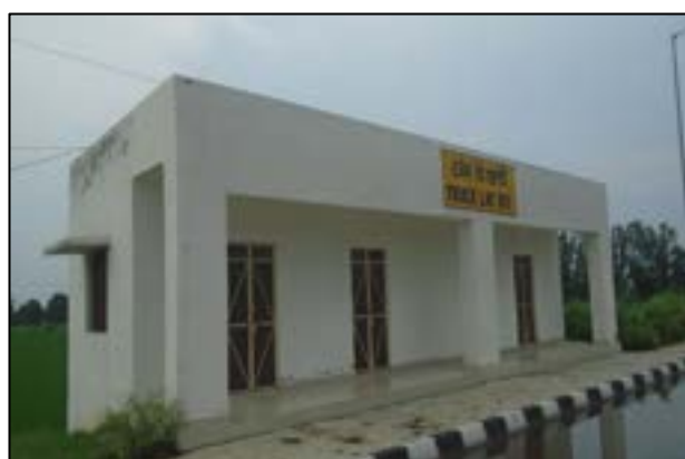
Truck Lay-Bye at km. 1+600
