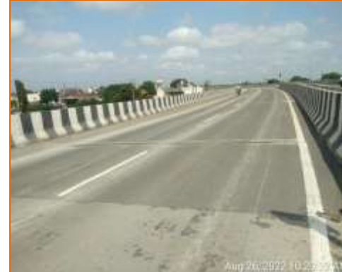
Good condition of BC surface of Flyover at km. 130.650 (LHS)
