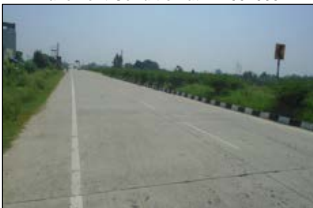
Rigid Pavement at km. 38+000
