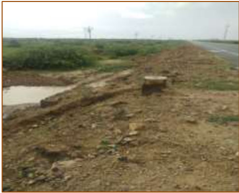
HPC at km. 487+054 (LHS)
