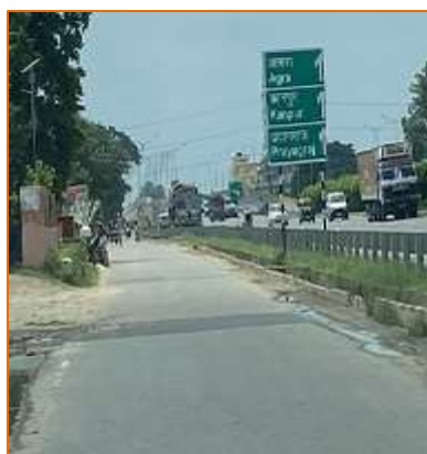
Slip Road at km. 764+700
