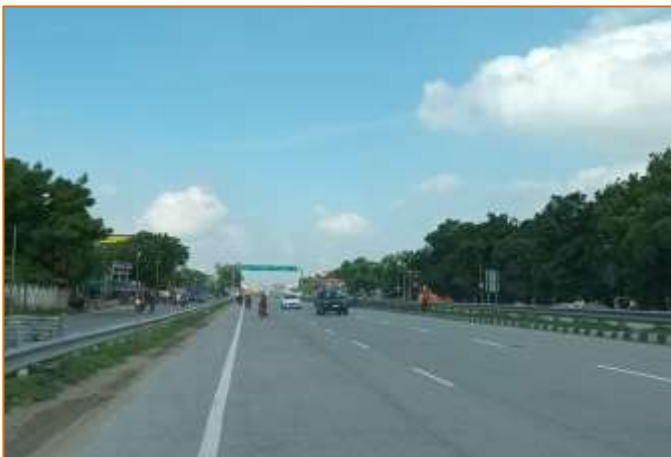
Crash Barrier at km. 785+240
