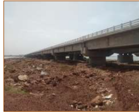
Major Bridge - km. 433+295 (RHS) side view
