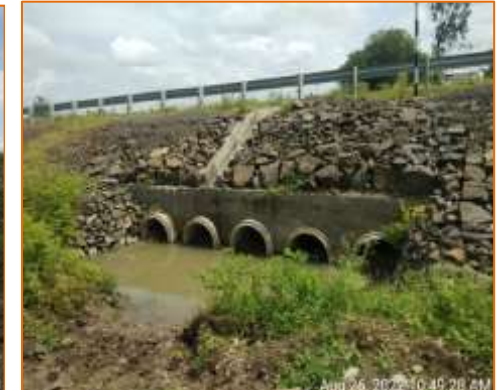
Pipe Culvert at km. 124.106-LHS (Widening)
