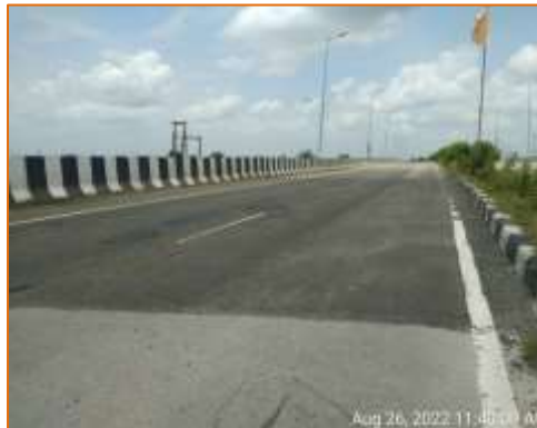
LVUP at km. 111.260 (LHS)
