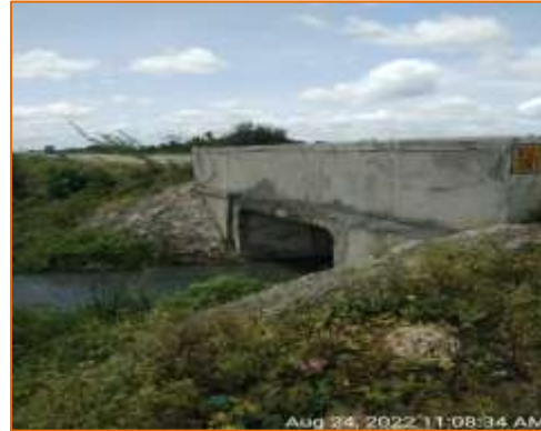
Box culvert at km. 101.823 - RHS (New Construction)
