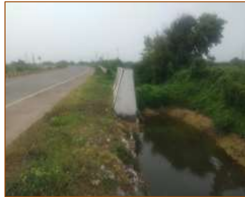
Slab culvert at km. 439+458 (RHS)
