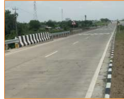
Wearing Coat of Minor Bridge at km. 64+660 (LHS)
