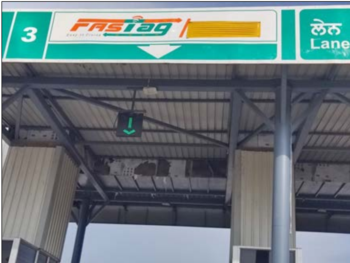
Figure 9-10 Over Head Lane Signal (OHLs)
