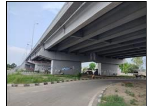
Flyover at km. 9+335
