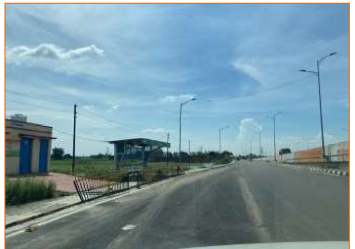
Toilet Block at km. 775+910
