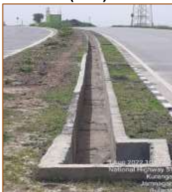
Median longitudinal drain from km. 472+000 to km. 473+000
