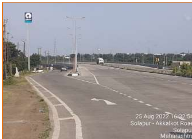
End of the Bypass at km. 106.526
