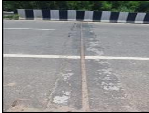
Minor Bridge at km 59+237 (Expansion Joint)
