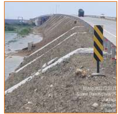
km. 1+000 to km. 0+000 (RHS)
