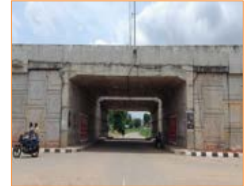
View of LVUP at km 71+140
