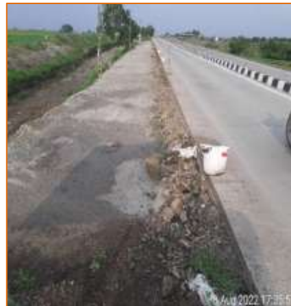
km. 46+000 single lane constructed
