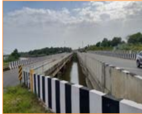
View of Major Bridge at km. 48+222
