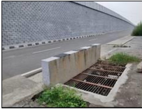
Box Culvert at km. 2+531
