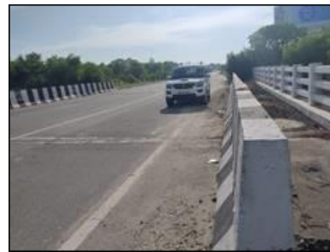
Minor Bridge at km. 71+727 (Top View)
