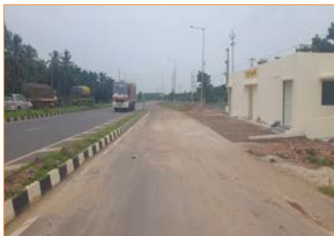
Truck Lay bye at km. 41+500
