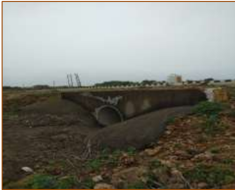
HPC at km. 380+328 (LHS)
