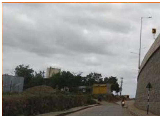
Start point of Sangola Bypass at km. 287+050
