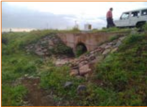
Pipe Culvert at km. 300+020
