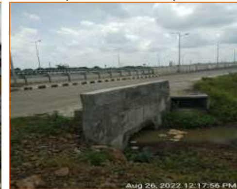
Box culvert at km. 133.524 - LHS (Reconstruction)
