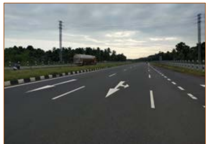
Road Markings at km. 56+760
