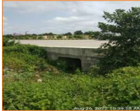
Box culvert at km. 125.495 - LHS (Reconstruction)
