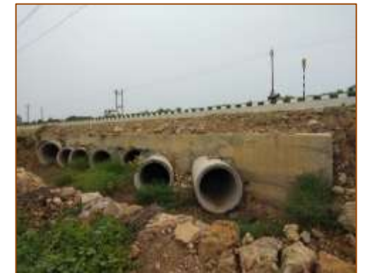
HPC at km. 456+200 (RHS)
