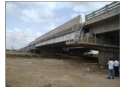
Rail Over Bridge at km. 294.125
