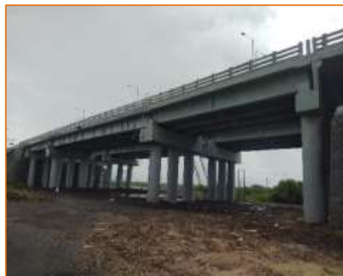
Side View of ROB at km. 0+527 (LHS)
