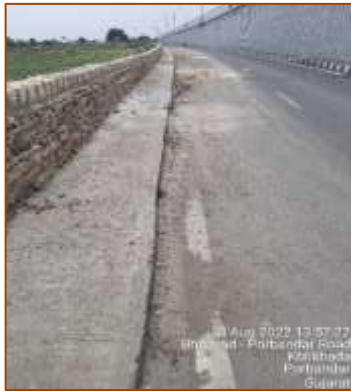
Built-up drain from km. 396+499 to km. 397+466 (LHS)
