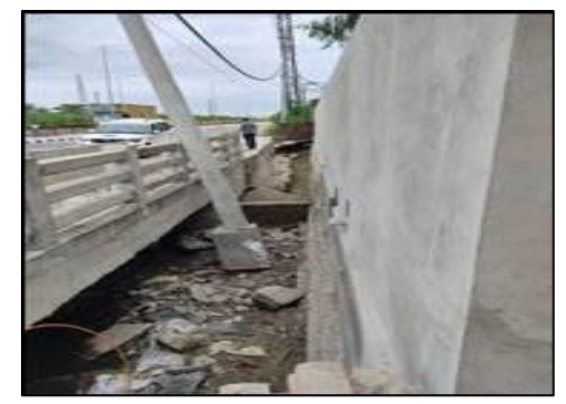
Minor Bridge at km. 80+045 (Structure View)
