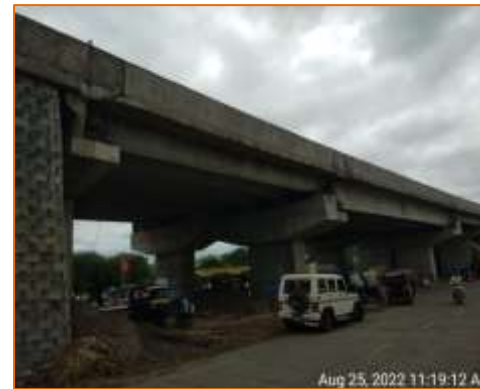
Side View of Flyover at km. 130.650 (LHS)
