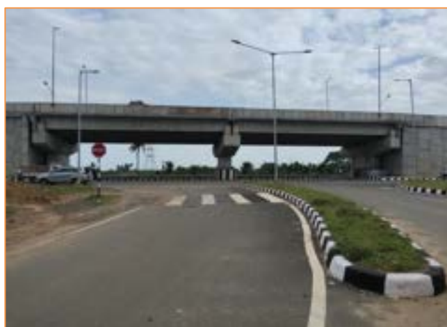
End of Project Road km. 48+830
