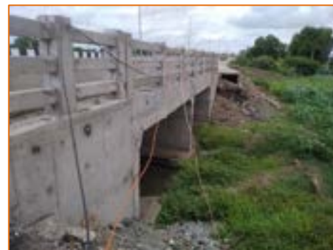
Reconstruction of Minor Bridge at km. 284.835
