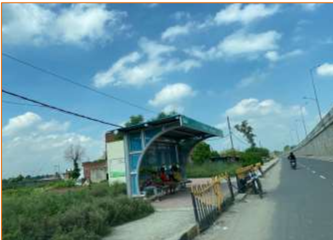
Bus Shelter at km. 775 + 900
