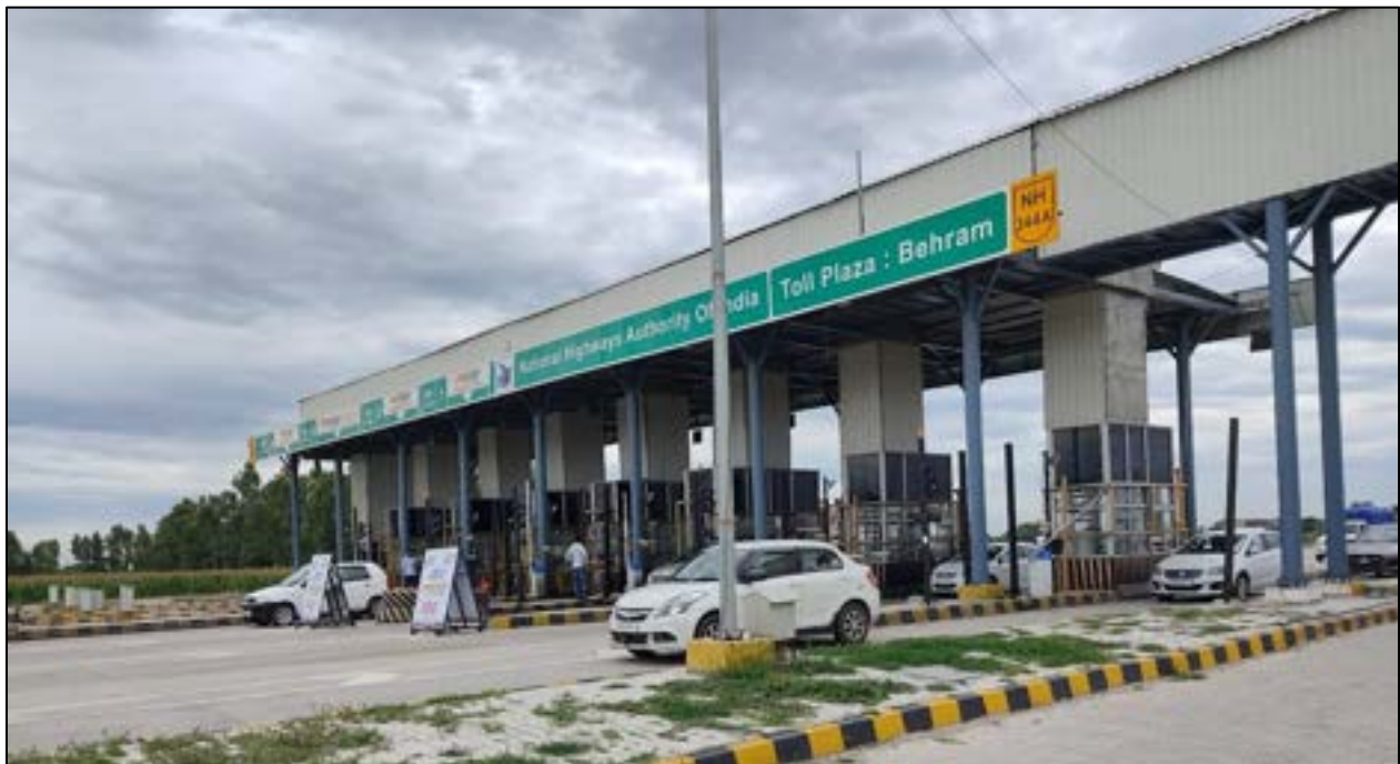
Figure 9-1 View of Behram Toll Plaza (km. 15+300)
