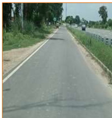
Slip Road at km. 784+400
