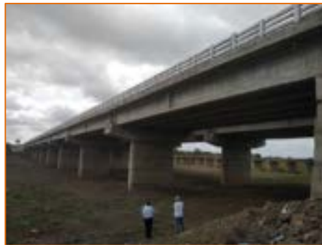
New Major Bridge at km. 298.190
