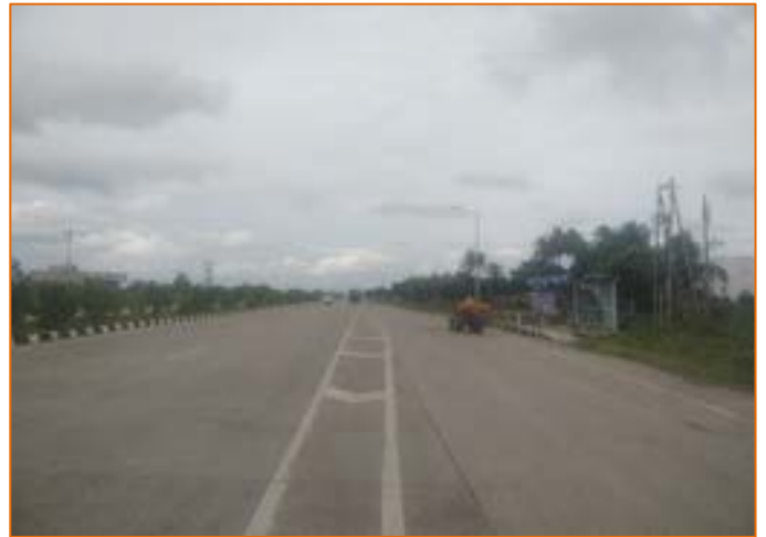
Bus Bay at km. 301+600 (Dighewadi)
