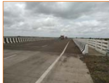
New Major Bridge at km. 280.420
