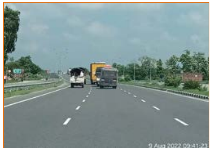
Road Marking at km. 761+200.
