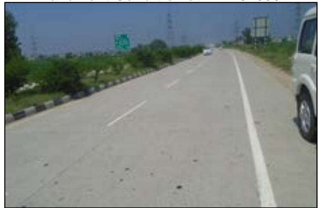
Rigid Pavement at km. 41+000
