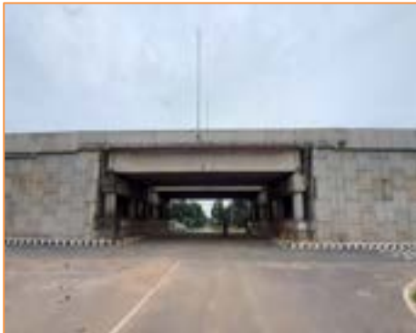
View of VUP at km 63+466
