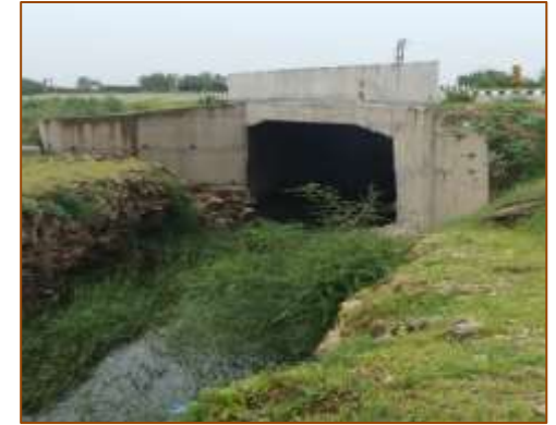
Minor Bridge at km. 385+350 (RHS) - Under COS
