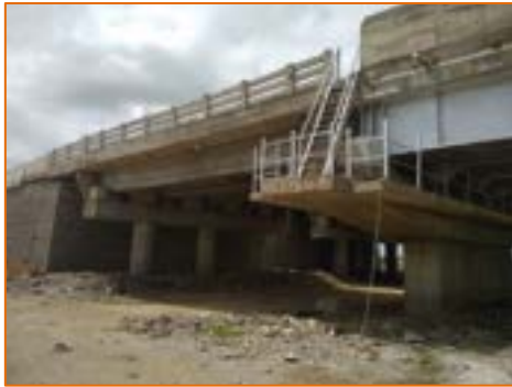
Rail Over Bridge at km. 294.125
