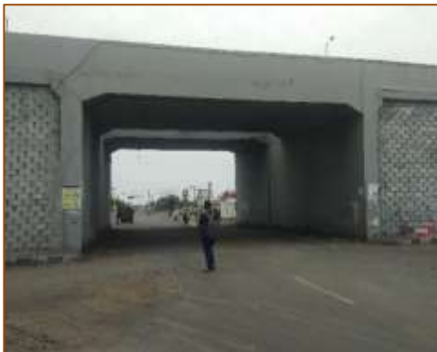
VUP at km. 400+681 (RHS)
