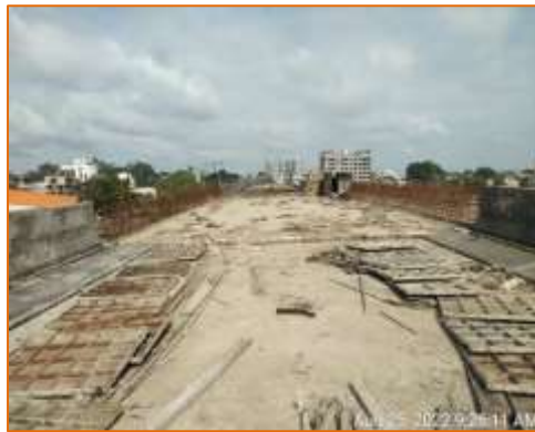
Expansion joint & crash barrier of Flyover is in progress at km. 136.857 (BHS)
