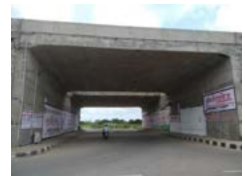
Vehicular Underpass at km. 287.300
