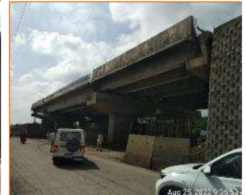
Side View of Flyover at km. 136.857 (RHS)
