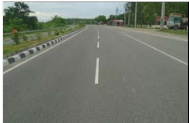
Pavement Condition at km.75+000
