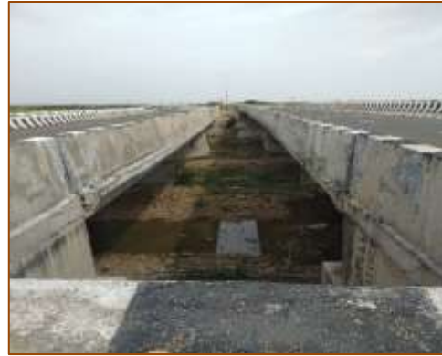
Mid Portion of Major Bridge at km. 395+255
