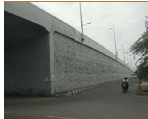
VUP at km. 400+681 (LHS) at A1 side
