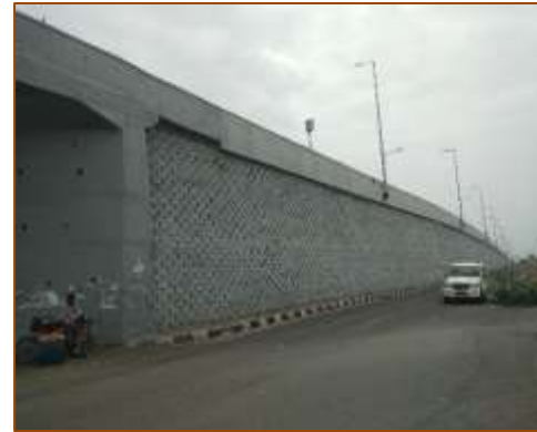
VUP at km. 397+096 (LHS) - Skew - A1 side
