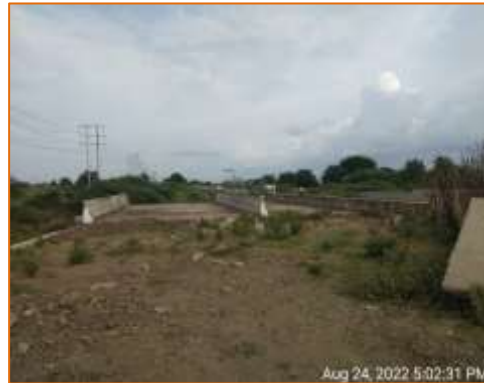
Balance work at A2 side at km. 99.586 - MNB (RHS)
