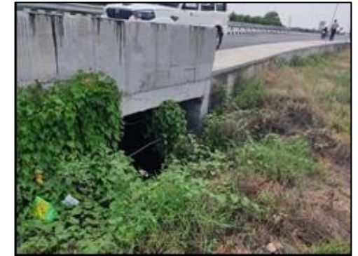
Box Culvert at km. 6+068
