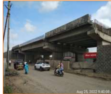
Side View of Flyover at km. 136.857 (LHS)
