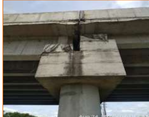
Hessian Cloth @ P2 Pier (RHS) of Flyover at km. 99.900
