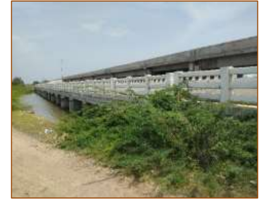
Side View of Major Bridge at km. 420+180 (RHS)
