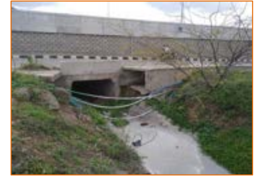
Box Culvert at km. 285+300
