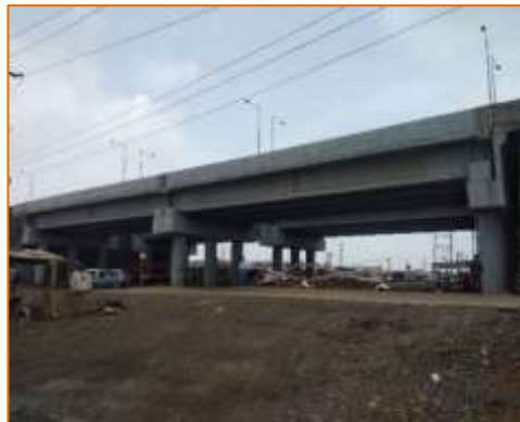
Side View of VUP at km. 12+420 (LHS)
