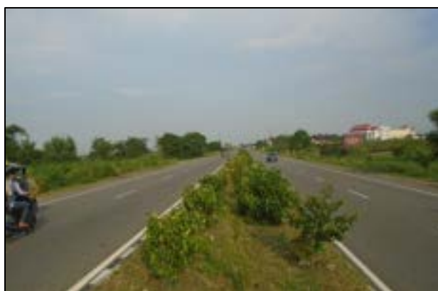
Median Plantation on project highway
