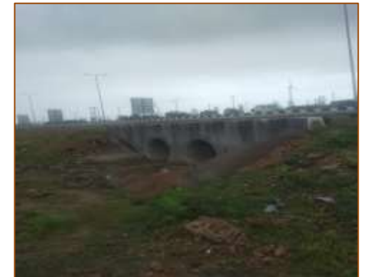
HPC at km. 409+195 (RHS)
