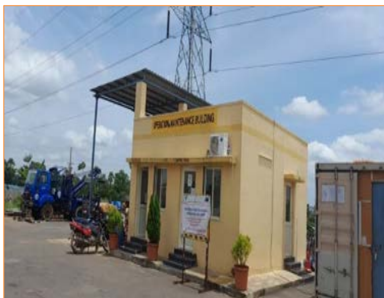
Figure 3-20 Operation and maintenance building at Toll Plaza
