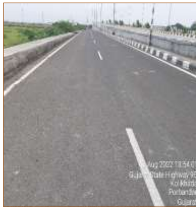
km. 396+499 to km. 397+466 (RHS)
