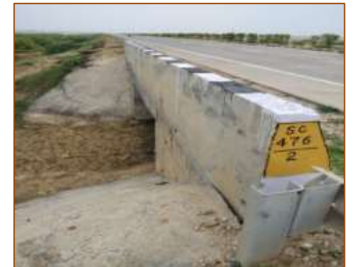
Slab culvert at km. 475+860 (RHS)
