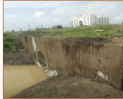
HPC at km. 490+350 (LHS)
