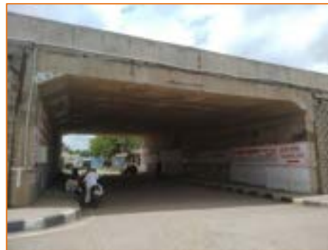
Light Vehicular Underpass at km. 278.700
