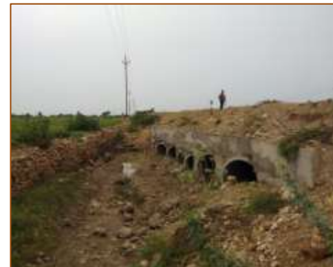
HPC at km. 456+200 (LHS)
