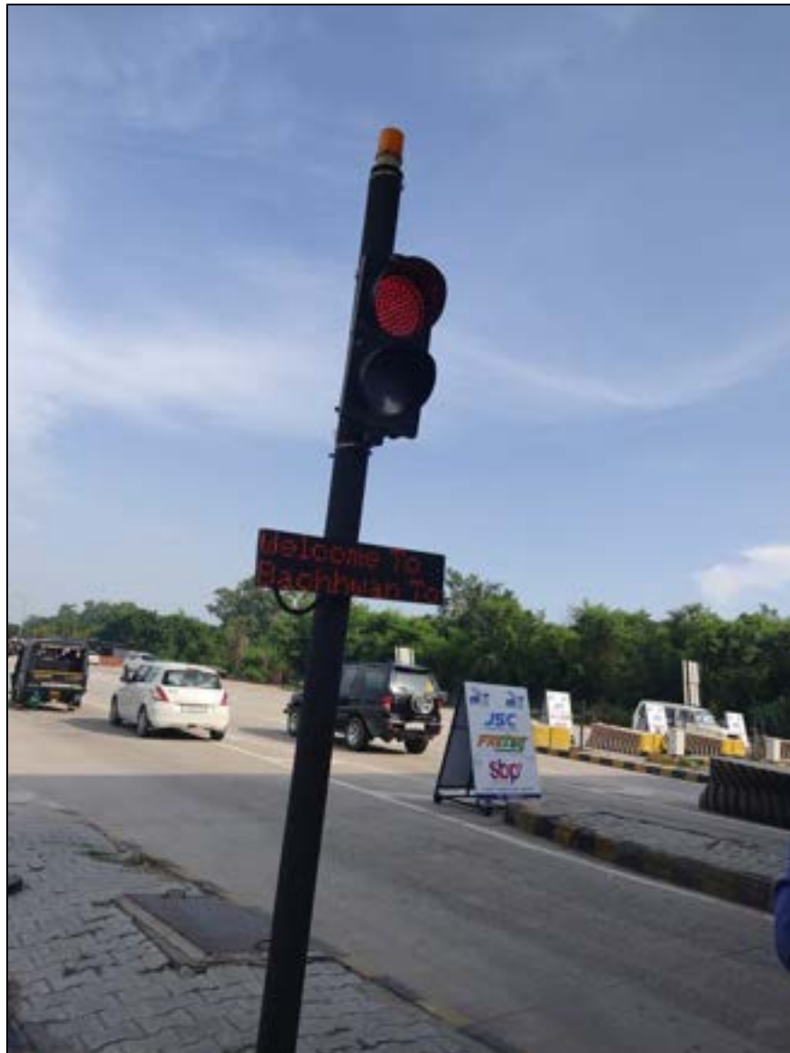
Figure 9-8 Lane Traffic Light (LTL) and User Fare Display (UFD)
