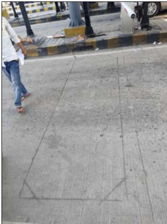
Figure 9-6 Inductive loop
