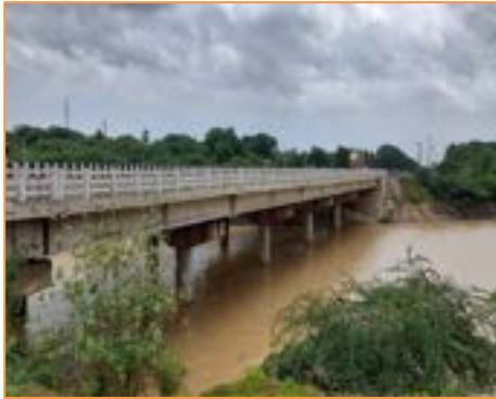
View of Major Bridge at km. 31+647
