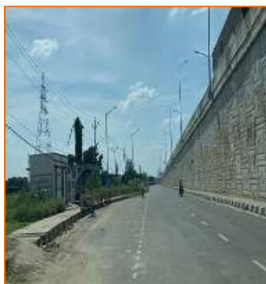
Service Road at km. 781+450
