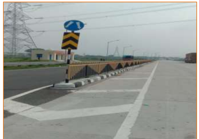
Pedestrian Guard Rail at km.766+600
