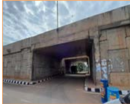
View of LVUP at km 36+420
