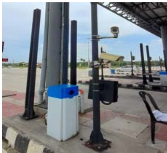
Figure 9-8 LPIC and AVC Cameras
