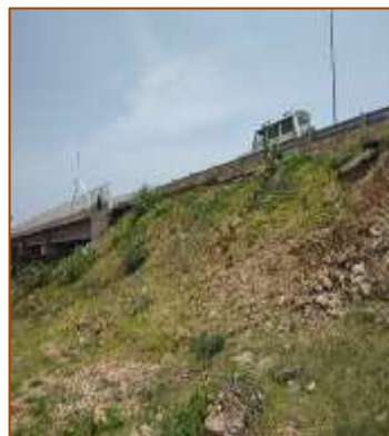
MJB at km. 415+929 (RHS)
