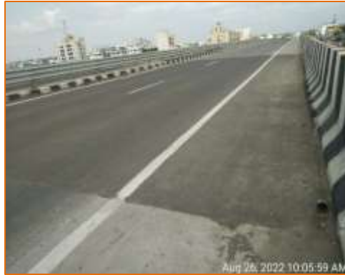
Good BC surface of LVUP at km. 135.100 (RHS)
