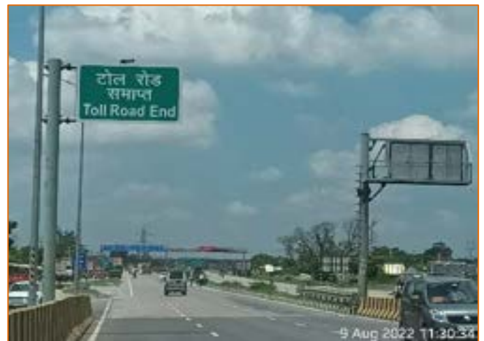
Cantilever Gantry Sign at km. 713+000.
