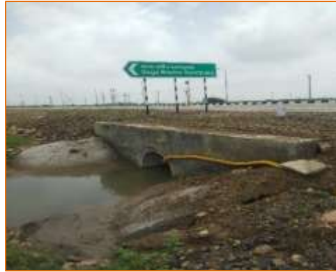
HPC at km. 5+800 (LHS)
