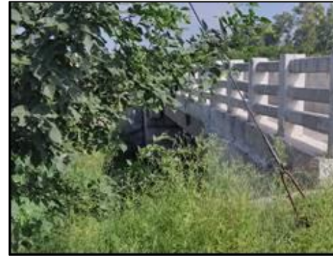
Minor Bridge at km. 63+615 (Existing Structure View)
