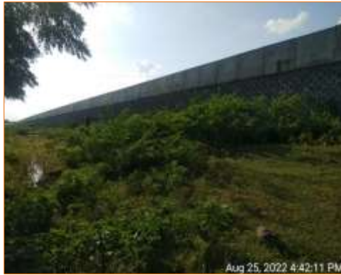
RE Block Wall @ A2 side of PUP at km. 104.820 (LHS)
