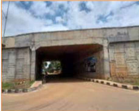
View of LVUP at km 27+790
