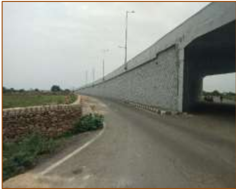
VUP at km. 397+096 (RHS) - Skew - A1 side
