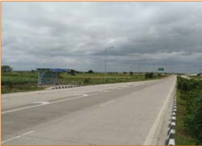
Bus Bay on service road at km. 305+800
