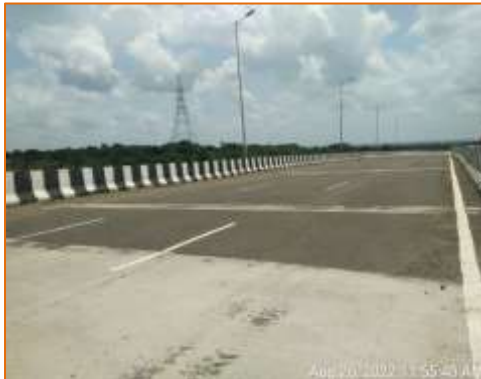
Flyover at km. 106.240 (RHS)
