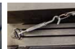
No-drill turn buckle installation
