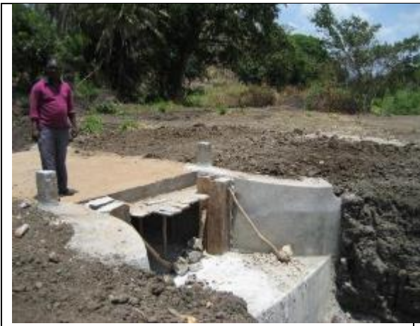
This is one of the two large 80 m long dams made by GSB to create a large artificial lake. This work was funded by the Japanese embassy
