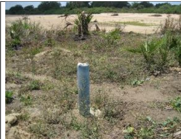
A machine drilled borehole near the Rope pump. The depth is 60 meters but the water at that depth is salt!!! This is part of a 0.5 mln $ project for piped water in Bilibiza.
