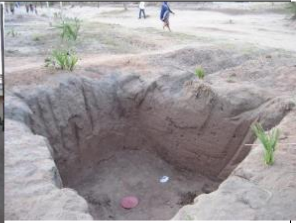
To capture rain water and infiltrate it in the ground, GSB made a large Tube recharge system of 8000 liter near the workshop
