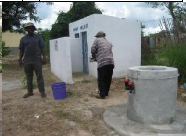
The school wash tank made in February 2016 is working. However the cups that are hanging on the rim were taken away by children
