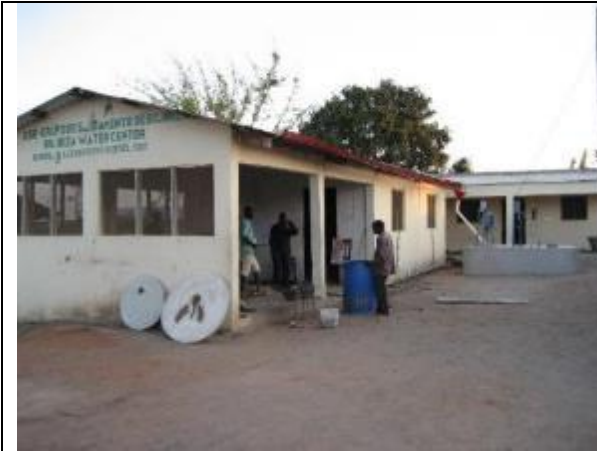
The GSB SMART Centre in Bilibiza. Workshop plus office. Note the new rainwater harvesting tank
