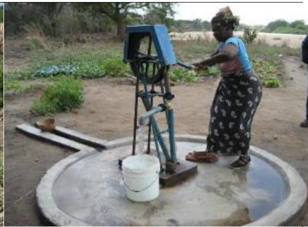
The pump of Mrs. Teresa is OK. The FLOM model works. She sells water at 2 Cents/bucket). This is for pump repairs, some income and she saves money for a new pump.
