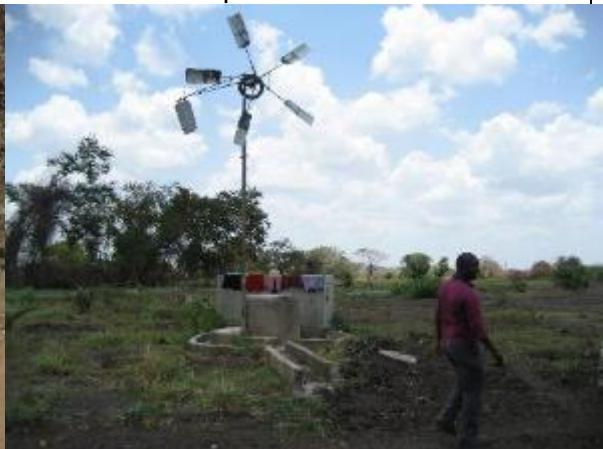
GSB is planning to repair the Wind mill ( wind rope pump) installed in Bilibiza in 2006
