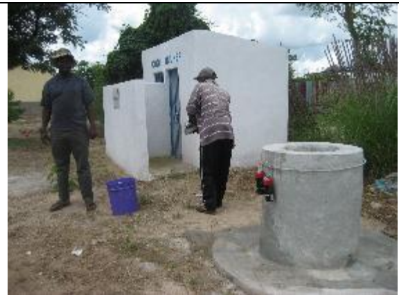
The School wash tank (Bili wash tank) installed in a school in Bilibiza
