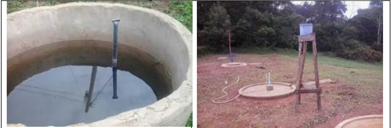
Water storage tank combined with Tube recharge . The tank is full in rainy season
