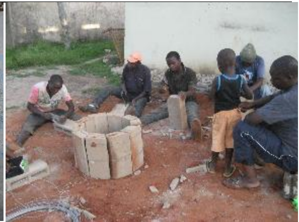
Training in making a School wash tank.
