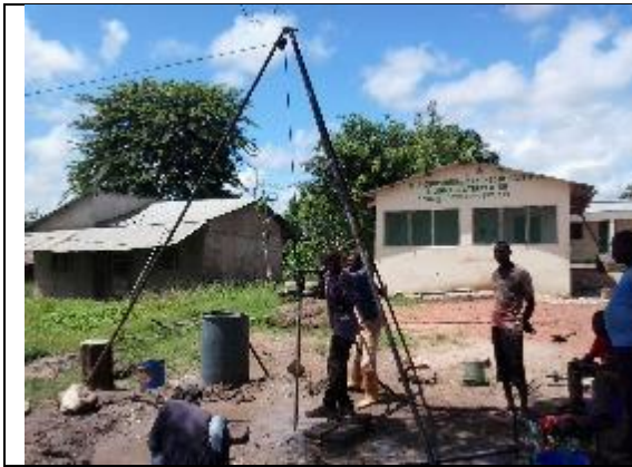
Training in SHIPO drilling with Jetting
