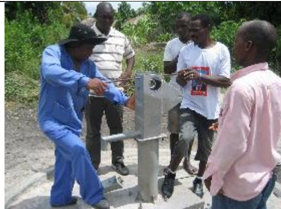
Repairing an Afridev pump. GSB is now involved in repairing 10 Afridev pumps.
