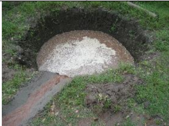
Tube recharge. Here a Tube recharge pit at the GSB Training Centre
