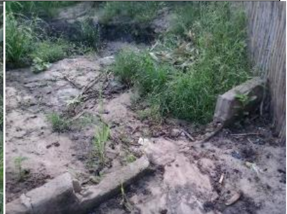
Here a hole for a Tube recharge system that was completely filled up with mud by the flood
