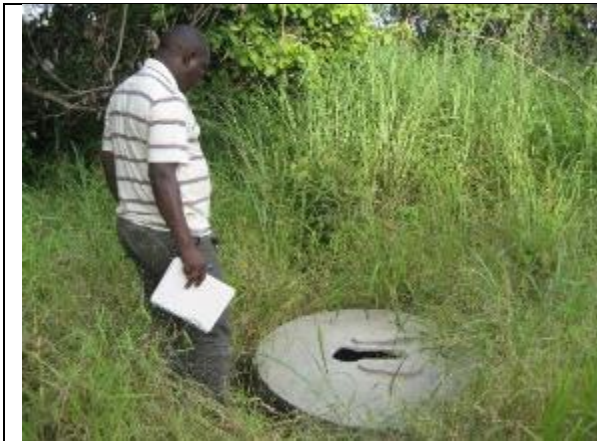
Inspecting a school latrine in Bemvindo installed 6 years ago in a Arrakis funded project. The Super structure has gone but the slab is still used.
