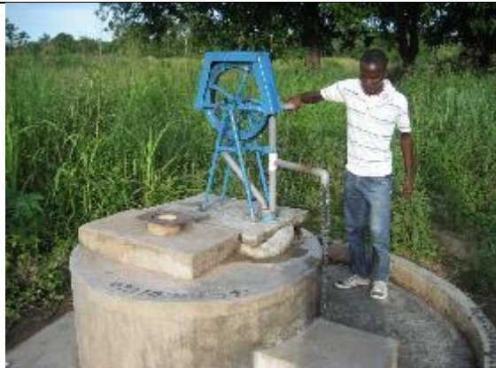
This Rope pump replaced a broken Afridev pump. The cost of repairing the Afridev pump was more than installing a new Rope pump.
