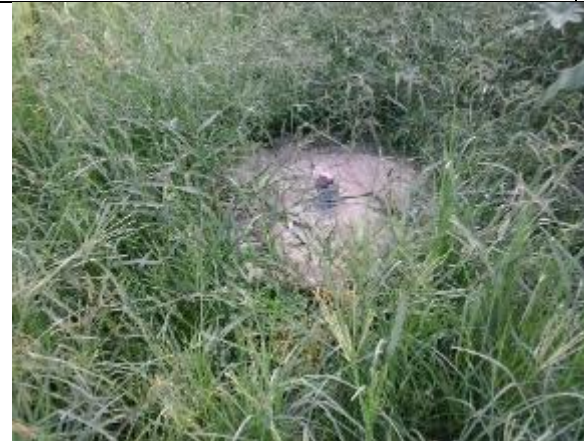
More effects of the flood. The Rope pump installed on this tube well was taken off before the floods and the well closed with a cap. After the rains the pump will be installed again
