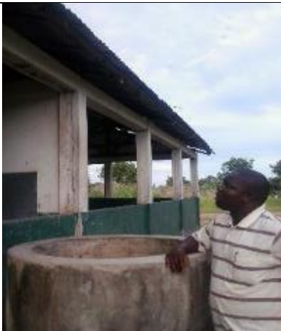
Rain water harvesting tank built in a former project. Despite broken gutters it is still used.
