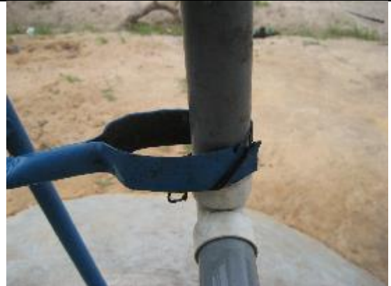
Here the pump pipe support is too short
