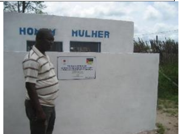
One of the 20 School latrines built with funds from the Japanese embassy
