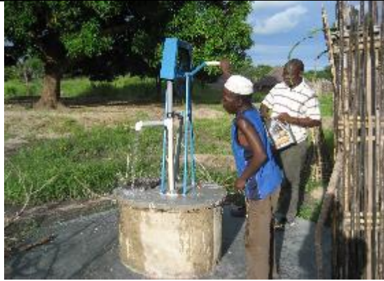
Pump problems. In this case the pump should have a Platform so the handle is at the height of the belly button
