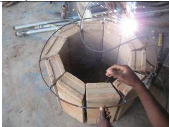
Making a metal ring for the wash tank
