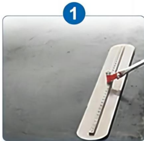
Screeding the concrete
