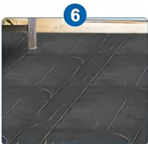
Spray sealing protective agent
