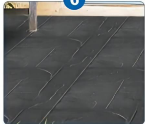
Spray sealing protective agent
