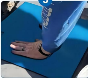
Stamp the concrete
