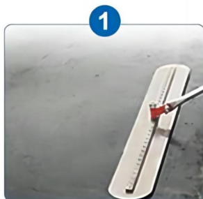
Screeding the concrete
