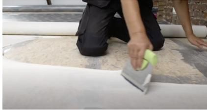
2. Apply the adhesive to the subfloor in accordance with the adhesive manufacturer's instructions.
