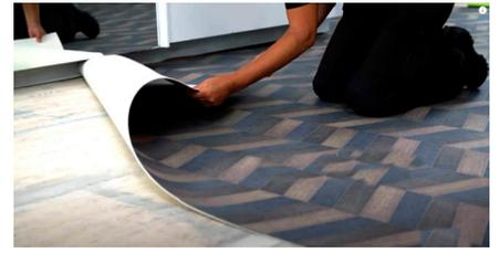
3. Allow the recommended drying time and then reposition the flooring material over the prepared subfloor.
