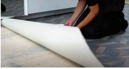
1. Turn back the first piece of flooring to expose about half of the subfloor.
