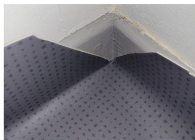
4. Cut section as shown, once completed open up to see perfect corner shape cut - trim edges.
