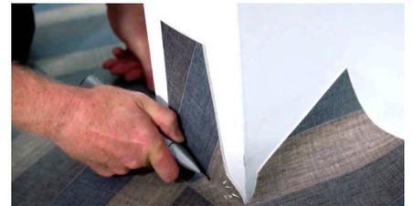
6. With the material now lying flat around the fittings and corners, the final cutting along the wall lengths can be carried out.
