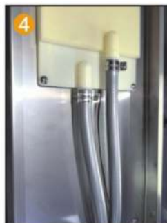
4 Fix the PVC pipe with a throat clamp On the top spray joint
