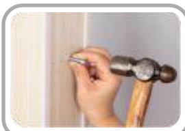
14. Insert the expansion screw in de gaten.
