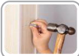
14. Insert the expansion screw in die Löcher.
