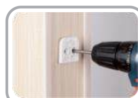
15. Drill the two brackets to wall as the holes.
