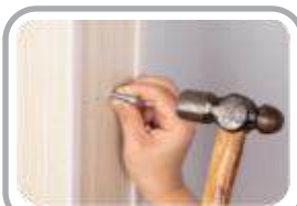
14. Insert the expansion screw in de gaten.
