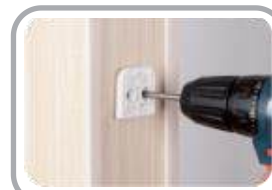
15. Drill the two brackets to wall
