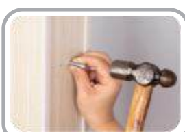
14. Insert the expansion screw do dziur.
