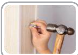
14. Insert the expansion screw in die Löcher.
