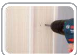
13. Drill holes in the marked place with an electric drill.
