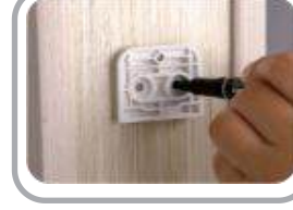
12. Mark the holes position of the two brackets and then pull out the two brackets from wall.
