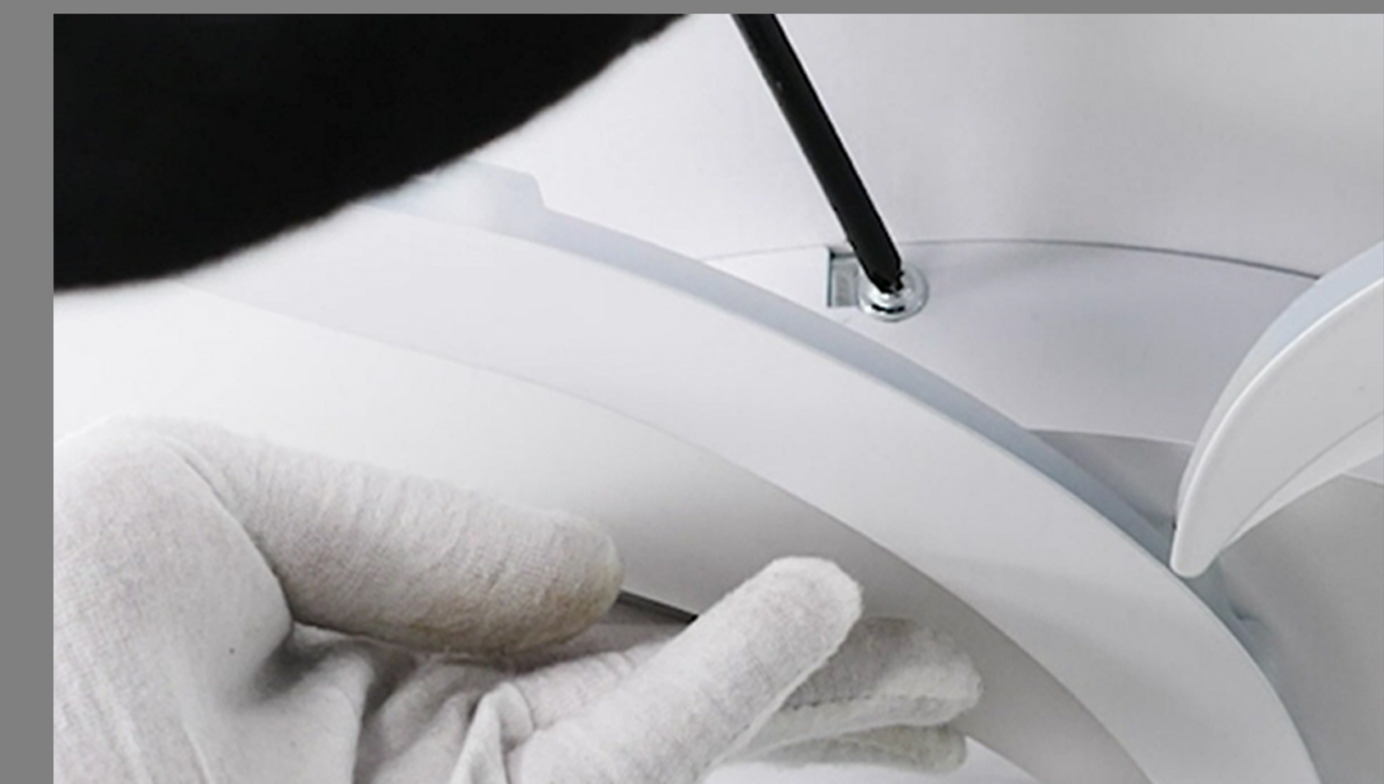
Step 9: Fixing the canopy and mounting plate with screws.
