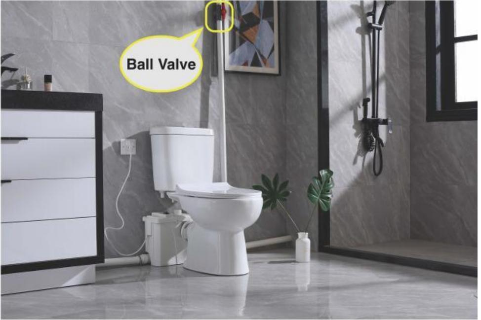
(5-4), Please install a ball valve (not provided) near the water outlet to prevent sewage leakage when the pump is disassembled.
