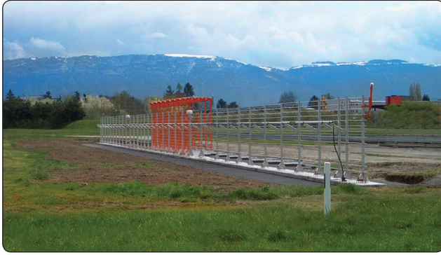
Figure 11-111. An ILS localizer antenna.
