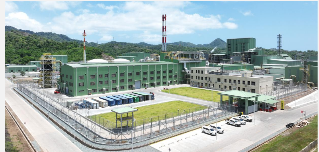
Smelter and PMR complex
