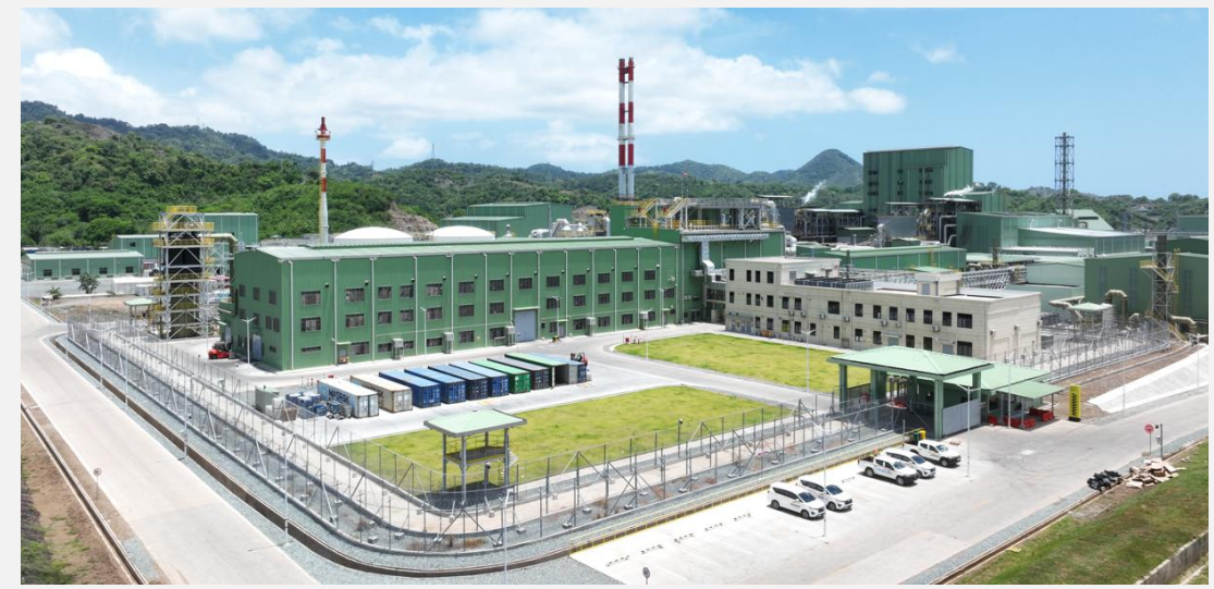
Smelter and PMR complex
