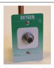
which is serviceable without shutting off the gas service and is capable of supporting 10 pounds @ 2" from the nameplate without leaking.
