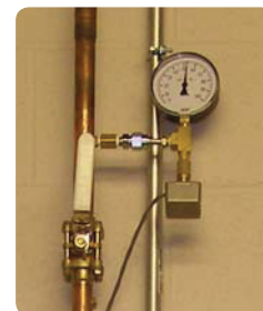
Manifold line transducer mounted remotely.
