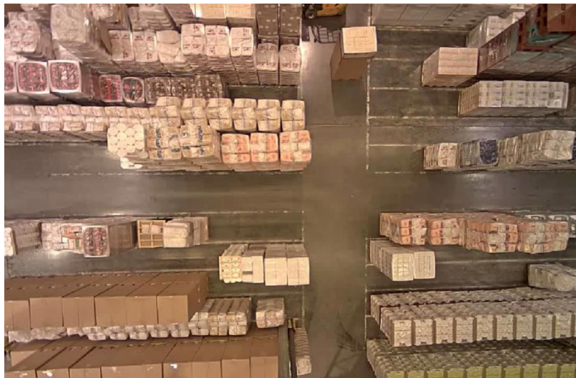
Figure 7: Image of high ceiling warehouse facility where VSD is a suitable early smoke detection method
