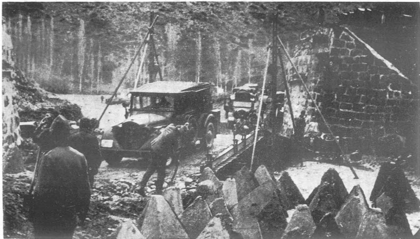
Figure 5. German emergency bridge replaces demolished structure.
