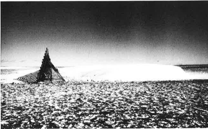
Sixteen-foot-high snow fence, which traps snow more effectively than traditional four-foot-high slat fences.
