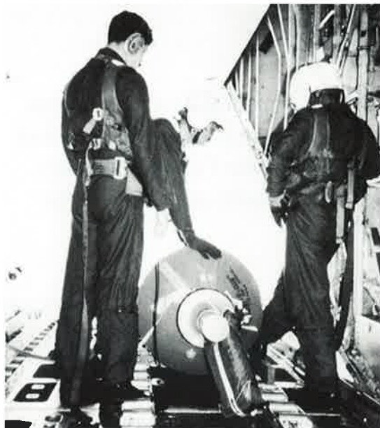
International Ice Patrol air deployment of a TIROS oceanographic drifter over the North Atlantic from a Coast Guard HC-130 fixed-wing aircraft.
