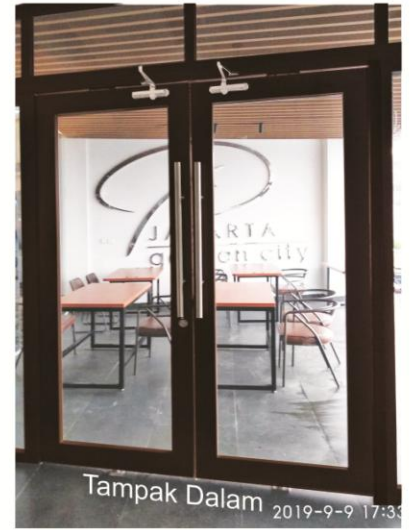
Pintu uPVC Frame Bercat Duco Acrylic Coklat Mahakam + Kaca Bening 5 mm.
