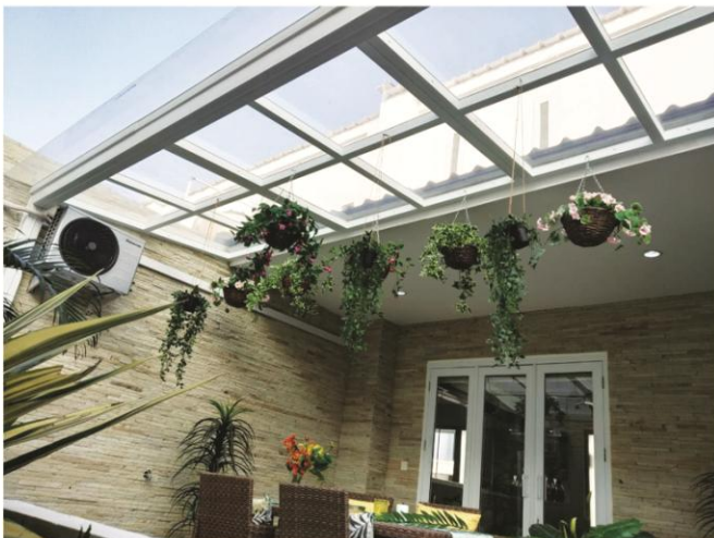
Skylight uPVC Homogeneous White + Polycarbonate.
