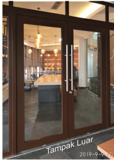
Pintu uPVC Frame Bercat Duco Acrylic Coklat Mahakam + Kaca Bening 5 mm.
