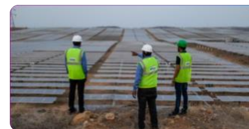
Conventional Module Cleaning System (Manual)
