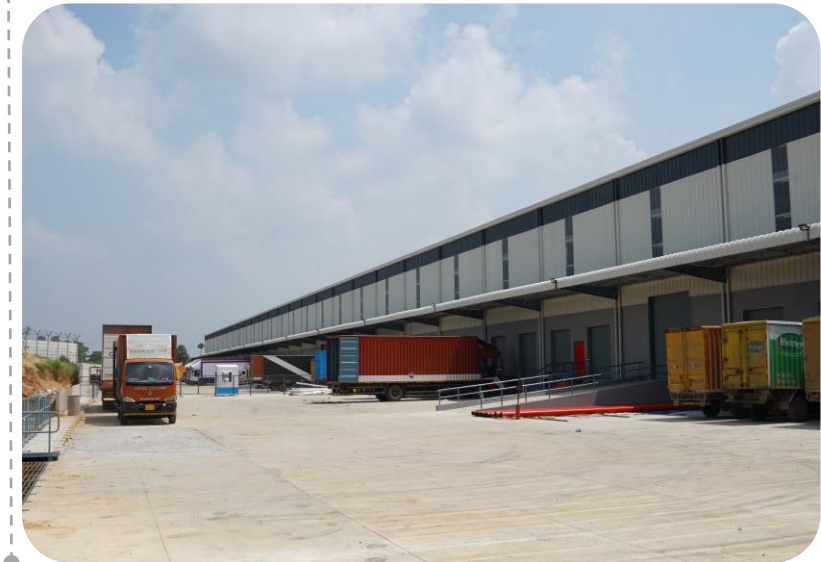
Loading dock at Hyderabad
