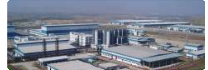
Aerial view of Khandala plant
