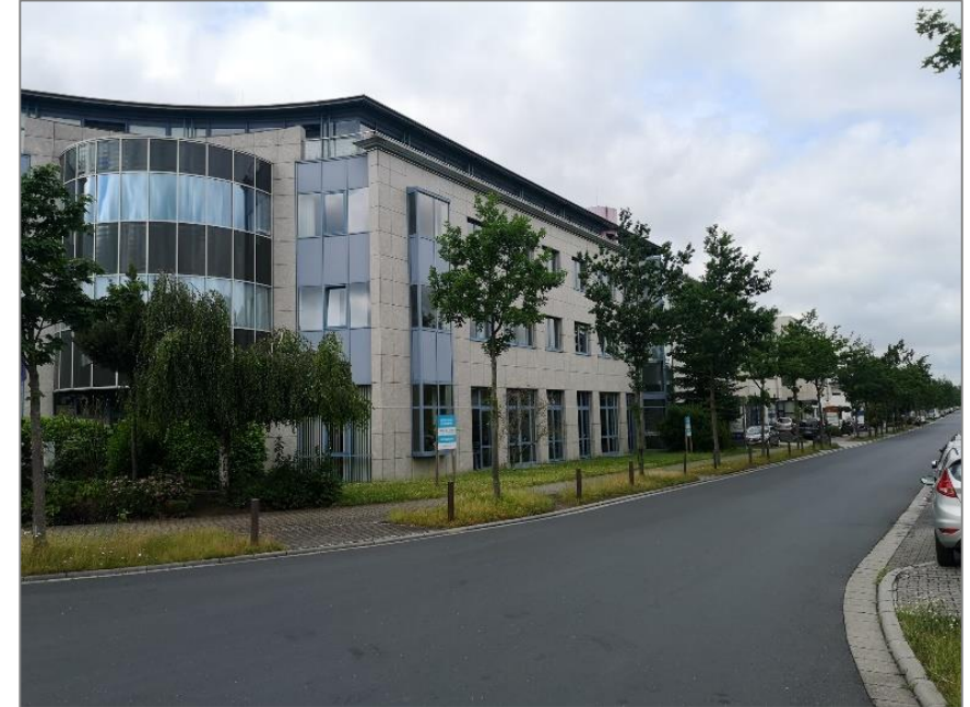
R&D Office, Germany
