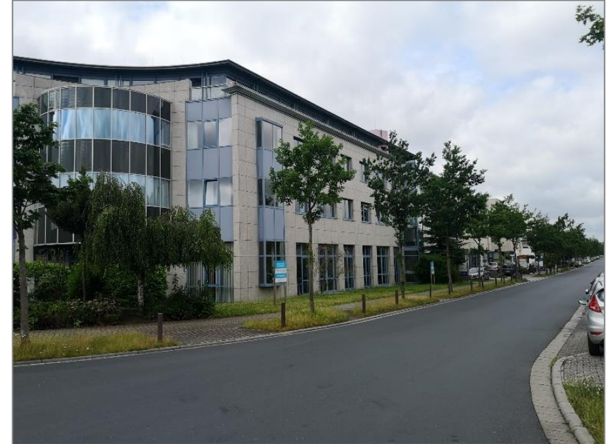
R&D Office, Germany
