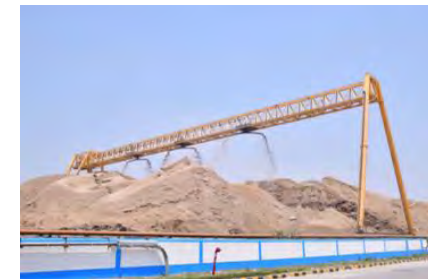
Raw Material Storage and Chipping
