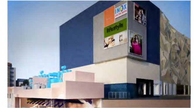
Underground 132 kV SS at 'Quest Mall'
