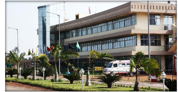
HEL Admin Building - Certified “IGBC Platinum” green building under O&M category in Jan 2018
