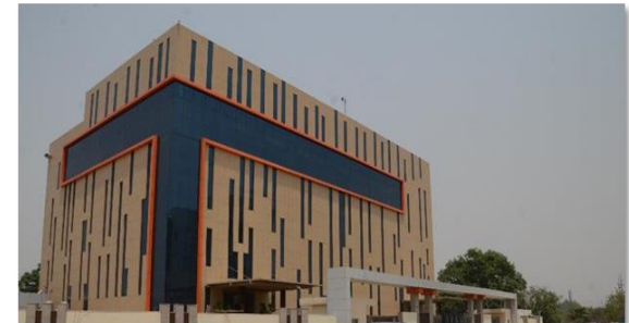
NPCL Corporate Office – Certified as “LEED Gold Green Building” under NC Category in Aug 2018.
