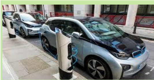
Creation of EV Charging Infrastructure : Public Charging stations**
