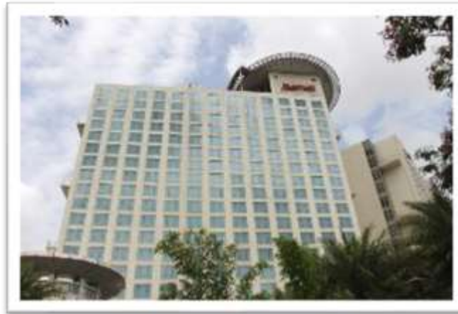
The office space in the erstwhile Accenture Learning Centre Tower to be converted to additional ~140 guest rooms
