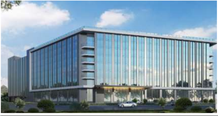
5-star Hotel at Terminal 3, Delhi Airport ~400 rooms
