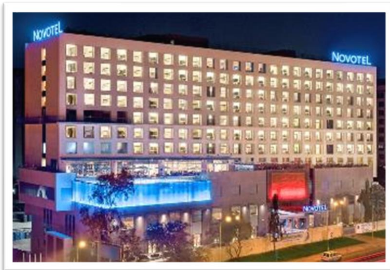
Addition of 88 rooms at Novotel Nagar Road Pune
