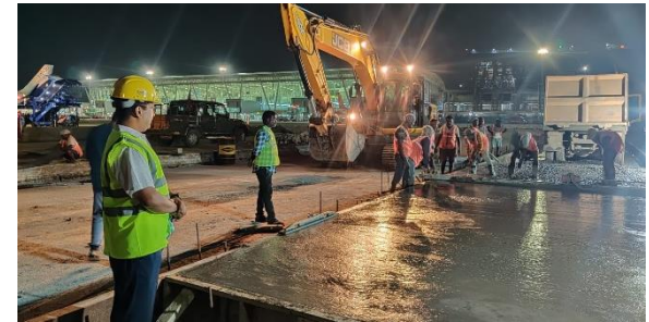
International Airport Taxiway Project, Chennai
