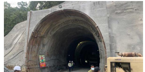
Sevoke-Rangpo Railway Tunnel, Sikkim Blended Cement in Concrete Tunnel Lining
