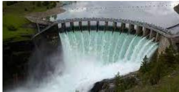
Kopili Hydro Electric Project, Assam
