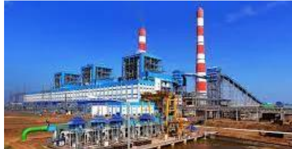
North Karanpura Thermal Plant, Jharkhand 1980 MW (3 x 660 MW) Thermal Plant
