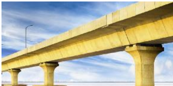
Dhola-Sadiya Bridge, Assam The largest road bridge in Asia
