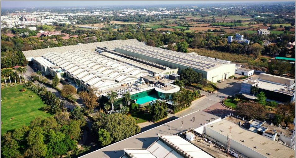
Bird's eye view of the Facility
