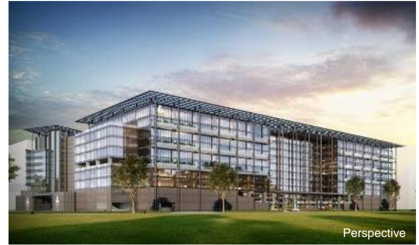
Embassy Manyata – D1/D2 Redevelopment (1.4 msf)
