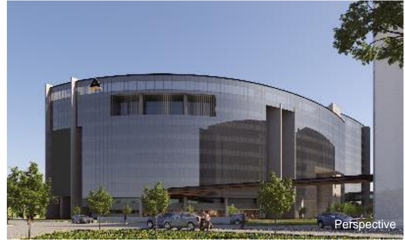
Embassy Manyata – F2 Block (Refurbishment)
