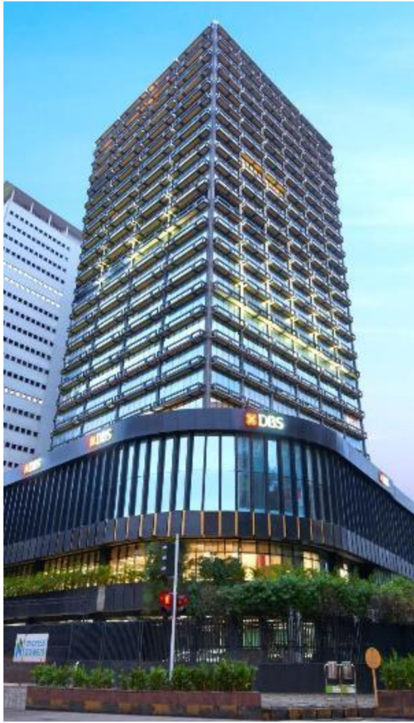
Express Towers Mumbai (0.5 msf)
