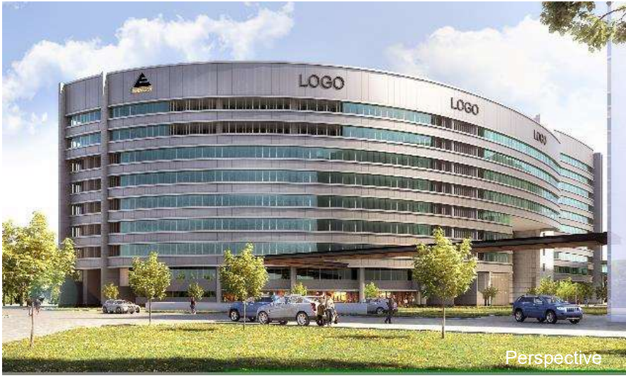
Embassy Manyata – F2 Block (Refurbishment)
