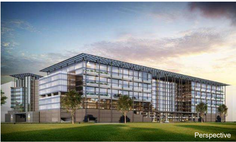
Embassy Manyata – D1/D2 Redevelopment (1.4 msf)
