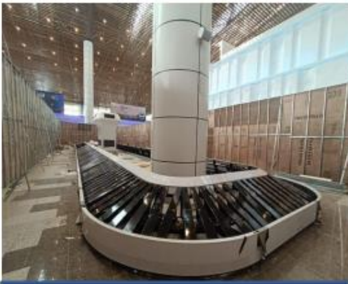
Arrival Hall - BHS works
