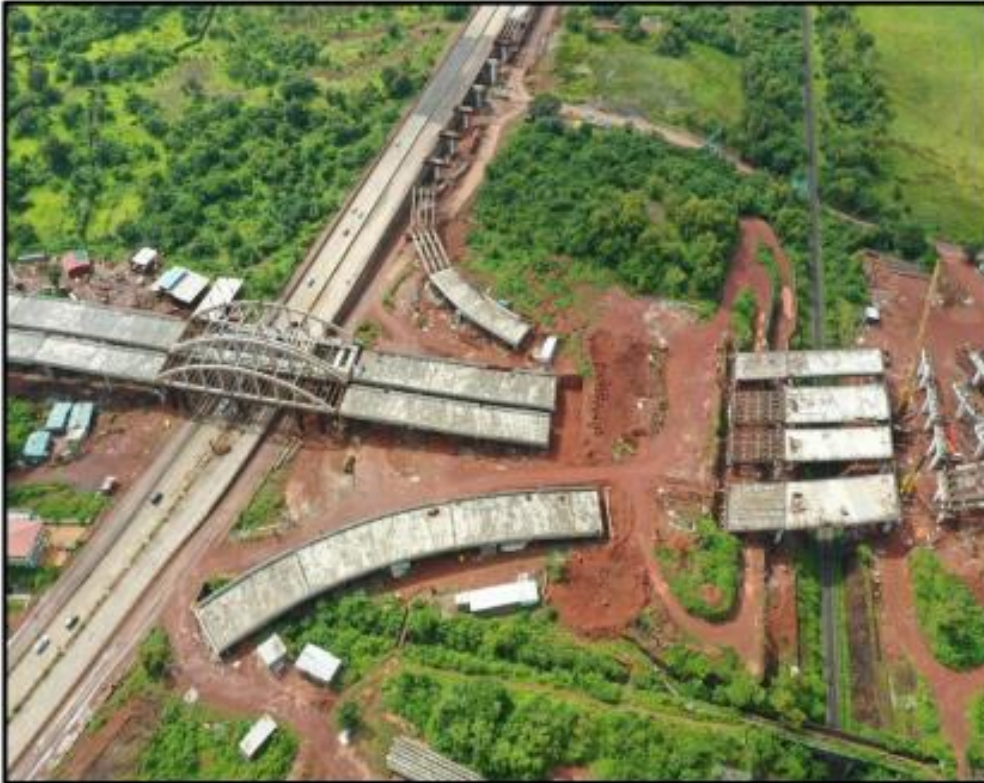
Trumpet Interchange Construction WIP
