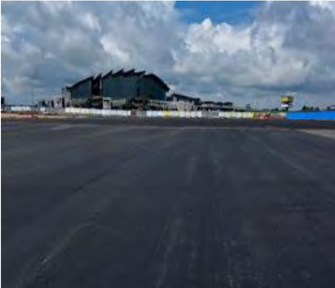
Taxiway at N-E Apron
