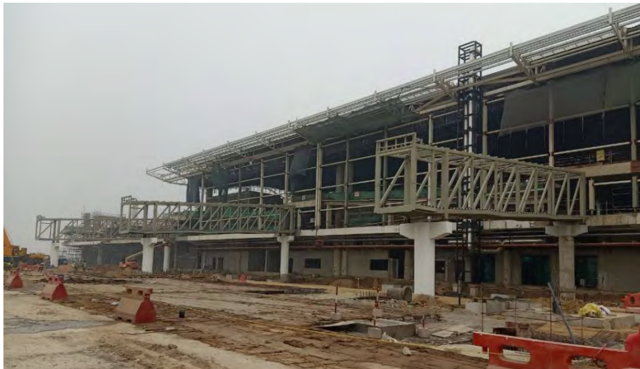
Apron works & Fixed Link Bridges Installation
