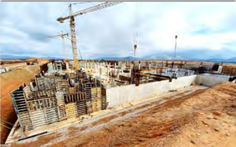
Construction progress - Formwork, Rebar fixing concreting at Terminal Building, Earthwork and road works
