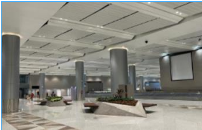
West Processor – Level D
