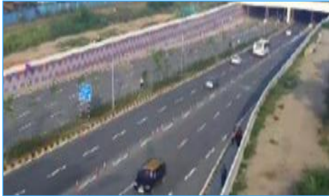
Radisson Under Pass Road
