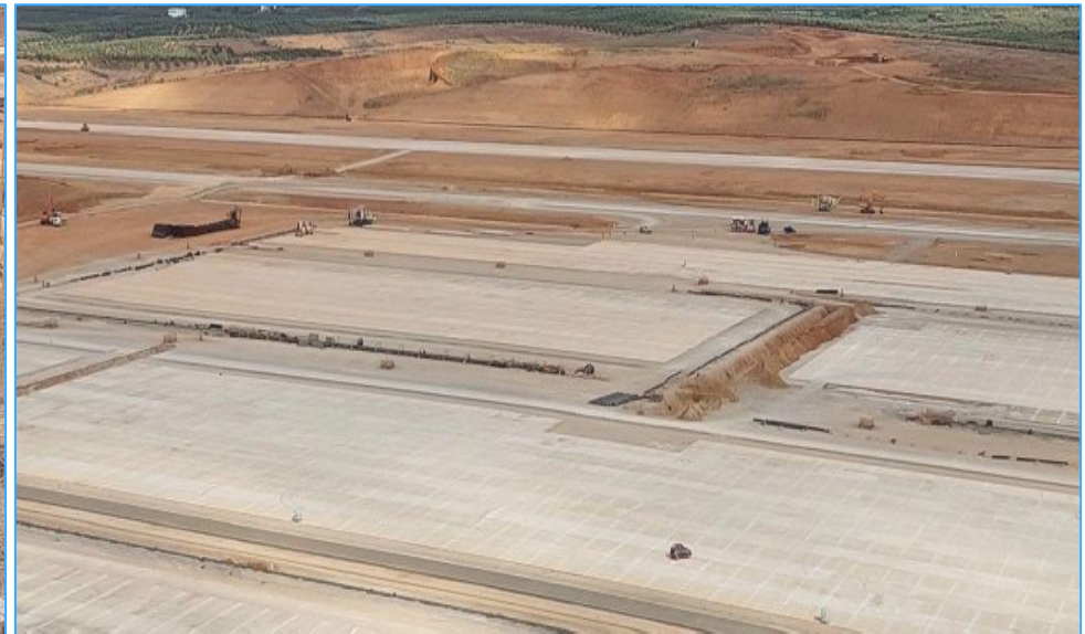
Apron: Laying & Compaction of capping layer & lean concrete pavement work
