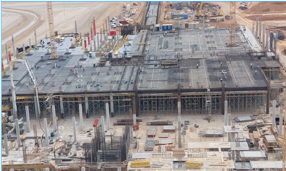
Progress of readiness for departure slab Concreting
