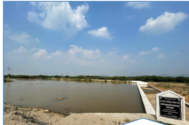
Assessment of water conservation structures through volumetric analysis of 33 check dams.
